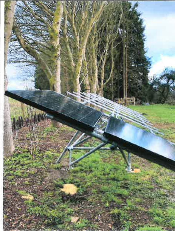
Fig.1 Two PV panels in parallel at 25 degrees on partially completed frame
