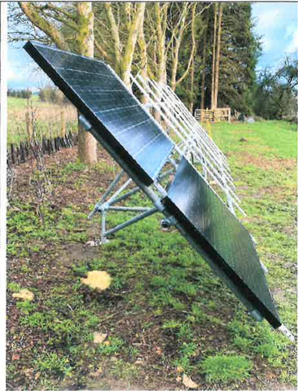
Fig.2 Two PV panels in parallel at 50 degrees on partially completed frame
