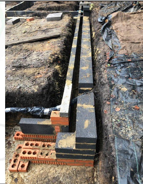
Concrete lintel placed over root with necessary clearance.
