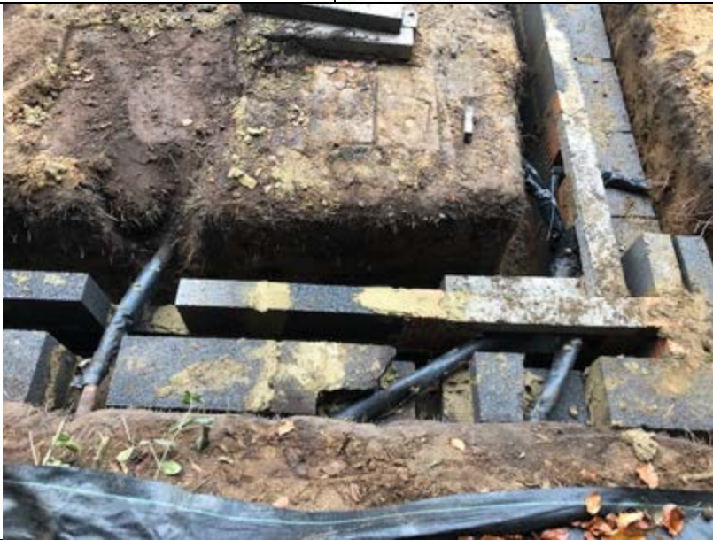
Block work built up around roots giving sufficient clearance.
