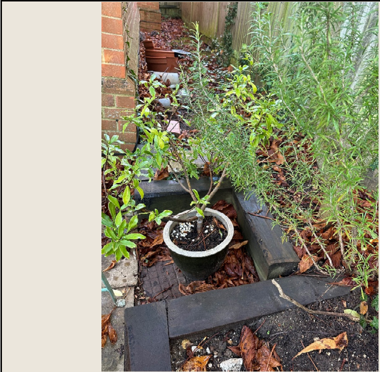
Drainage cover located close to existing property and surrounded by raised vegetation bed.
