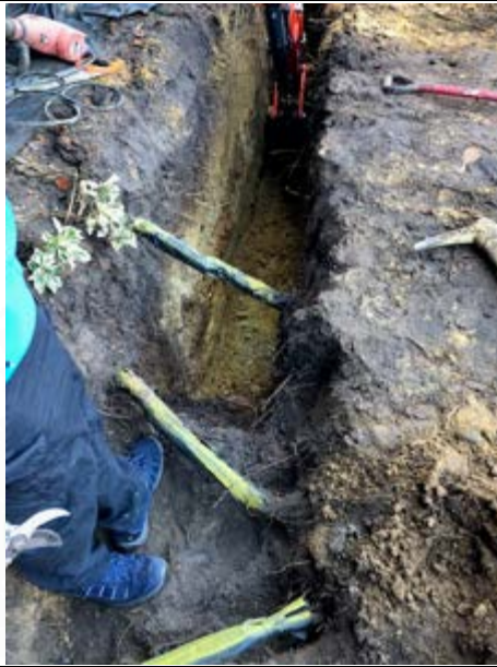
Roots wrapped in hessian and non permeable membrane.
