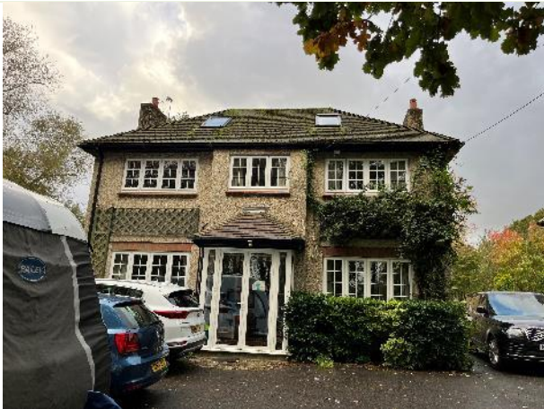
Assessed Structure – front of the surveyed house (northern orientation)
