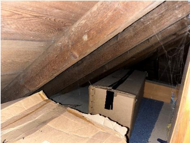
Internal Feature: the accessible side loft
