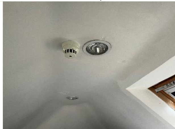
Internal Feature: the inaccessible loft void under the ridge
