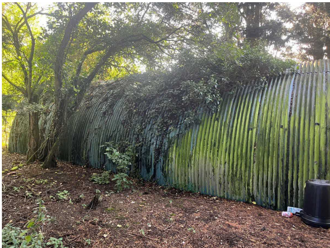
Side Elevation, showing the existing corrugated metal (Iron) sheeting.
