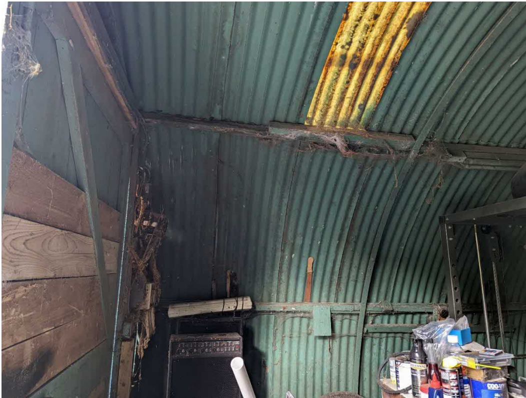
Internal view of Nissen Hut, showing the curved structural T-Shaped ribs, purlins and corrugated iron sheeting exterior.
