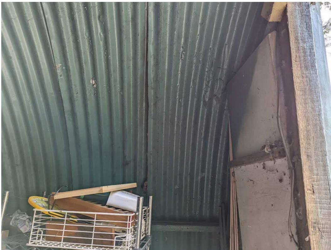
Internal view of Nissen Hut, showing the curved structural T-Shaped ribs, purlins and corrugated iron sheeting exterior.
