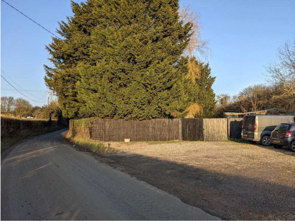
Close boarded fencing and gated entrance to new house site
