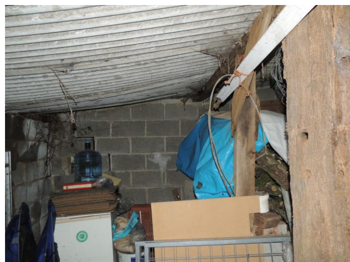
Photo 9: Interior of the building
