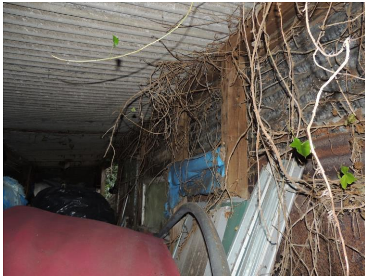
Photo 5: Interior of the building
