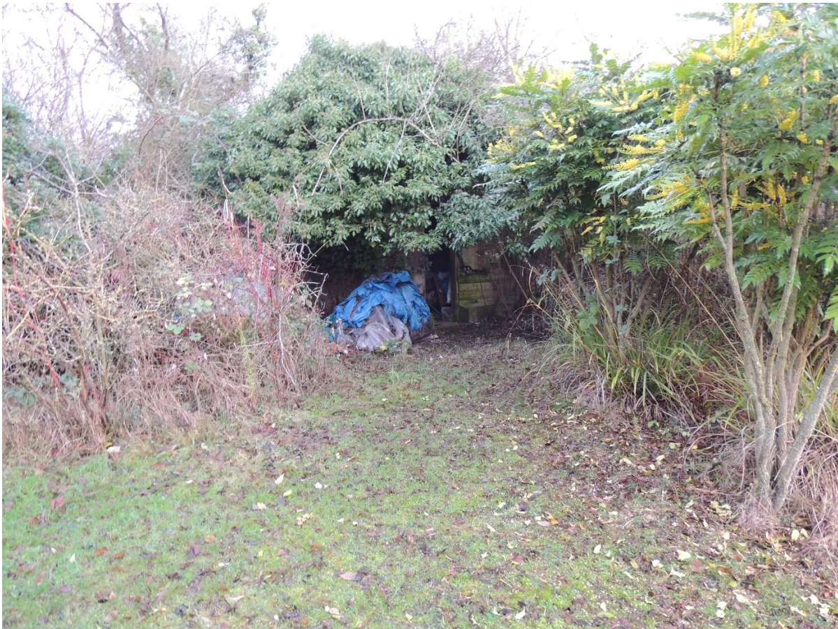
Photo 1: South-western corner of the building which is almost entirely engulfed by ivy. Access to the inside is via the gap in the centre of the picture
