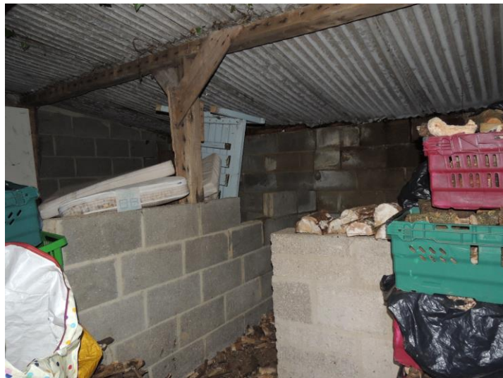
Photo 11: Interior of the building at north-eastern end
