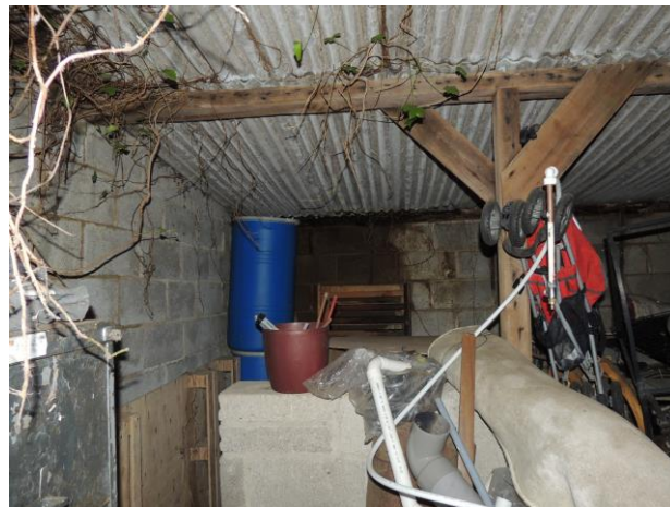
Photo 2: Looking north-westwards in the building
