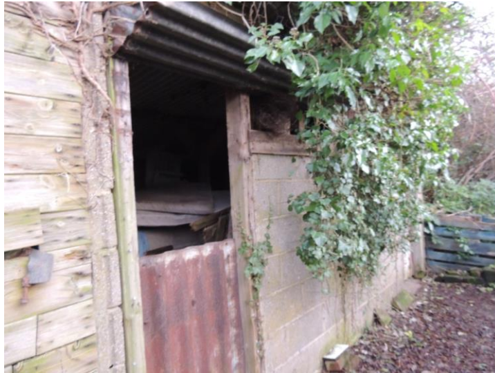
Photo 10: South-eastern elevation at north-eastern end
