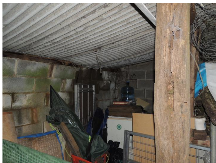
Photo 8: Interior of the building
