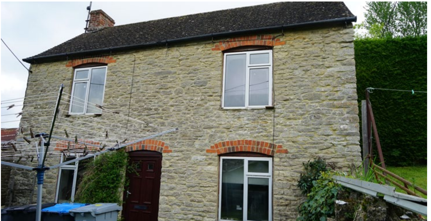
View from the west of the later 19th century wing with shallower pitched roof and brick detailing to the window heads, similar to the cottages opposite rebuilt c1895-8
