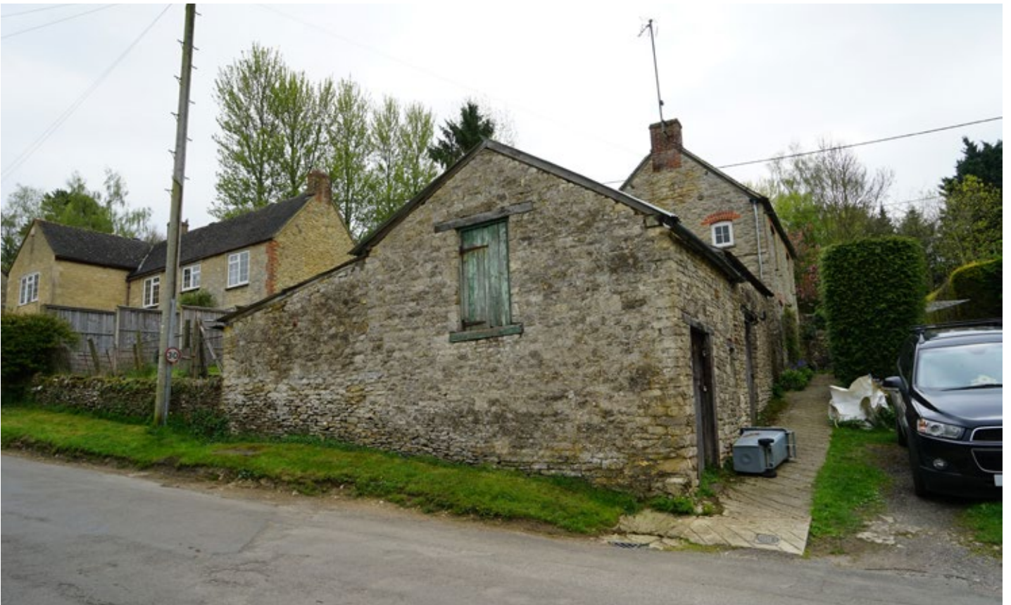
Detail of the gable to the road. The lower courses of stone suggest an existing boundary wall to the road above which the second stable has been constructed
