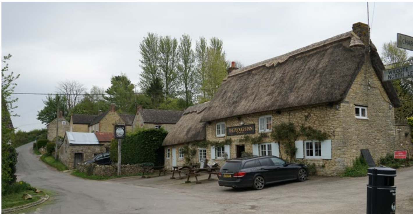
View of 1 Wilcote Riding from the west with The Plough in the foreground, with the gabled roof of the two-storey house beyond, and the two former stables, one with a rusty metal roof, the second with a silver metal roof, stepping down to the road
