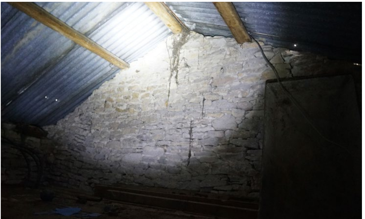
The roof structure is modern and basic
