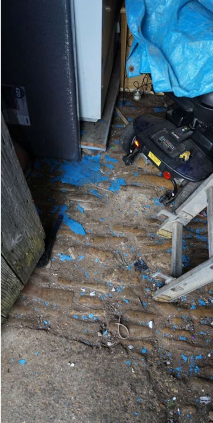
The stone on edge flooring confirms a stable use
