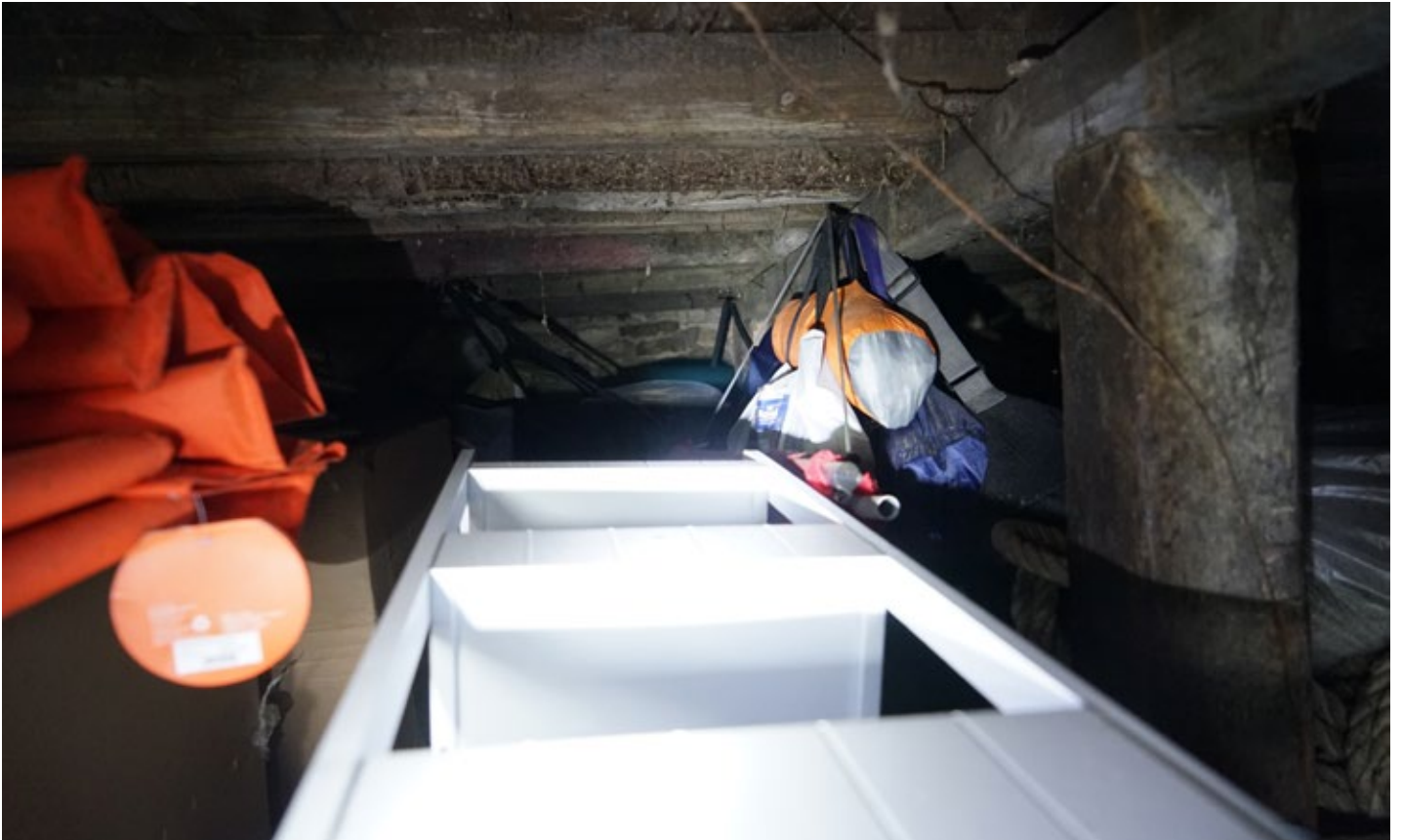
View looking east of the first floor structure
