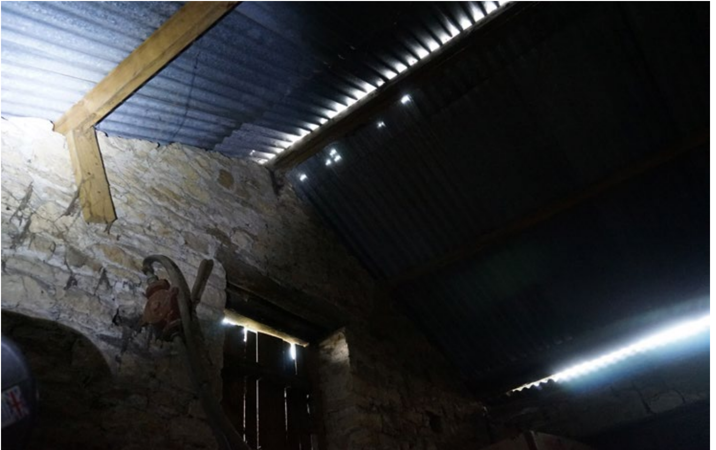
Roadside gable showing the access door
