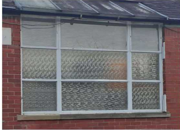
PHOTO OF EXISTING FRAME
