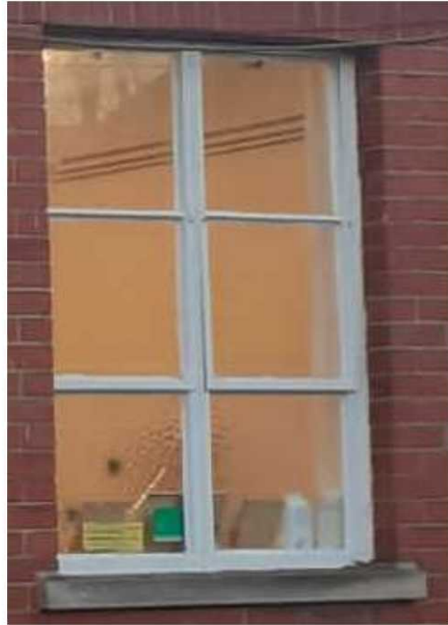
PHOTO OF EXISTING FRAME
