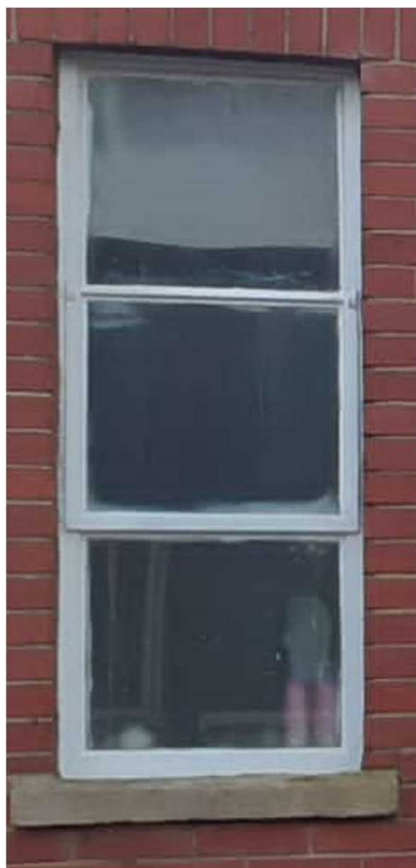
PHOTO OF EXISTING FRAME
