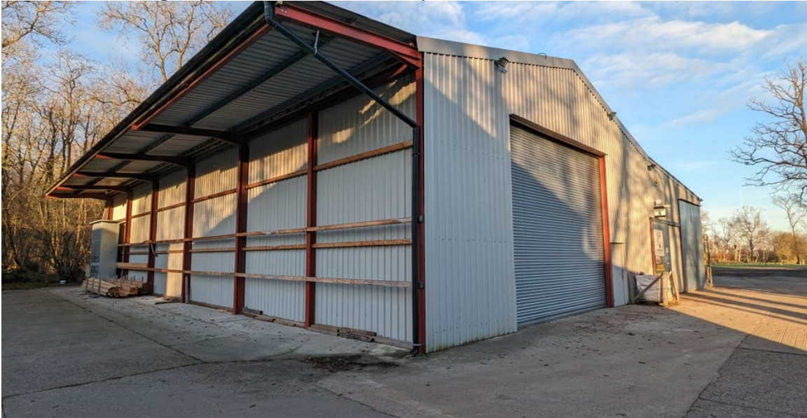
Photo of Building 3 (south & east elevation).
