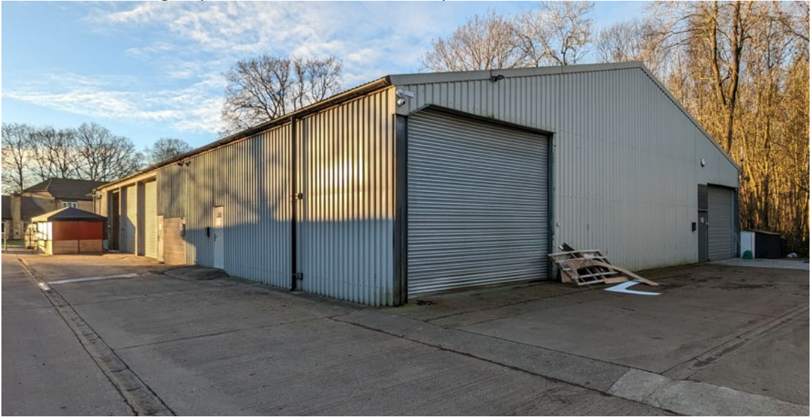
Photo of Building 1 (north and east elevation).
