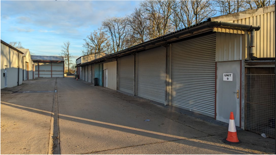
Photo of Building 4 (south & west elevation).
