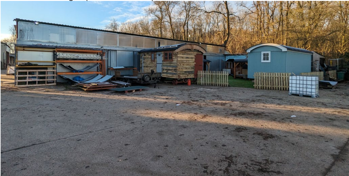
Photo of Building 3 (north elevation).
