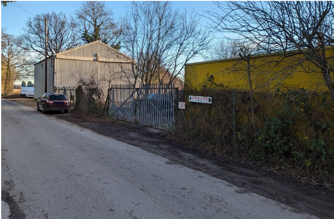
Photo of established commercial sites c.250m to the south-west of the site.
