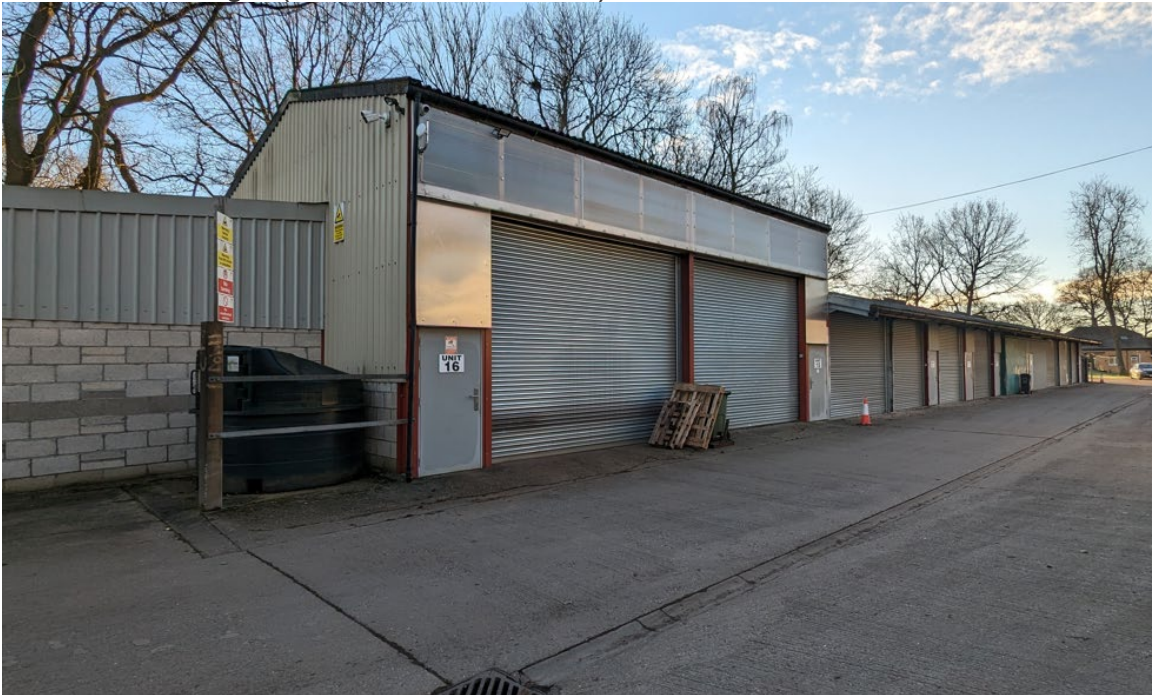
Photo of Building 4 (north & east elevation).
