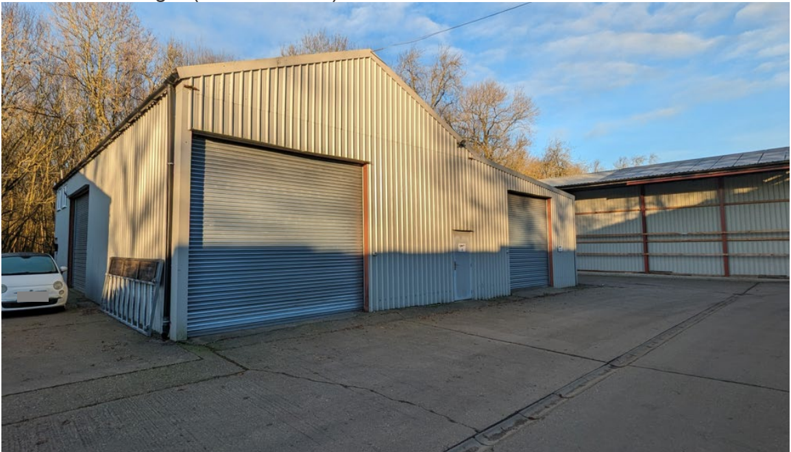
Photo of Building 2 (east elevation).
