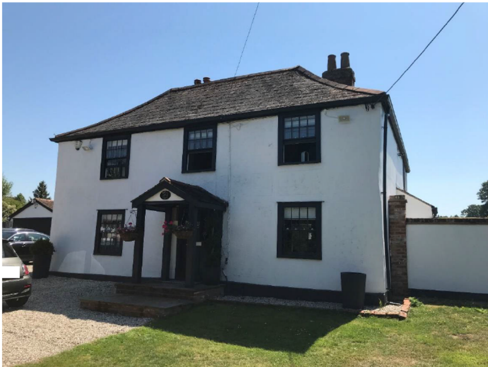
Figure 13 - Front (north) elevation of Bell Farmhouse.
