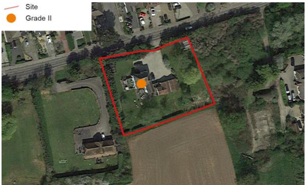
Figure 12: Aerial demonstrating the location of Bell Farmhouse
