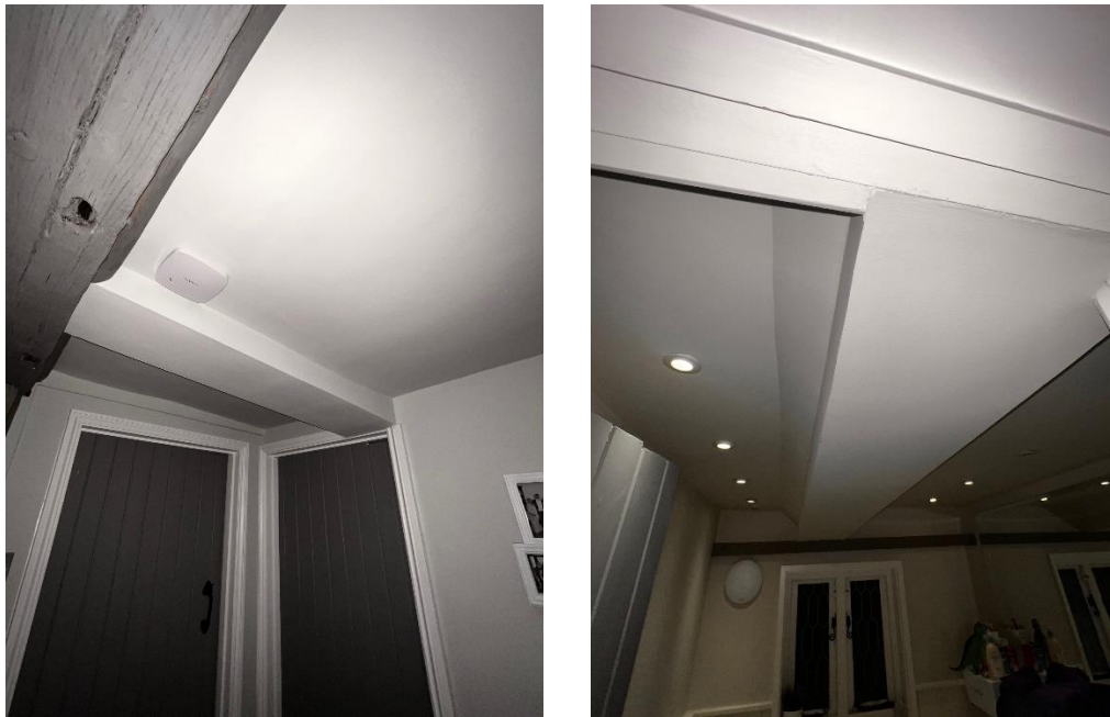
Figure 19 – Bulk heads at first floor
