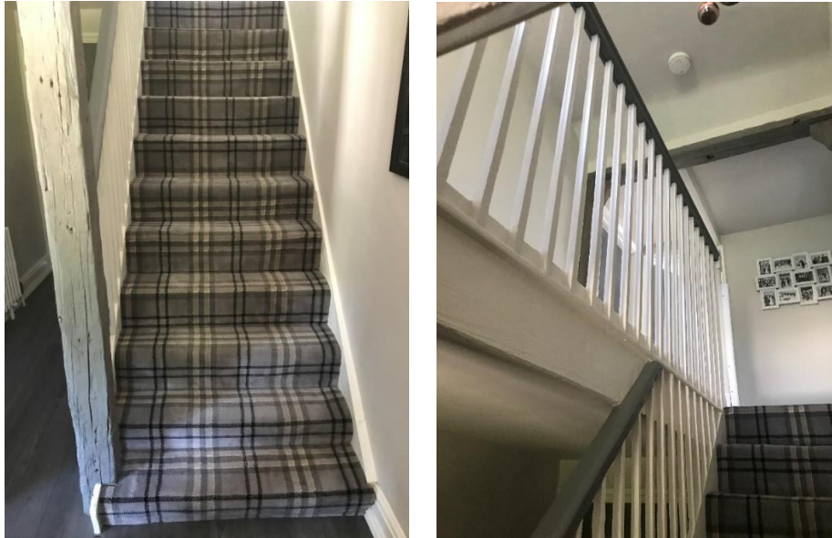
Figure 18 Staircase in central hallway.
