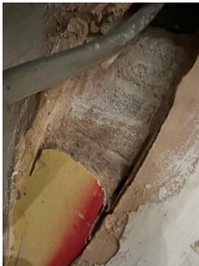
Figure 17 – Exposed breeze blocks within the kitchen extension. The first shows the eastern wall and the second the western wall.
