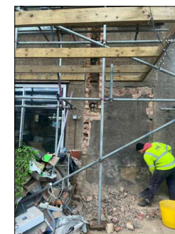
PICTURE SHOWS REMOVED CHIMNEY AND COAL ROOM
