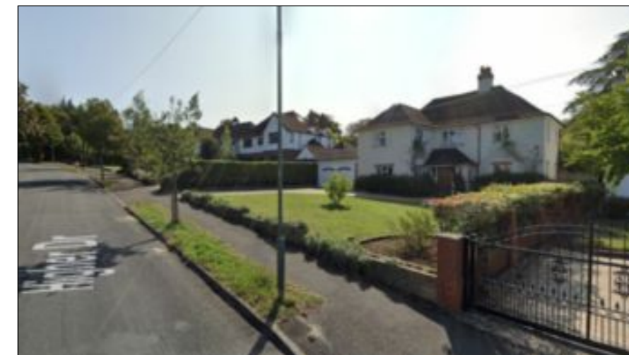
EXTERNAL VIEW OF No 35 HIGHER DRIVE ALLOWING DIRECT FIRE BRIGADE ACCESS AND SAFE ASSEMBLY POINT
