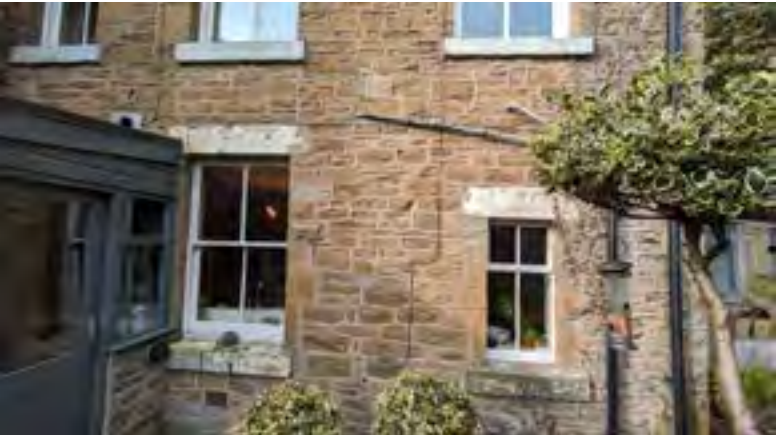
Rear wall of no.4 Ashfield Terrace
