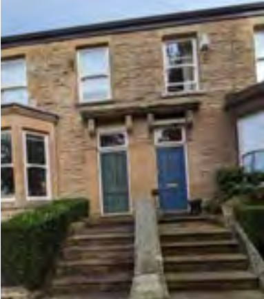
View of raised steps to entrance
