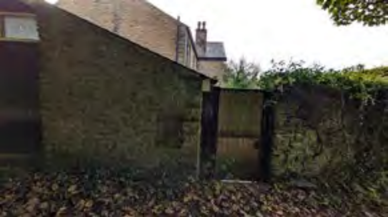
Rear gate to Apple Lane from No. 2 Ashfield Terrace
