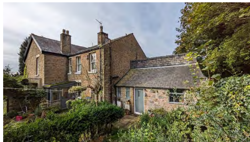
Figure 2 – Rear View [Source: Site Photos]
