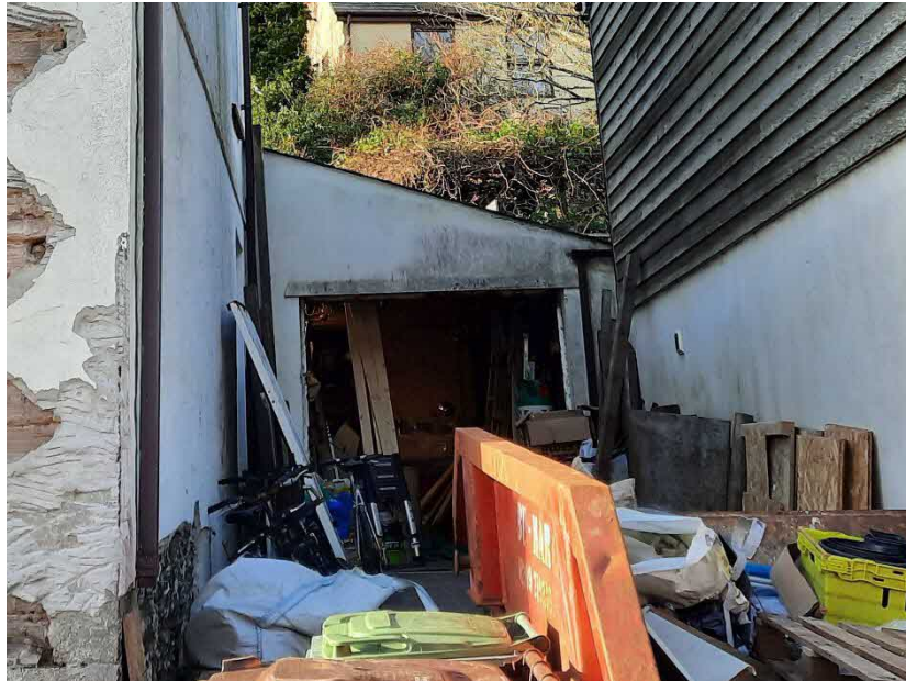
Figure 2: View of the eastern elevation of the garage at Derna House.
