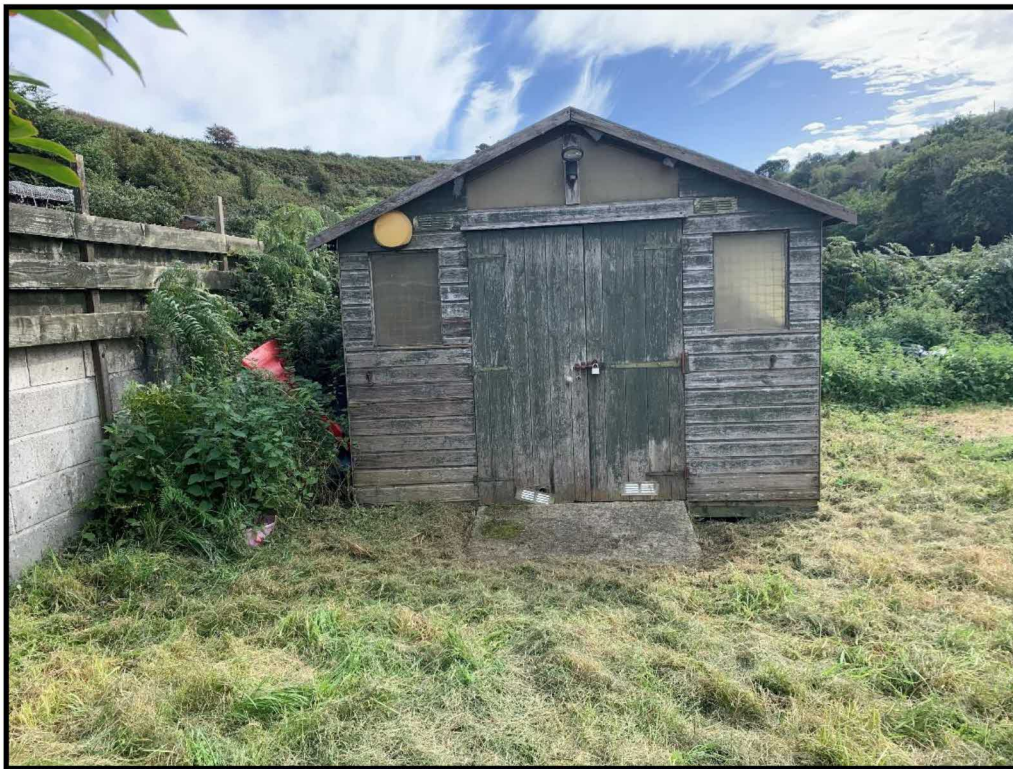
Photograph 9 - View of the shed in the southeastern corner of the site.
