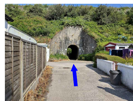
PHOTO P04 VIEW OF ARCH THROUGH RAILWAY EMBANKMENT
