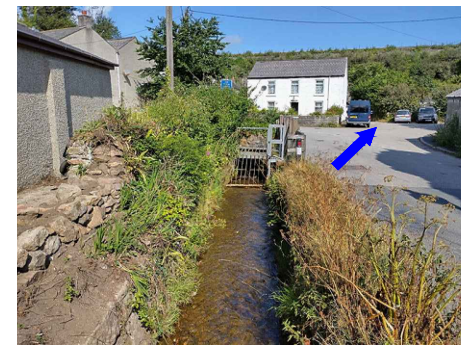
PHOTO P01 VIEW ALONG OPEN CHANNEL TOWARDS BREA VILLAGE SCREEN
