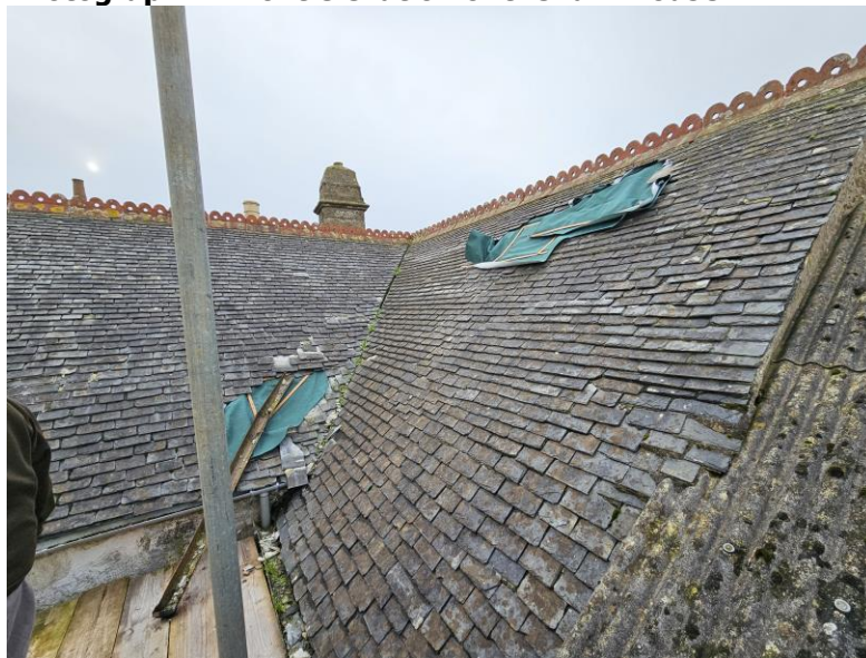
Photograph 2: Typical patch repairs
