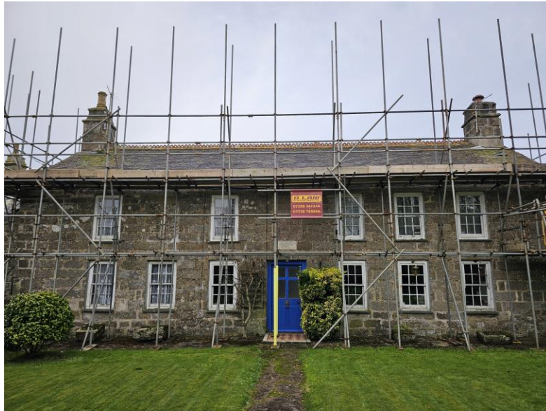
Photograph 1: Front elevation of the farmhouse
