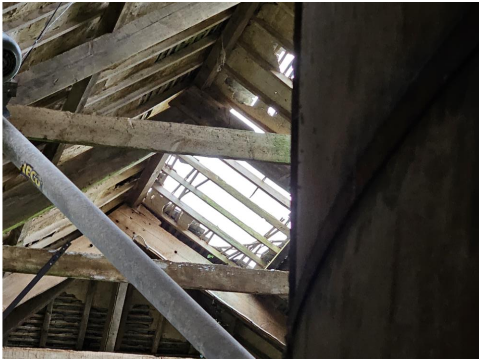
Photograph 6: Donor barn 2 roof covering condition
