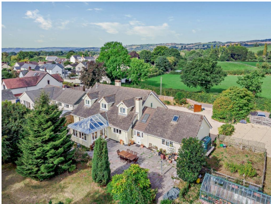
Aerial View looking North West
