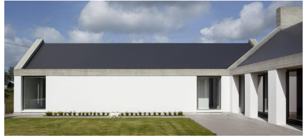
Image 3– Exemplar precedent with white render walls and fire cement roofing slates
