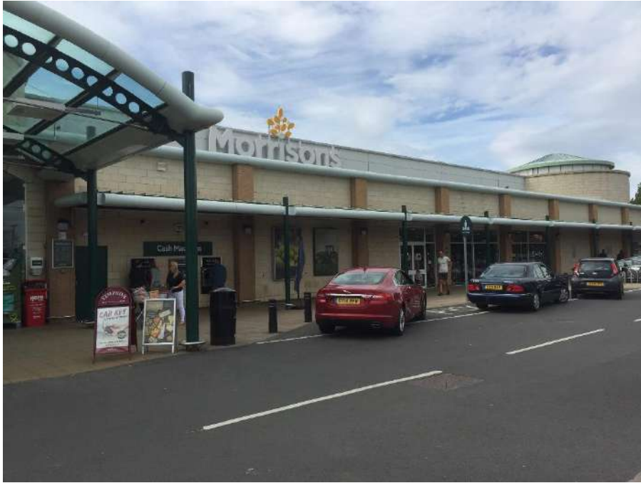
View along the North East elevation
