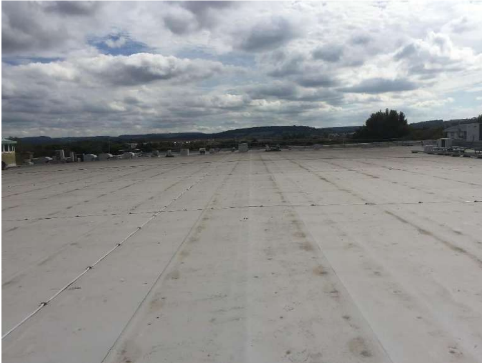
View across the roofline looking South East
