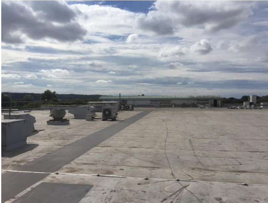
View across the roof looking West onto the first floor plantroom
