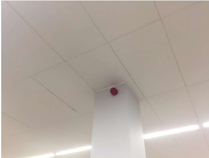
Lightweight ceiling seen throughout the store
