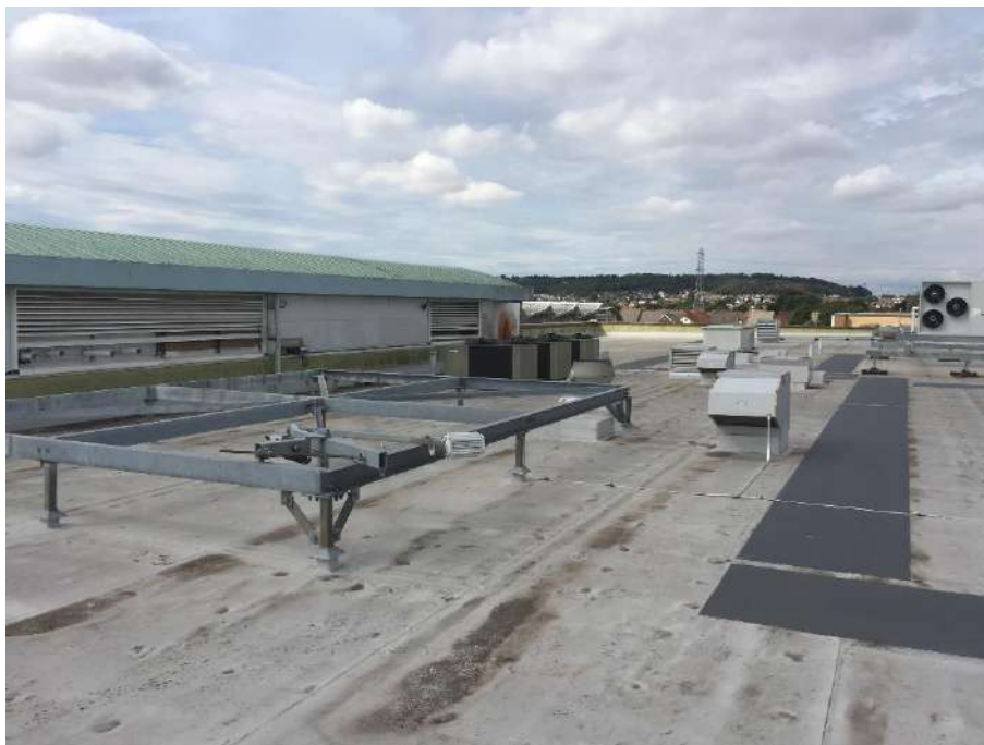
View along the rear of the first floor plantroom
