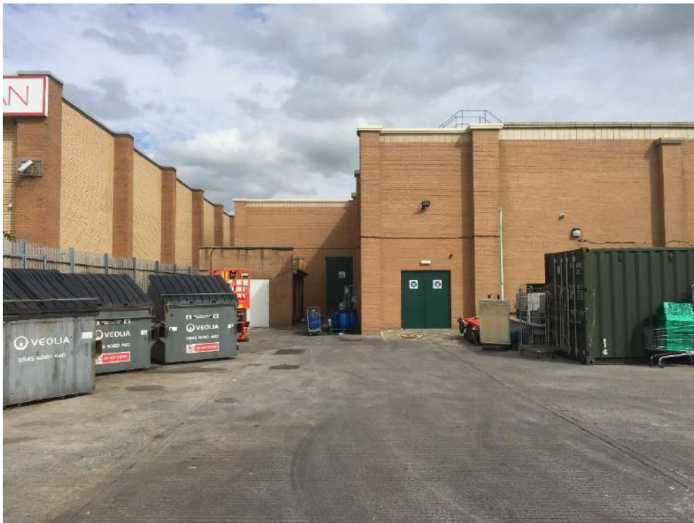
View on the South West elevation looking onto the store extension
