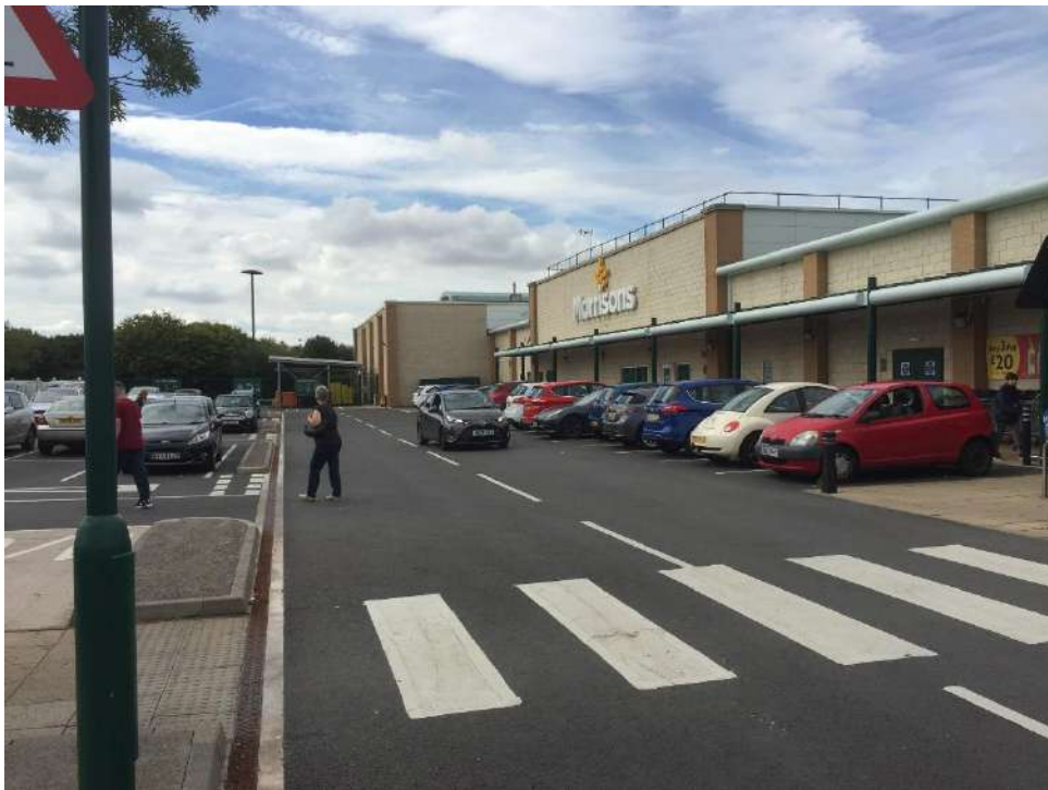
View along the South East Elevation looking towards the warehouse extension
