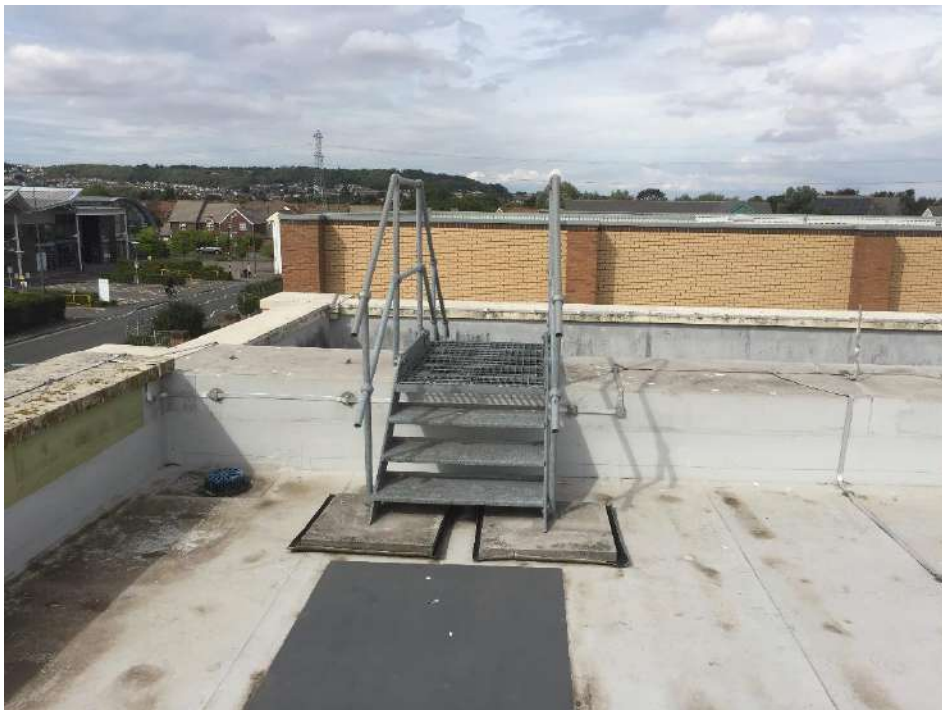
Steel stair access to the store extension roof
