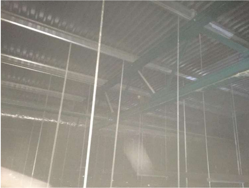
Secondary lattice truss seen above the ceiling, in the store area
