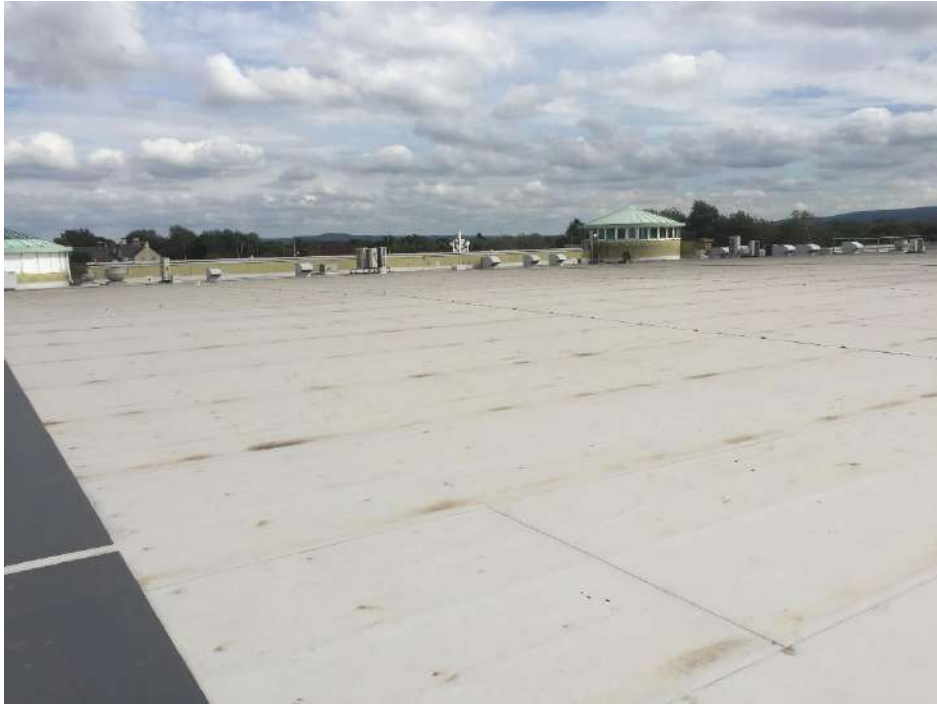
View looking East across the roof towards the Main Entrance area
