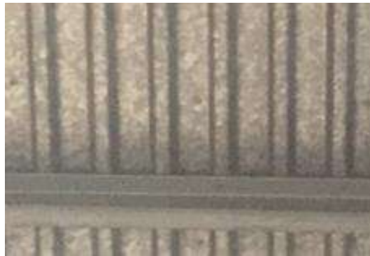
Figure 2 view on the underside of the roof deck in the warehouse
