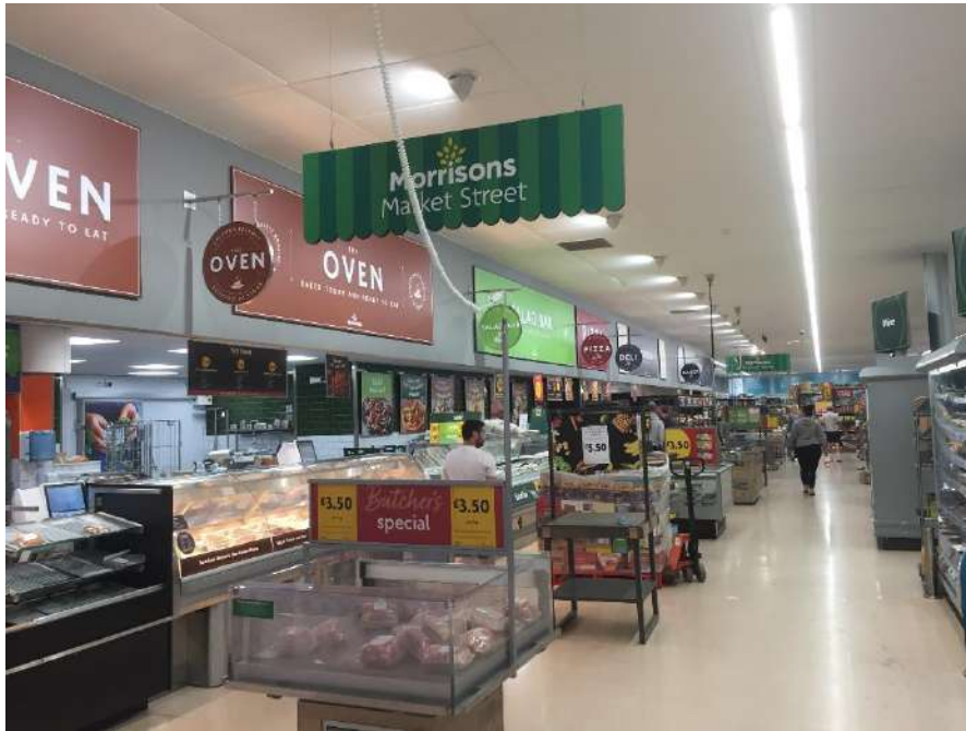
View along the bulkheads to front of the Prep Areas (parallel to the spine beams and South West elevation)
