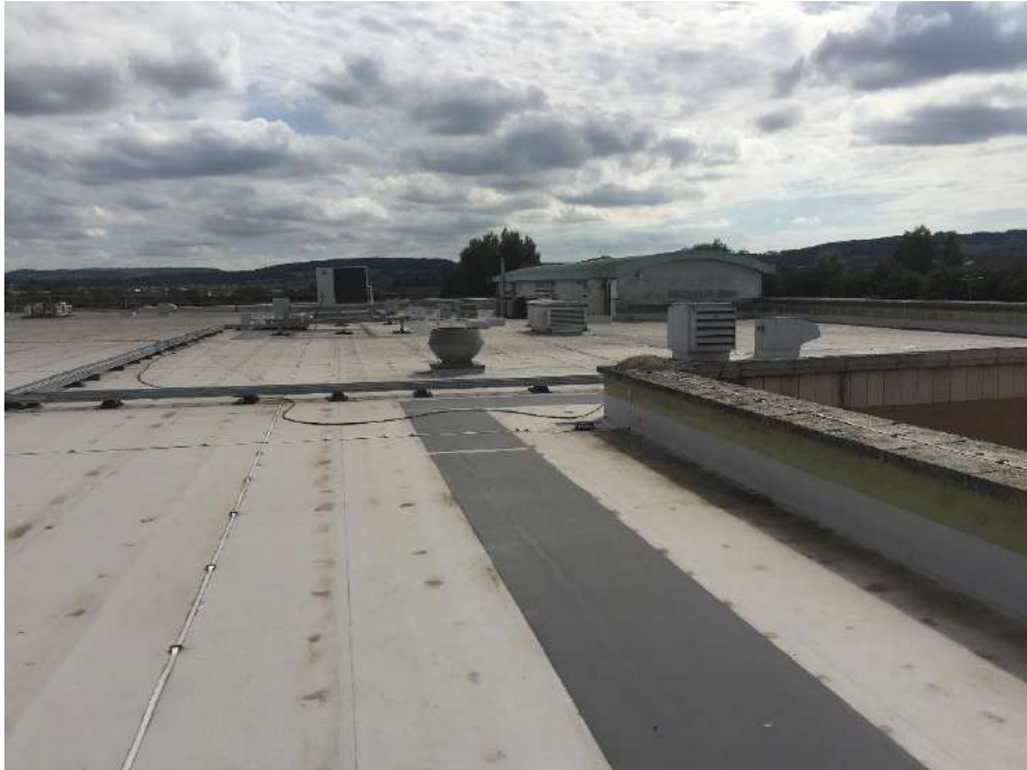
View looking North East towards the first floor plantroom
