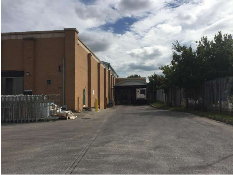
View along the South West elevation from the service yard area
