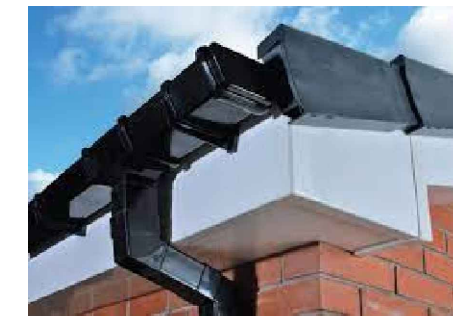
Soffits and Rainwater goods (white and black)
