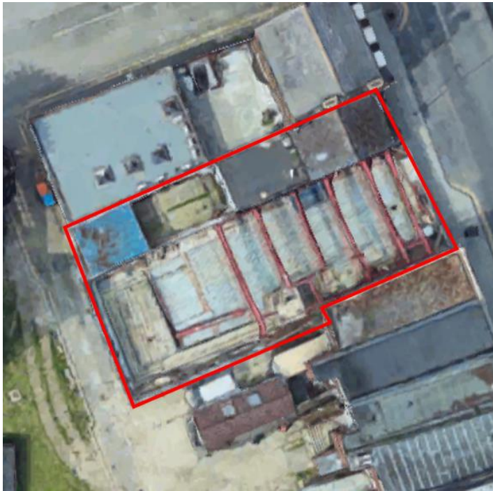
Figure 1: Aerial View of the Site (Google Maps)
