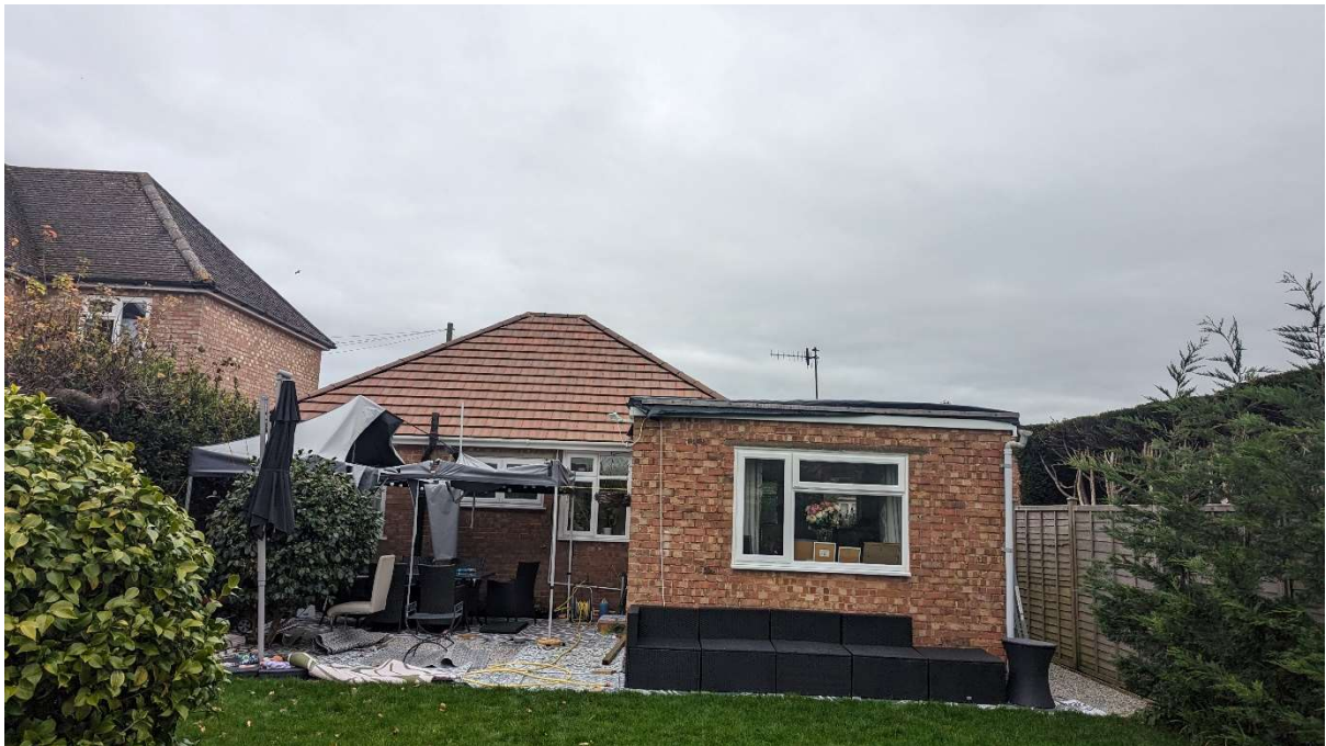
Photo 2 – View of the dwelling from the rear (south).
