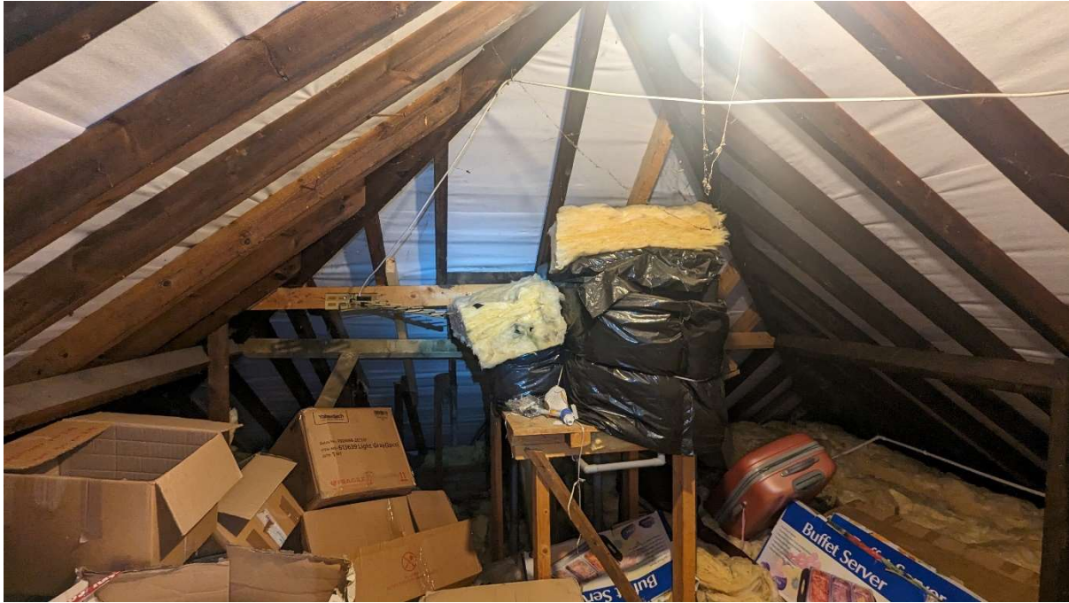
Photo 3 – View inside the loft.
