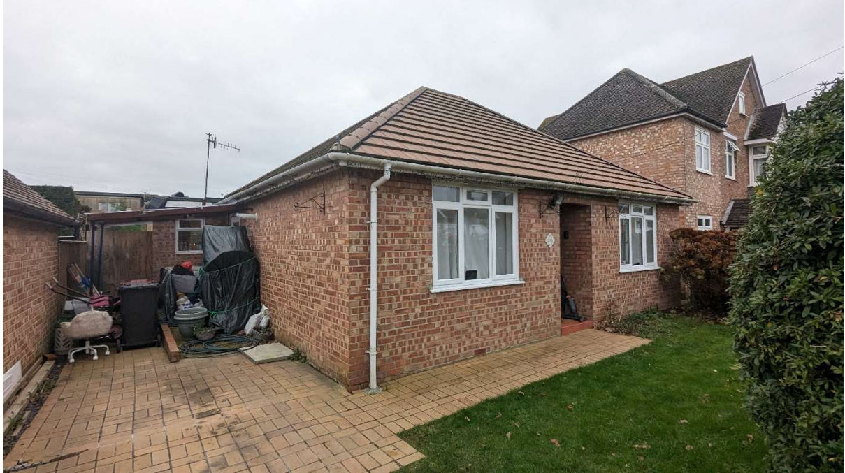
Photo 1 – View of the dwelling from the access (north-east).
