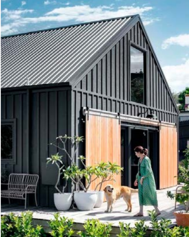
Precedent - Exposed rails & fixings
