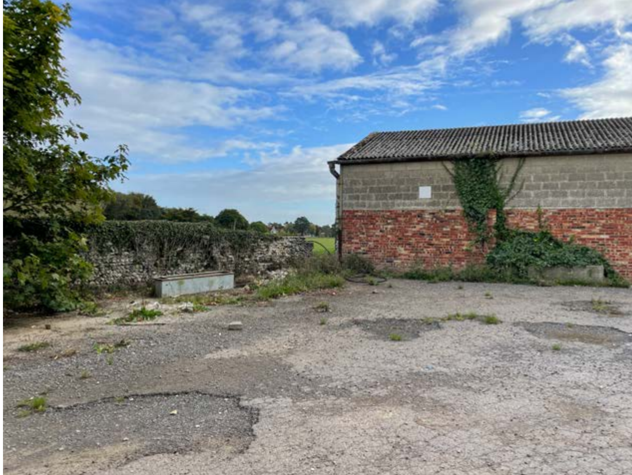
Historic flint wall which enclosed the east yard to the north
