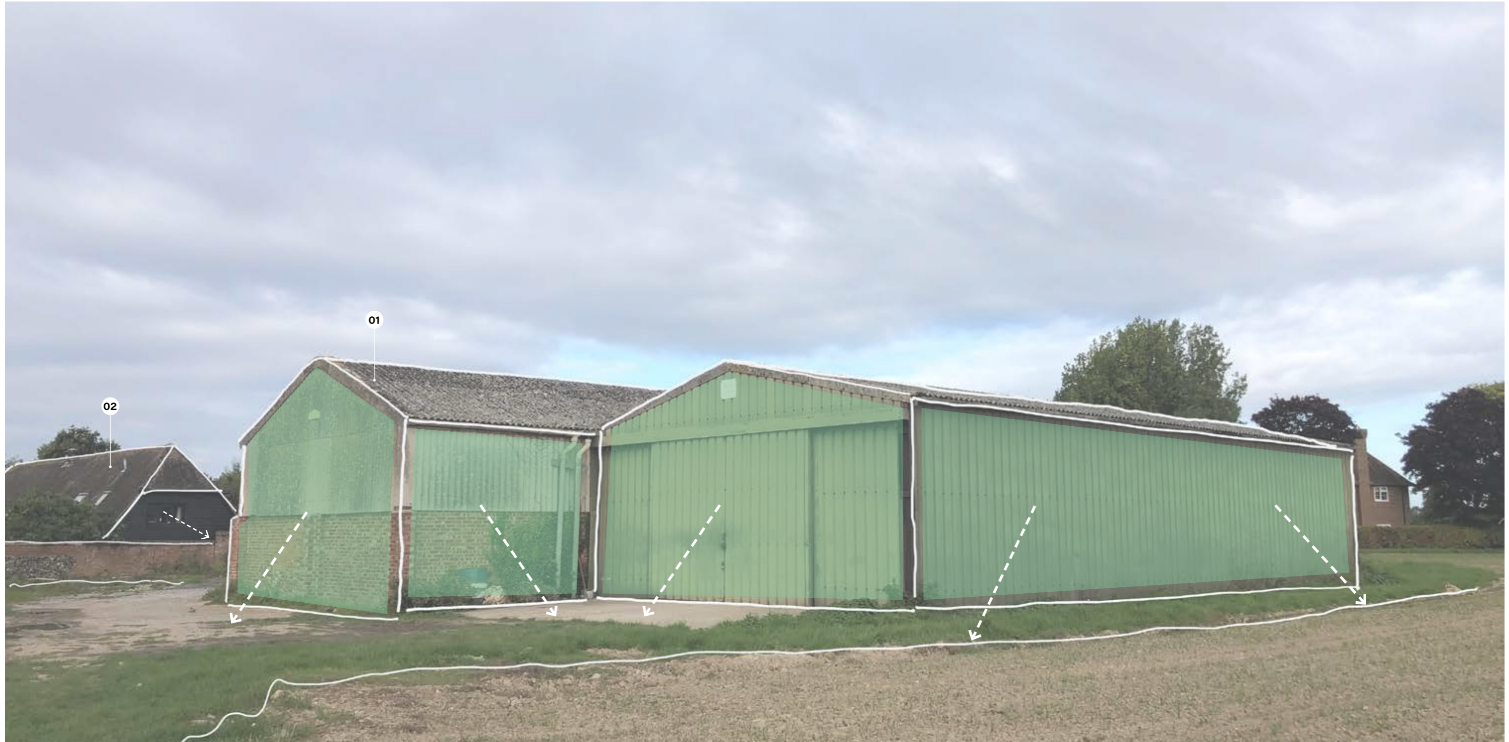
Overview photograph of east facade along Public Footpath
