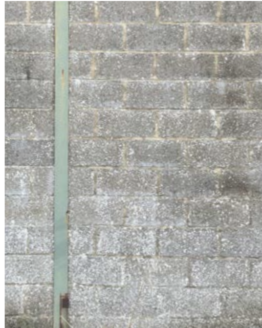
EXISTING Concrete Blockwork
