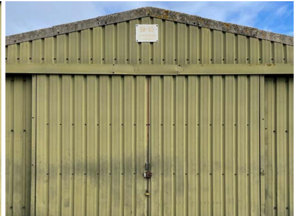
View 04: view of existing building from site south-east
