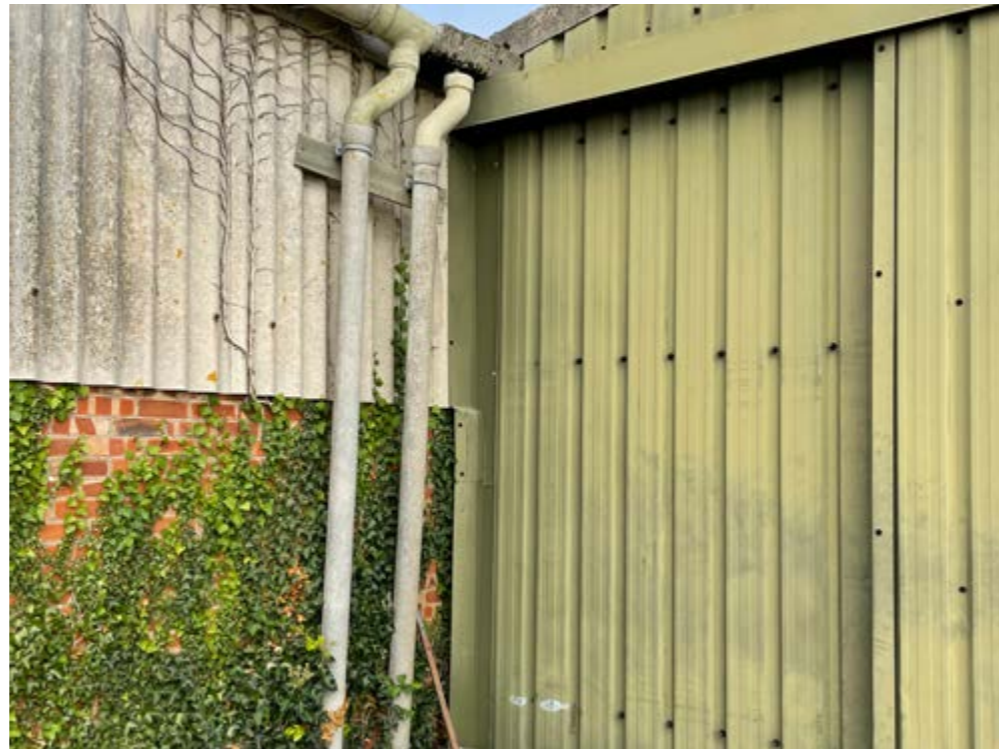
View 03: view of existing building from site south-west
