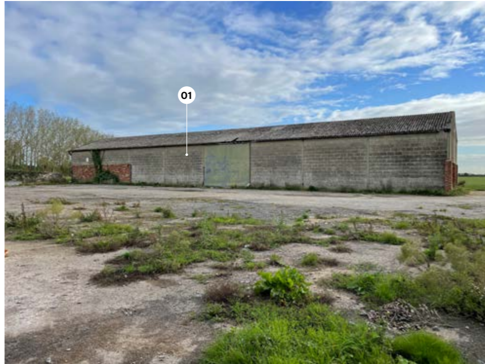
View 01: View of West Facing facade
