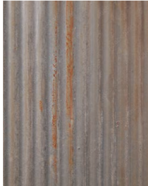
EXISTING Corrugated Metal
