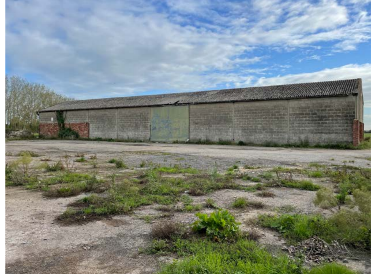
View of overall building in-situ
