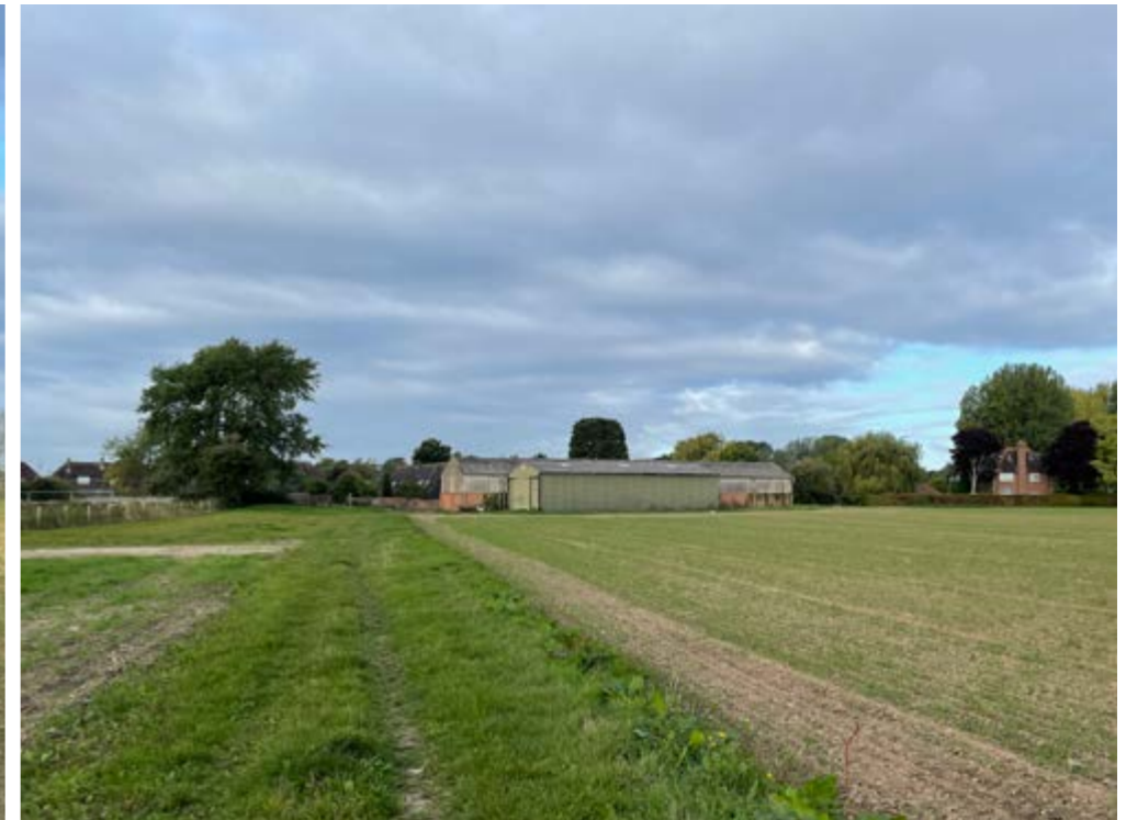
View 04: View of adjoining barns approaching from the east via public footpath
