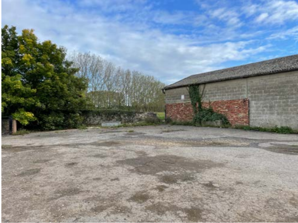
Existing view of west facing facade
