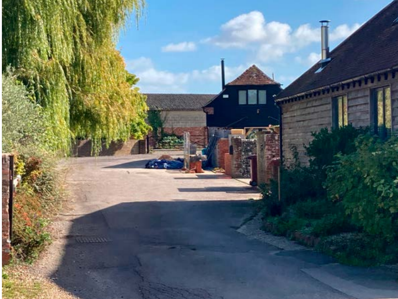
The concrete block walls are visible from within the conservation area.
