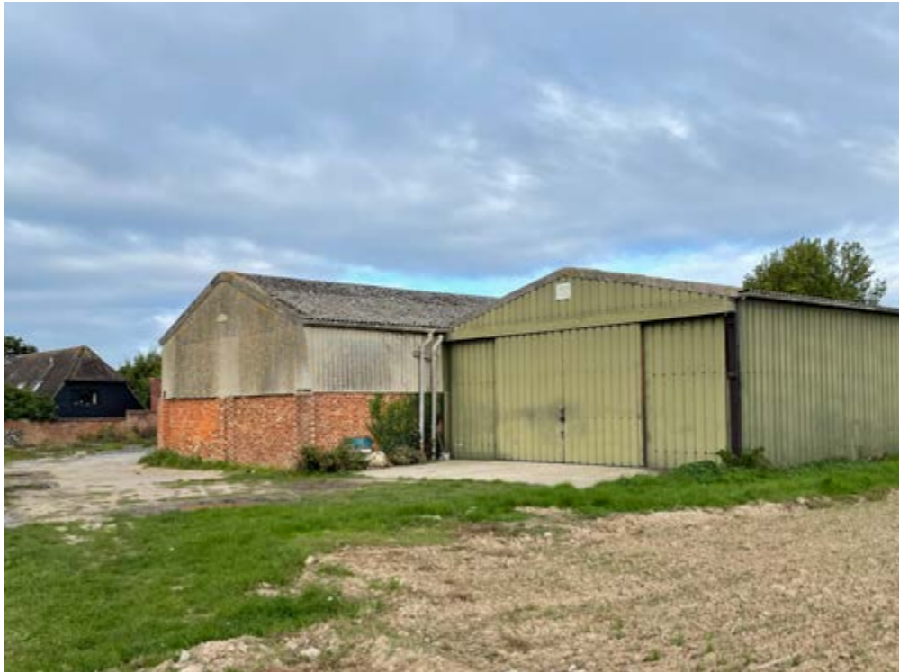
Existing view facing east side of building
