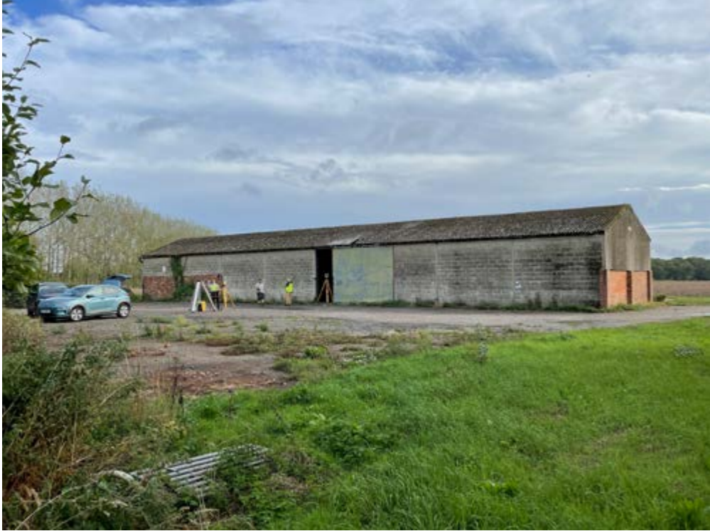
Existing view from Public Footpath facing west side of building
