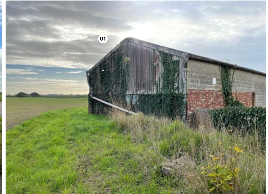
View 02: View of North Facing facade
