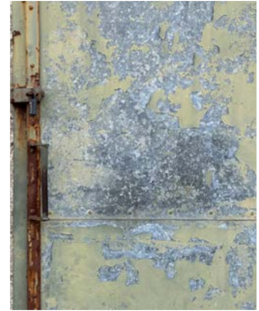
EXISTING Galvanised steel
