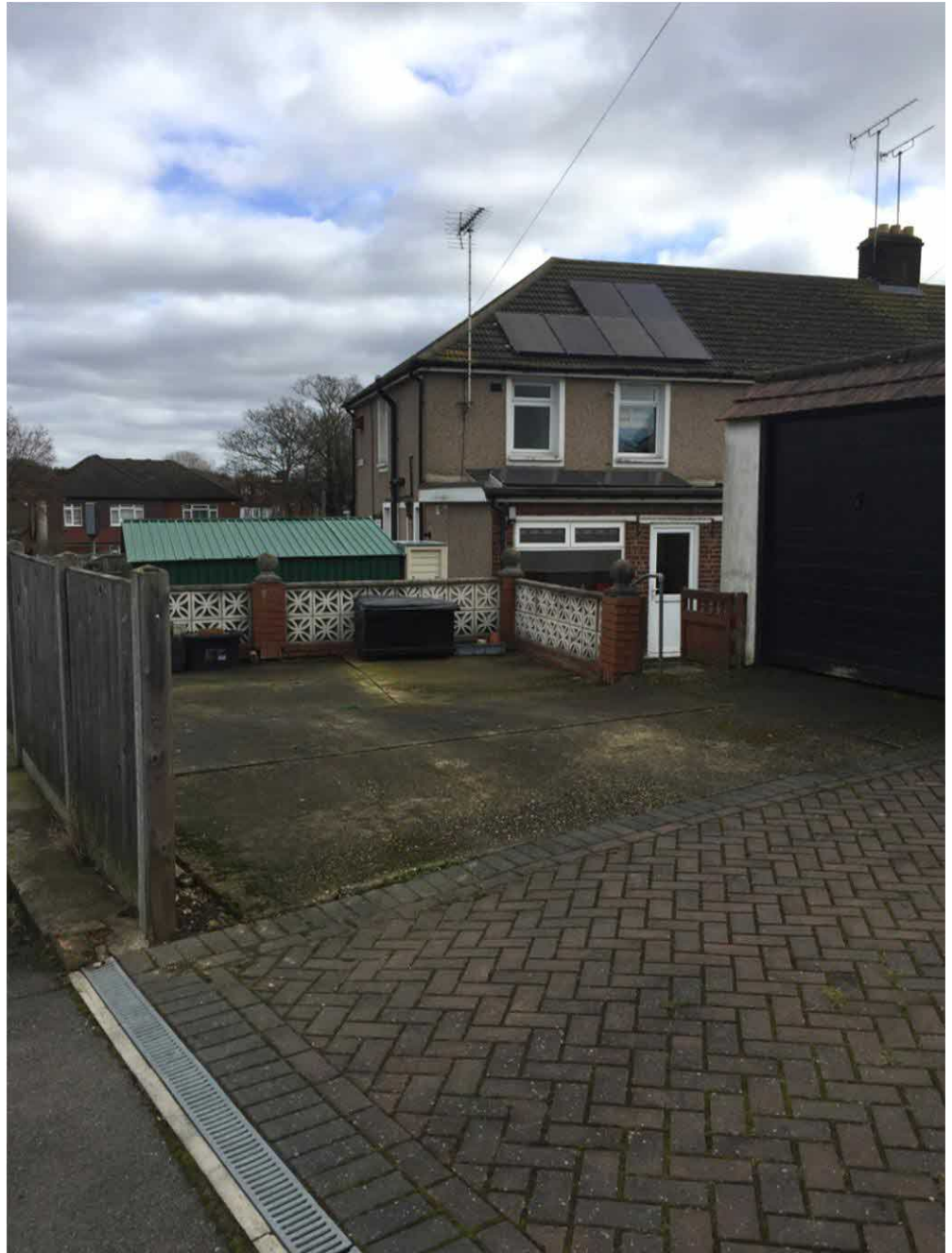
Garage at the rear to be demolished
