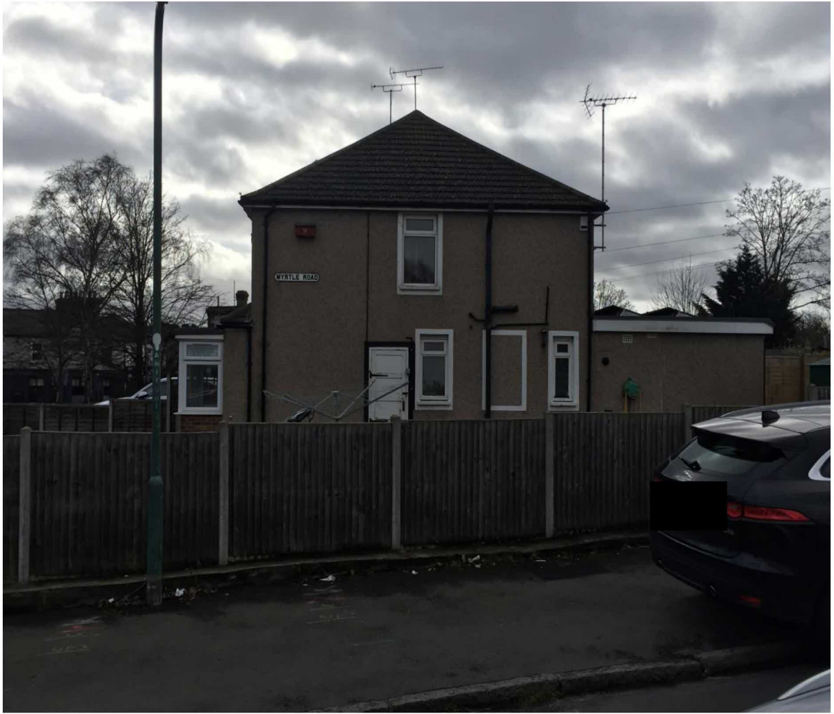
Side North Elevation as seen from Myrtle Road
