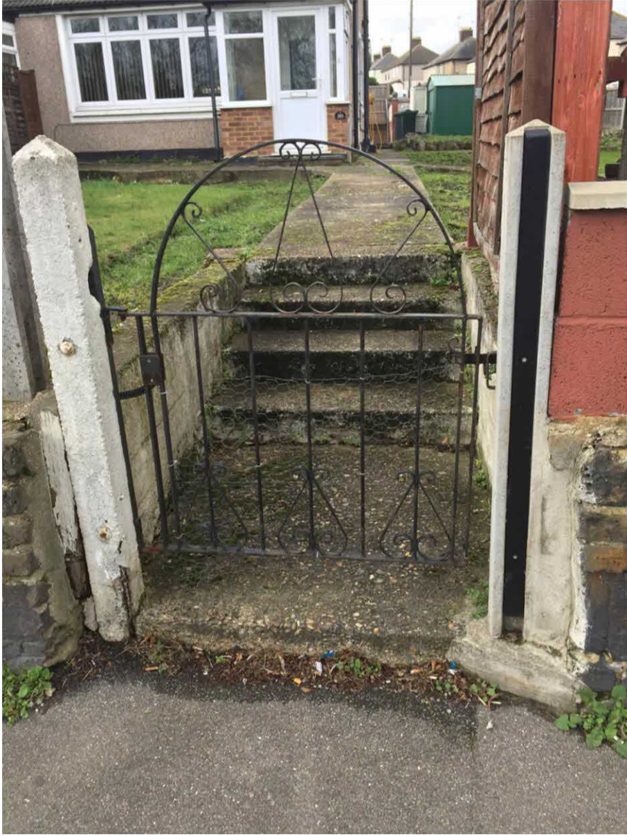
Existing Gate and steps at the front along Lowfied Street
