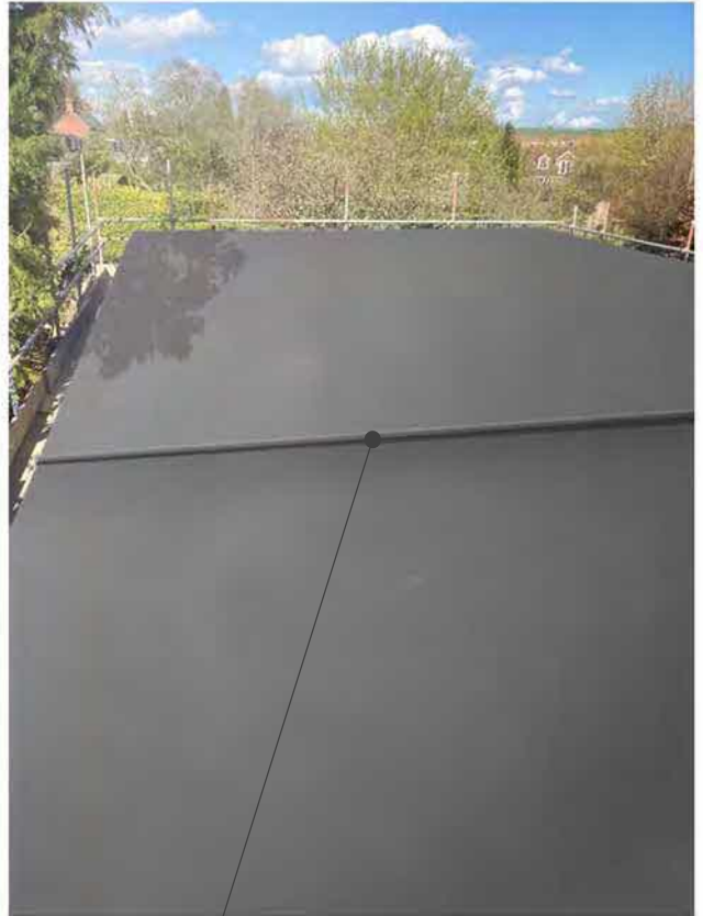
Flat Roof Finish Trim to Joint Line
