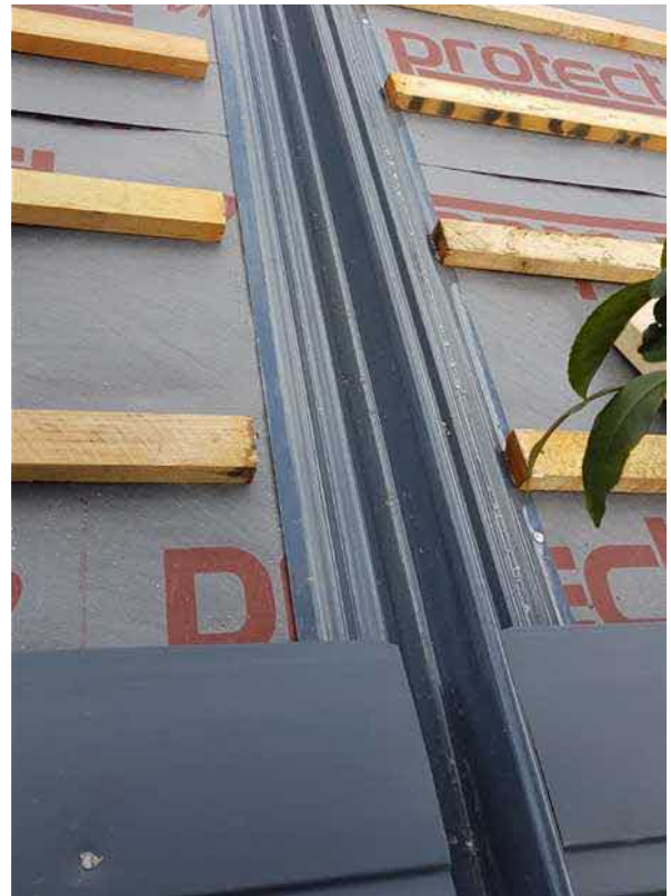
JOINT TRIM APPLIED TO PITCHED ROOF SITUATION
