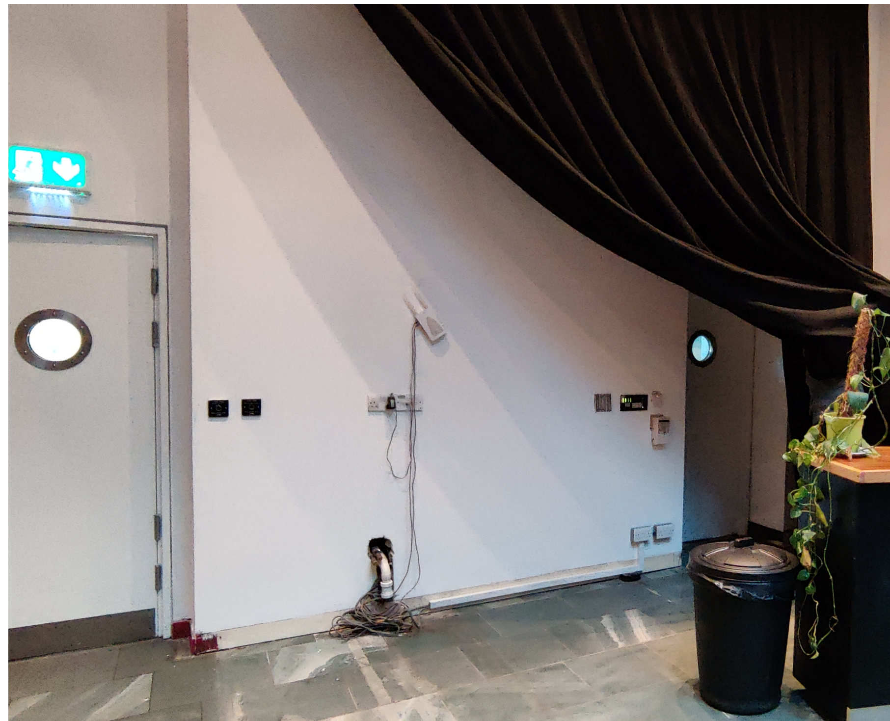
Photo of existing wall and opening
