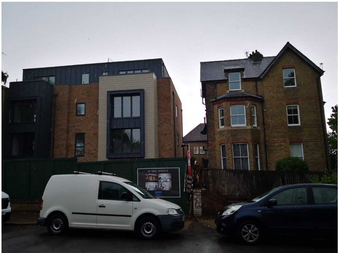
Recently built at The Avenue, adjoining the site to the north
