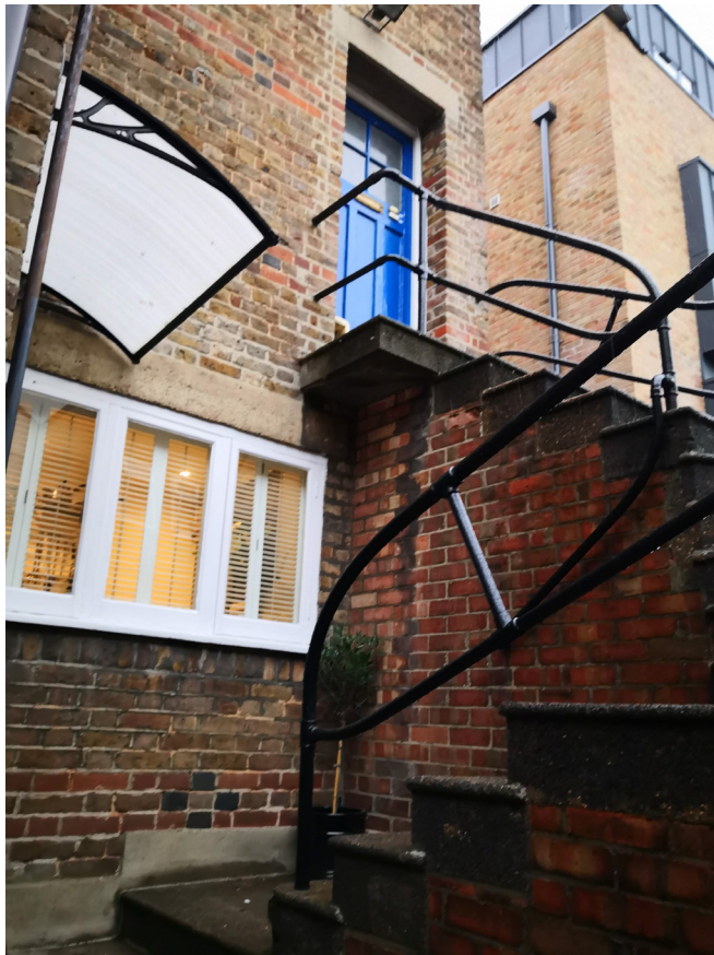
Access to the existing flats within No. 15 Avenue South, which will be removed and relocated as part of scheme
