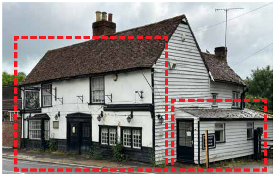
The White Horse Inn - Varying form achieved with single storey extensions from the main structure. Double doors, bay window and prominent chimney are distinct features.
