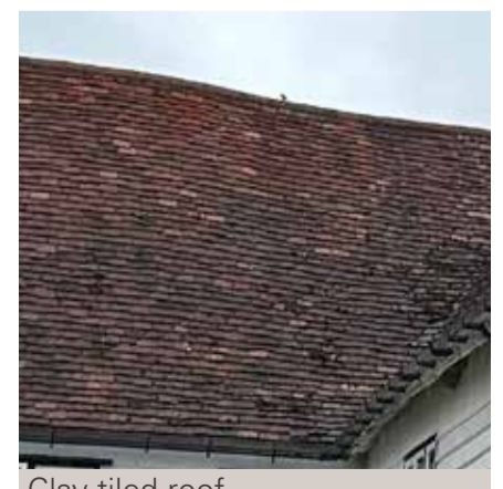
Clay tiled roof.
