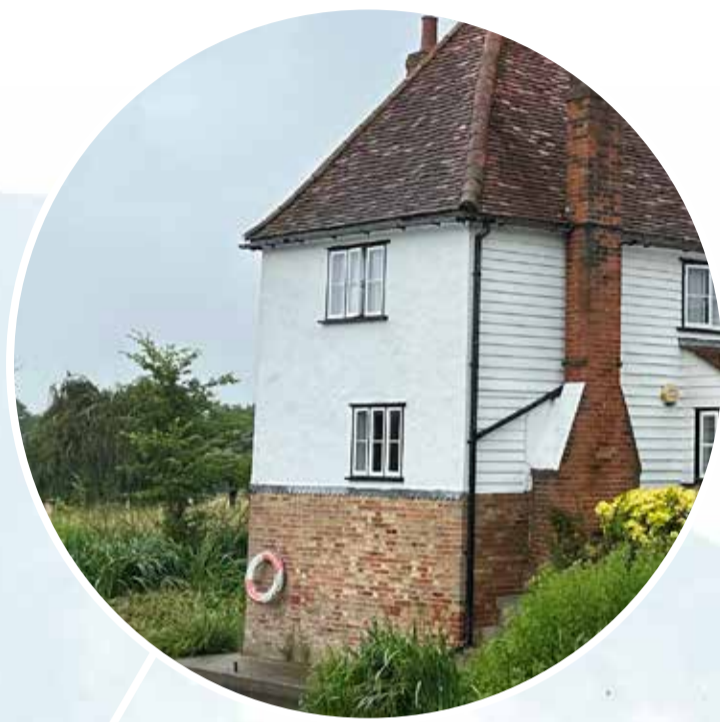
Brick sill, roughcast render and timber walls and clay tiles.
