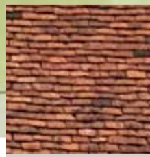
Plain tiles roof
