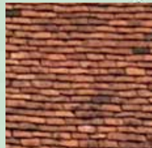
Plain tiles roof
