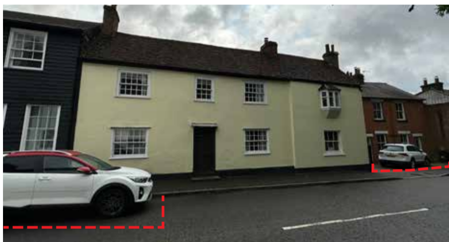
The Old Waggon (grade II*) - Continuous frontage, minimal set-back from the street and no boundary treatment.
