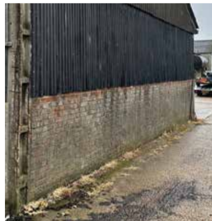
Weatherboarded walls and brick plinth.
