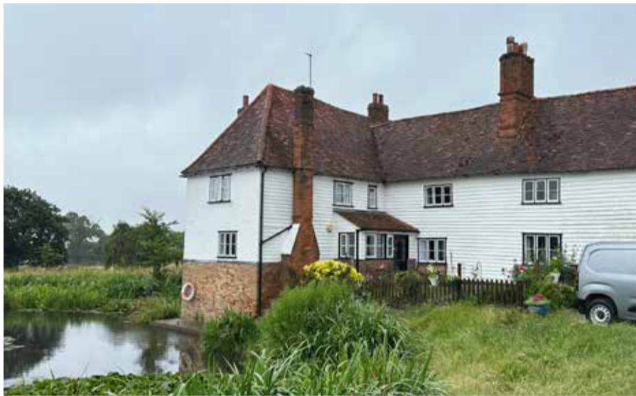
T shaped Sutes farmhouse in timber frame on brick sill and white weatherboarded.
