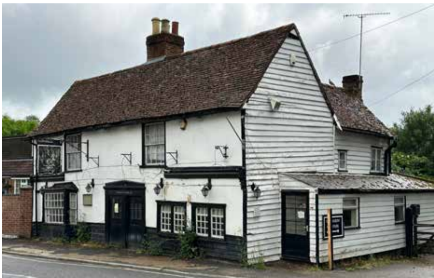
Former coaching house timber frame rendered with weatherboarded wing / side and boarded apron.
