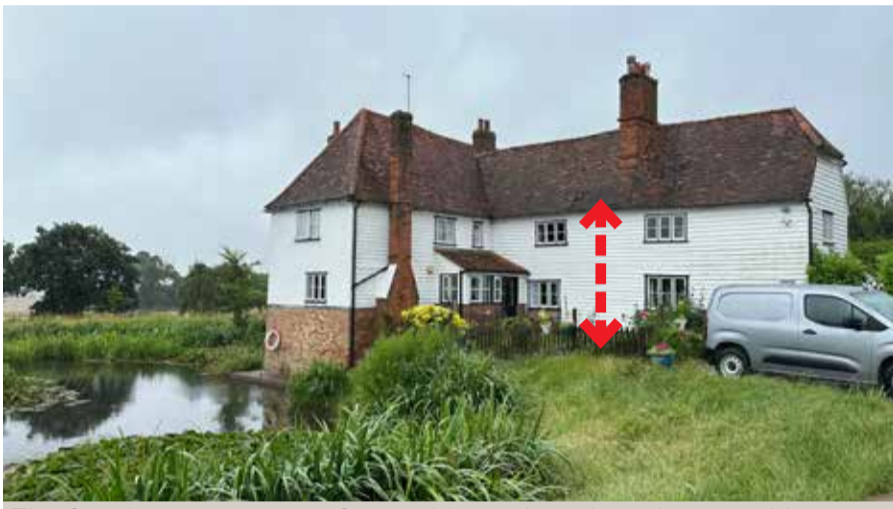
The farmhouse- 2 storey form with north and north-west sides rising from the moat.
