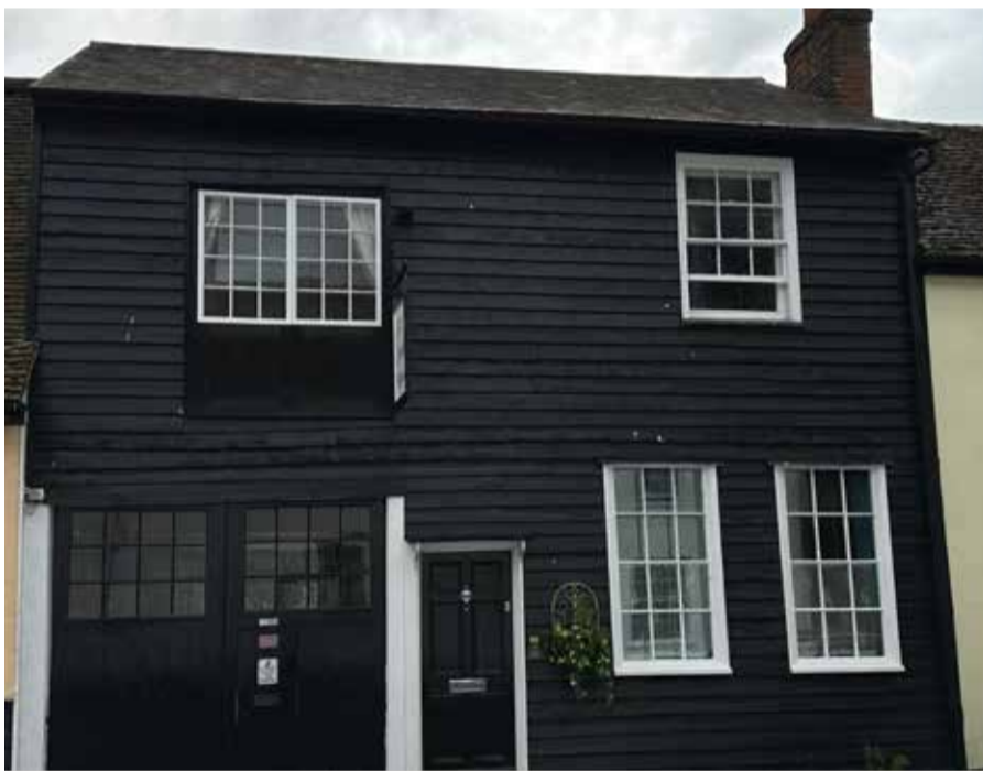
Coach House - example of former Coaching Inn with wide carriageway through to rear yard closed by a large double door.
