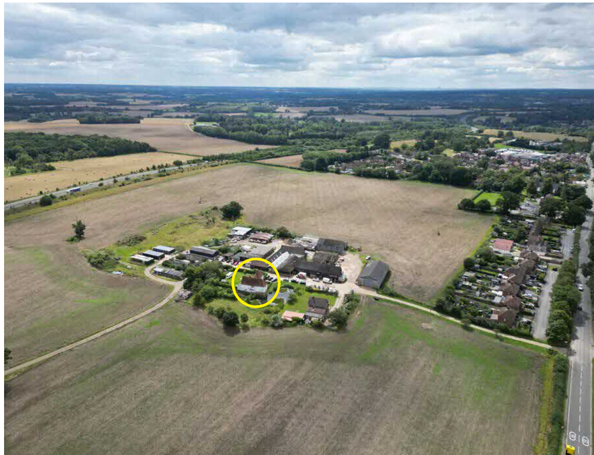
Figure 4.3. Aerial image showing the farmstead and its surroundings from the north, with the farmhouse circled in yellow. The driveway entrance from the High Road is evident, and the modern farm buildings to the south provide an evident visual barrier between the listed building and the land beyond.
