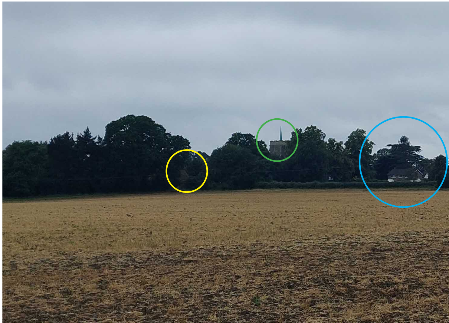
Figure 4.11. Looking from the Site to the south, with the top of the Church of St John the Evangelist visible above the tree canopy within the green circle. The yellow circle contains the location of the northern elevation of the garage of the Rectory, with the dense foliage screening any further visibility of the Rectory's plot. The blue circle indicates the primary school plot, with the listed element to the west mostly hidden behind the rest of the modern structures.
