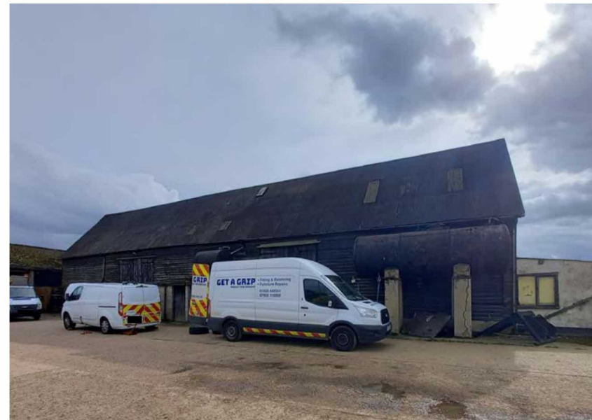
Figure 4.5. The northern elevation of the Barn.
