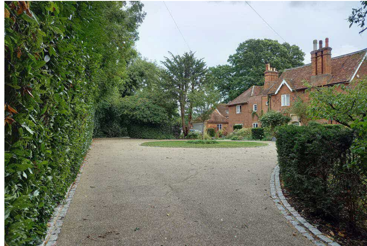
Figure 4.10. Front elevation of the Rectory, from the entrance to its driveway.
