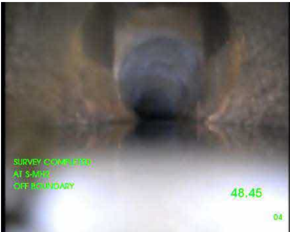
SMH1X_9ec9ca48-520a-4286-9957-903a5a0b1306_20231019_220044_228.jpg, 00:06:30, 48.45 m Finish node, manhole, reference: LINE X
