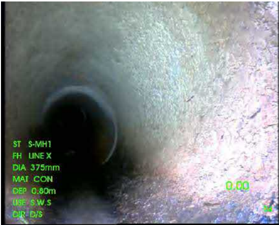
SMH1X_b95f4870-4fa2-426a-8192-8b1cd1919709_20231019_215355_061.jpg, 00:00:00, 0.00 m Startnode, manhole, reference: SMH1
