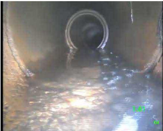
SMH1X_2d5870d9-fb26-4858-88ba-4e31f1436847_20231019_215422_796.jpg, 00:00:27, 1.61 m Water level, 15% of the vertical dimension
