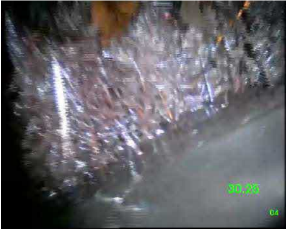
SMH1X_c5a0ea96-cb5c-4a7b-a4e3-b509a4127004_20231019_215949_612.jpg, 00:03:30, 30.25 m Roots, mass, 60% cross-sectional area loss
