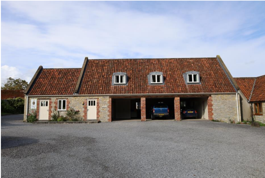
PHOTO 1: Front facing South elevation.
