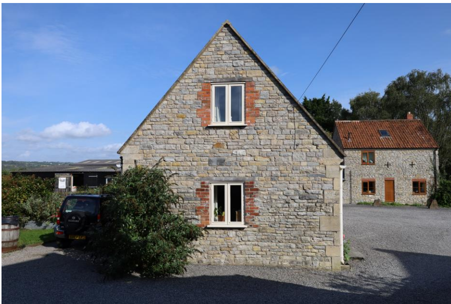
PHOTO 2: Part side East facing elevation.
