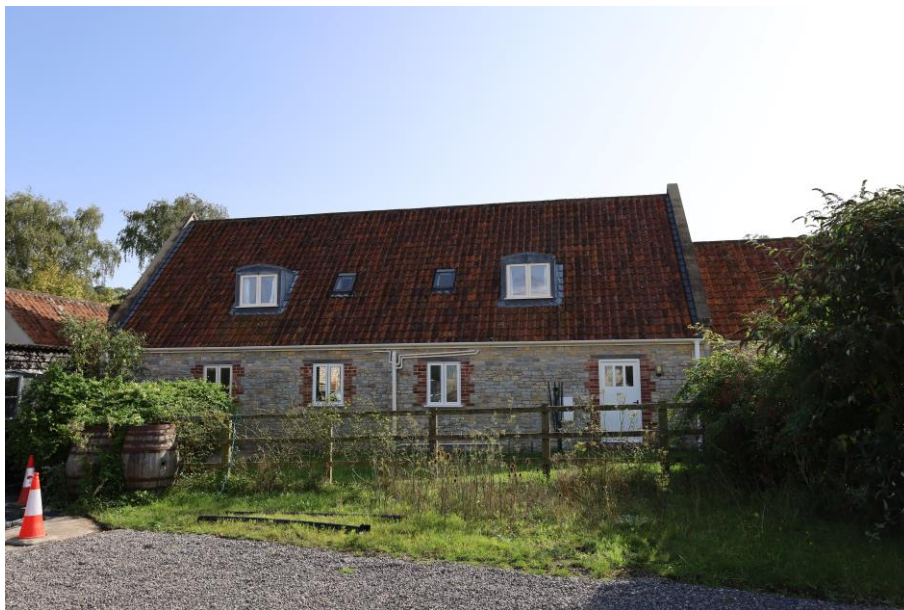
PHOTO 4: Rear North facing elevation.
