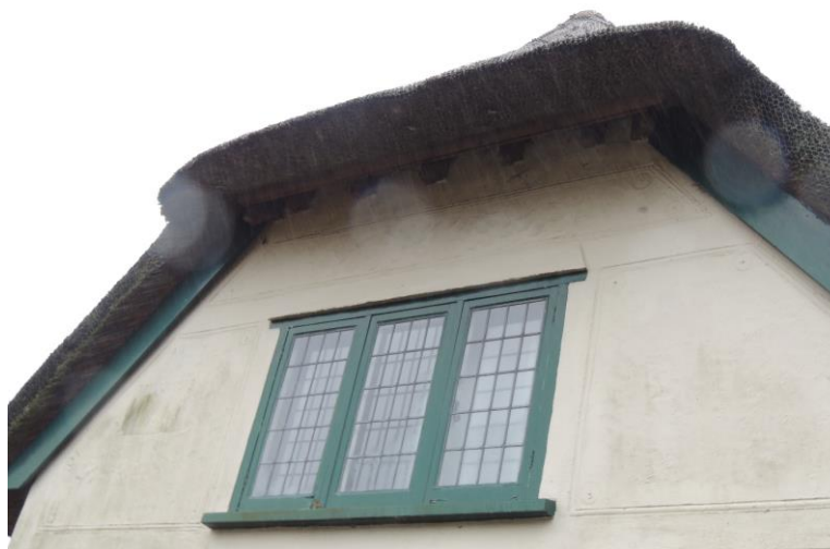
Photo 3: Showing tight seal to eaves
