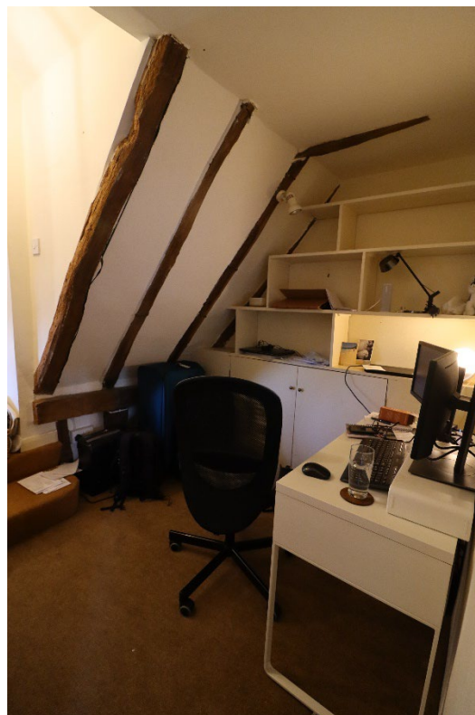
Figure 8. Existing study space at first floor that forms part of corridor. The ceiling and partitions are all C20th formed when the rear extension was added to the cottage. Some of the 'original' rafters have been retained. A new timber stud partition is proposed to form a separate first floor bathroom off the landing.
