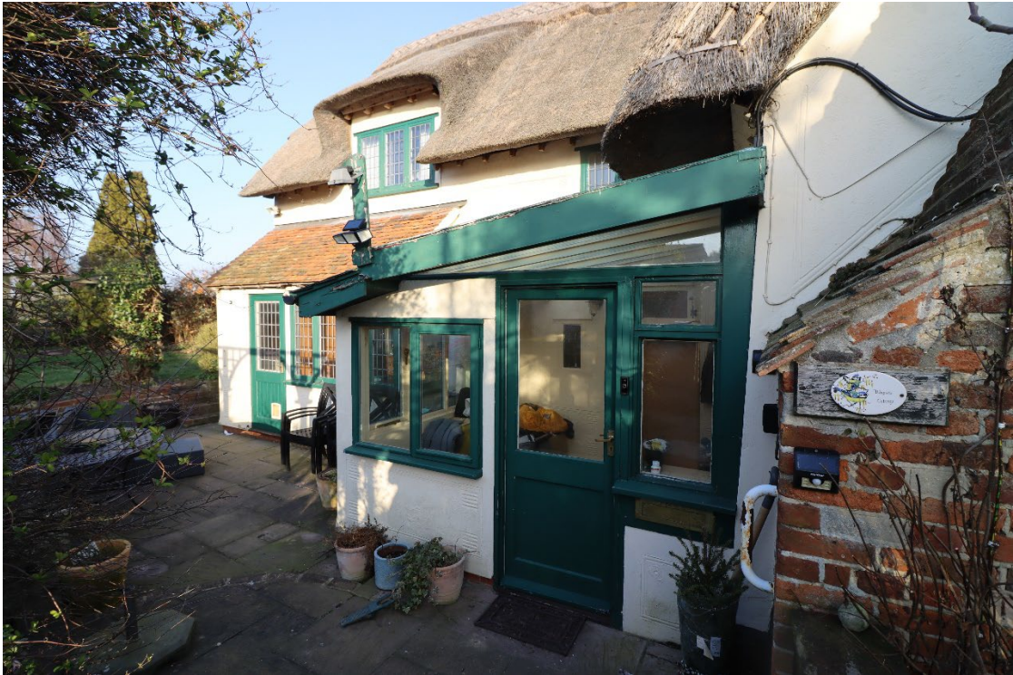
Figure 3. View looking east towards C20th side lean-to porch with two storey C20th extension in background. Porch to be removed and replaced with smaller external porch, distanced away from walls of original cottage.
