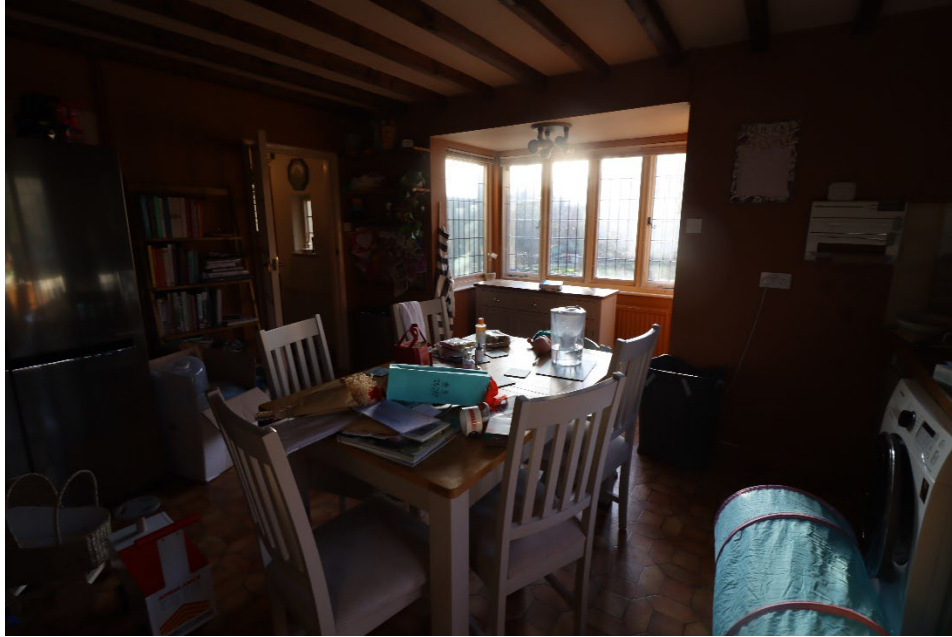
Figure 7. View within existing kitchen and C20th part of cottage where internal partition is to be removed as part of works and the existing glazed lean-to extended.
