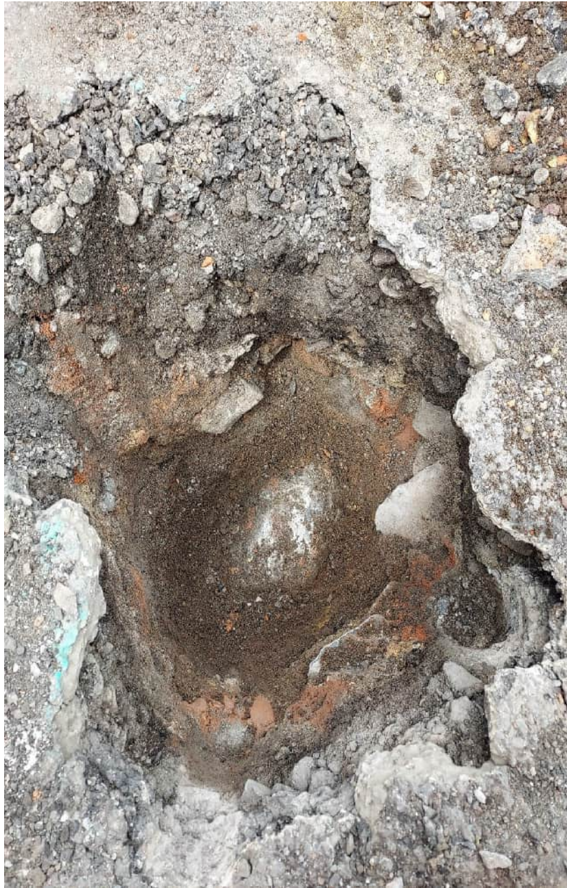
BH103 Inspection pit_2
