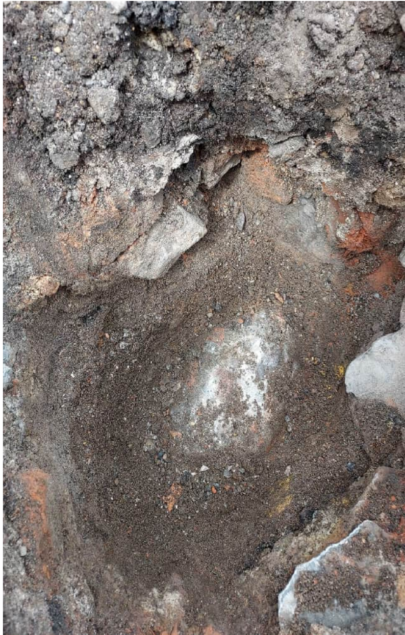
BH103 Inspection pit_1
