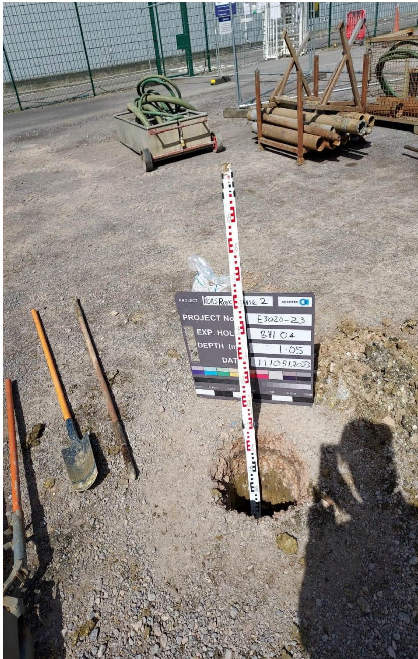
BH104 Inspection pit
