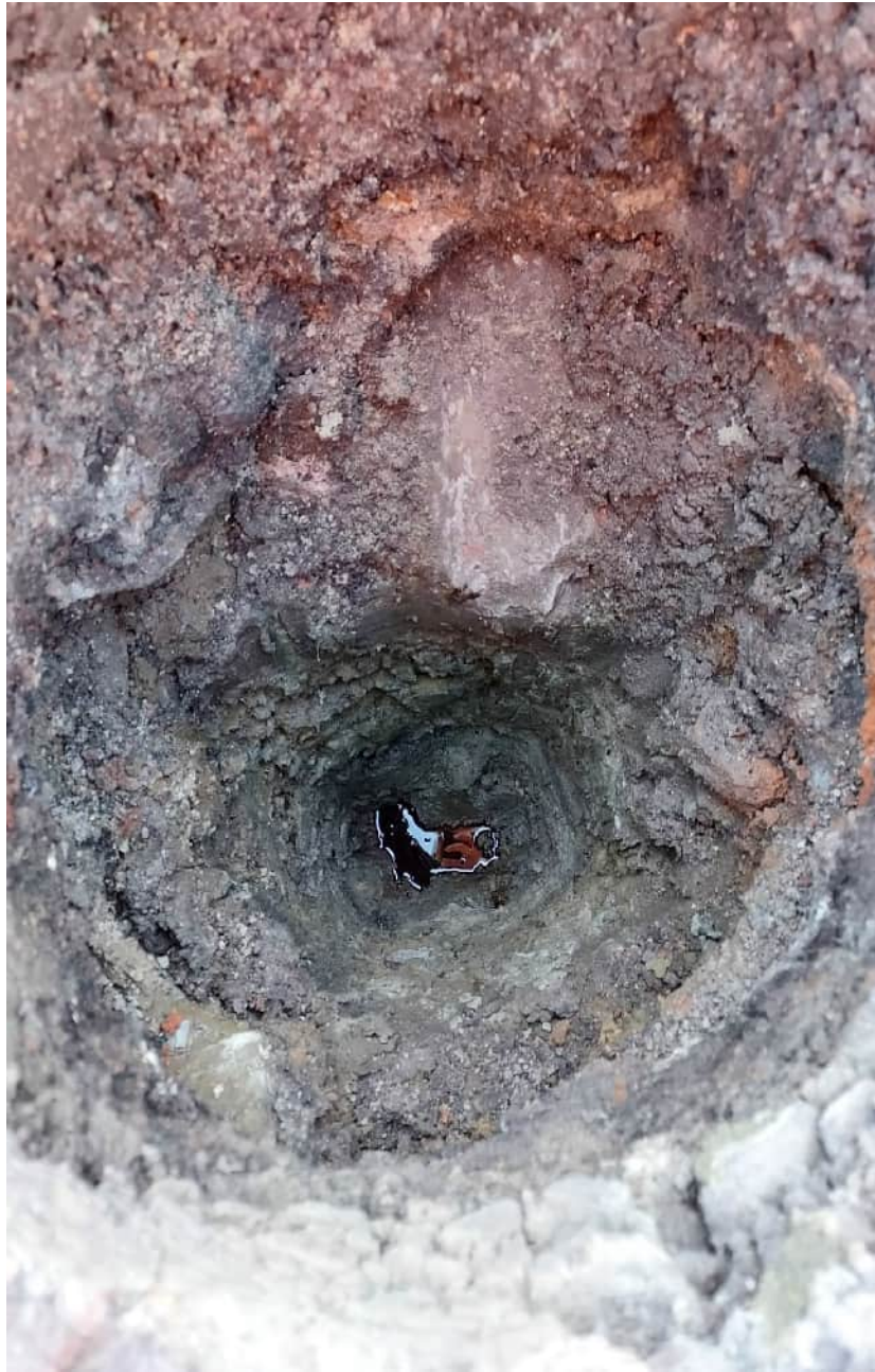
BH103A Inspection pit_2
