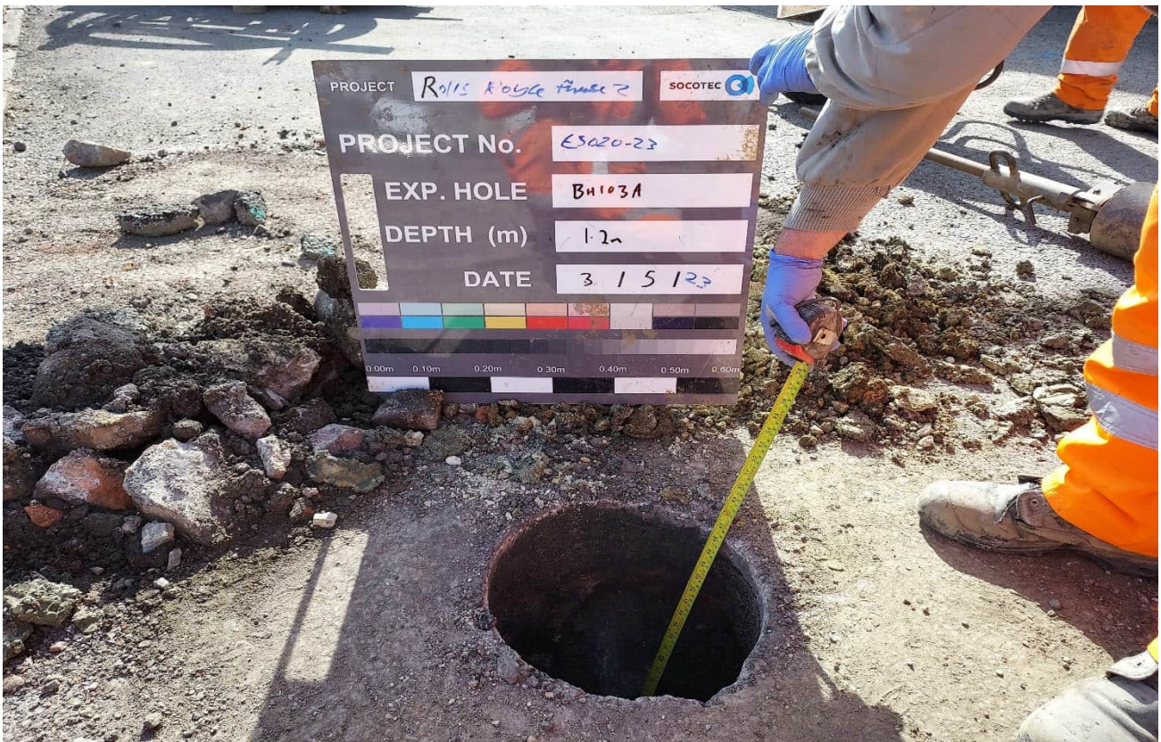
BH103A Inspection pit_1
