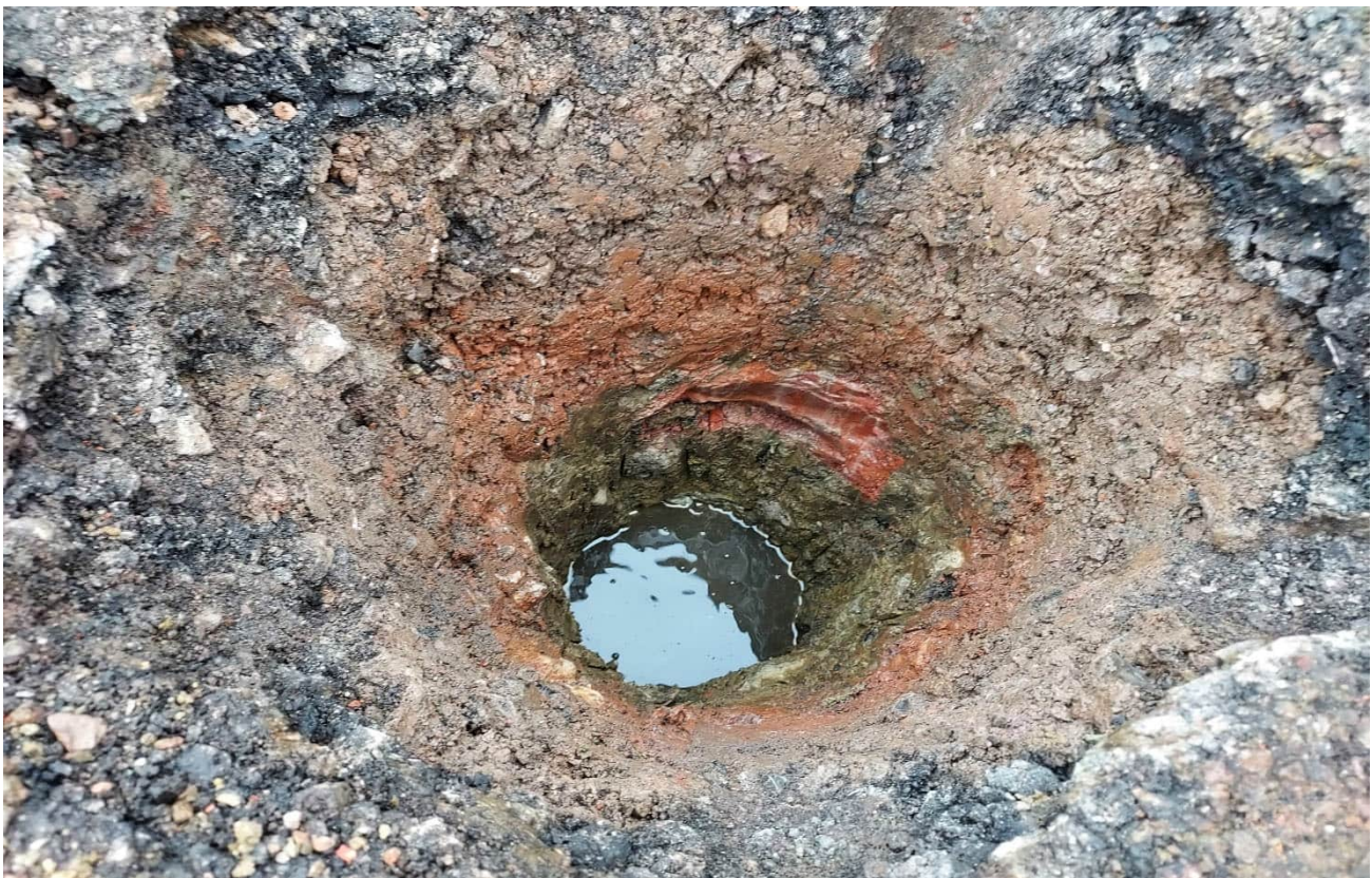
BH102 Inspection pit_2
