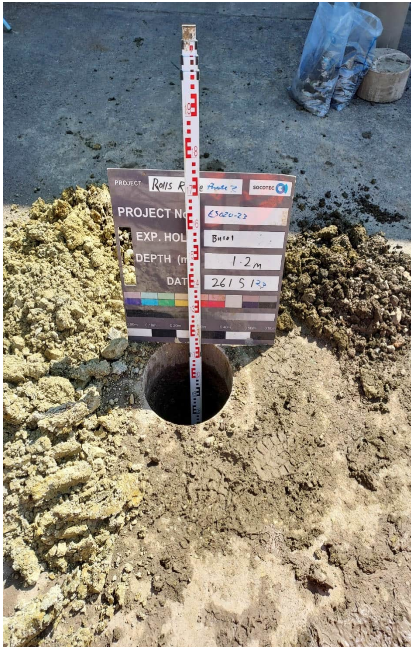
BH101 Inspection pit
