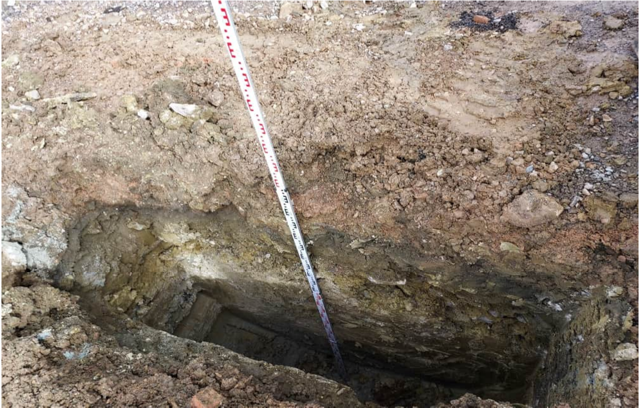
TP104 0.00m to 3.10m Side Wall
