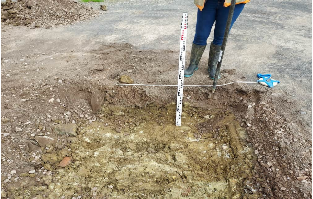
TP105 0.00m to 0.50m Side Wall
