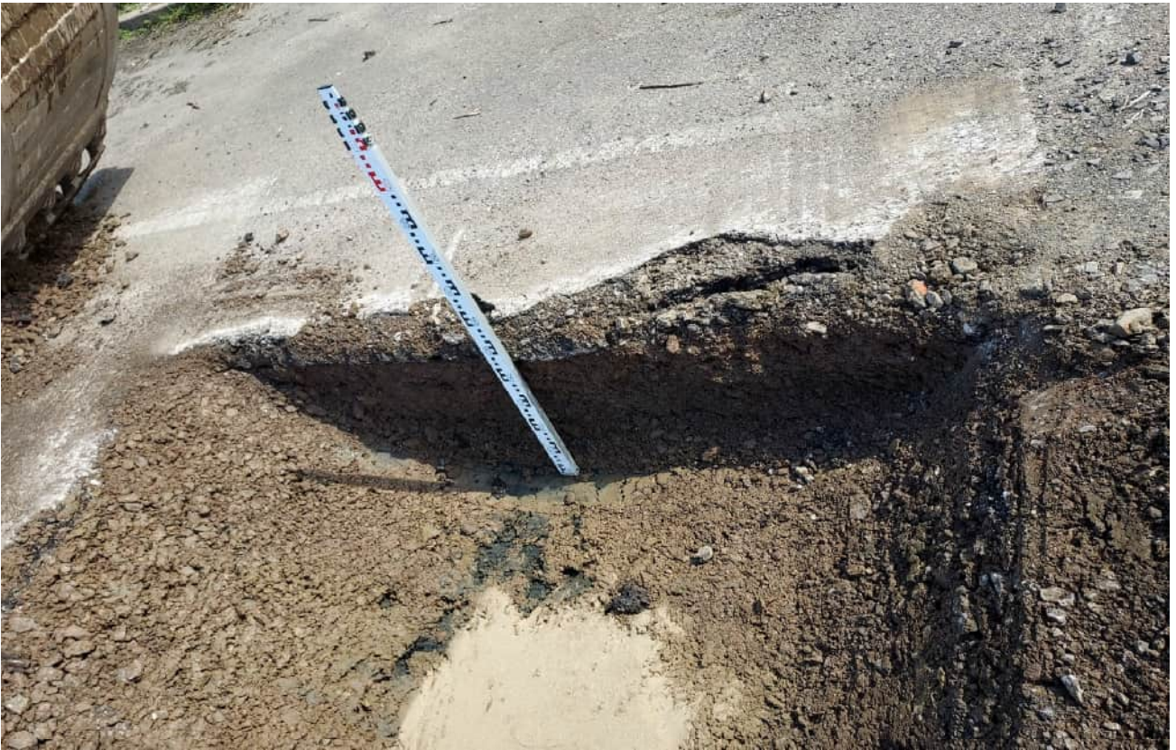
CBR004 Side Wall 0.00m to 0.55m
