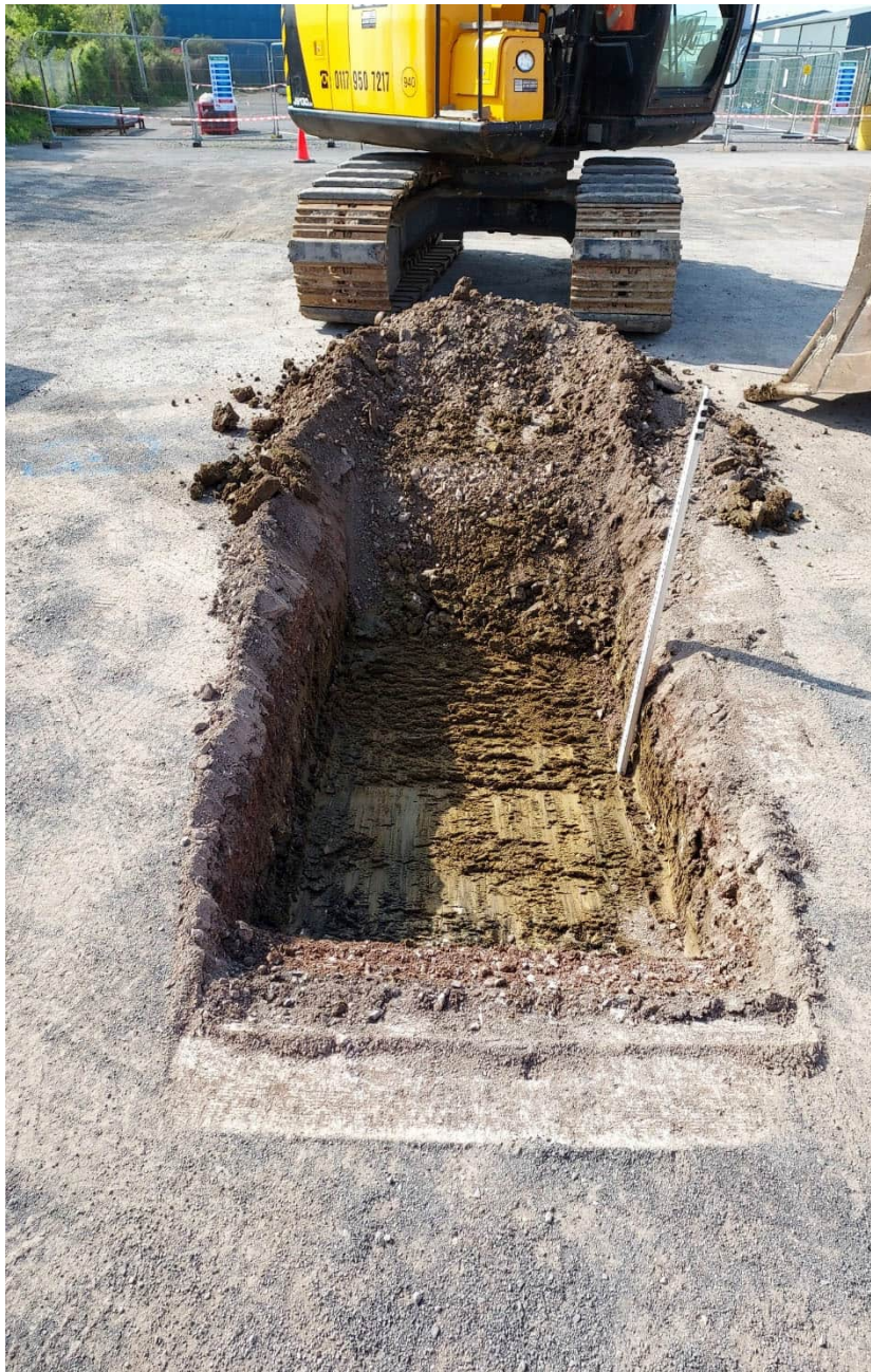
CBR003 0.00m to 0.50m End Wall
