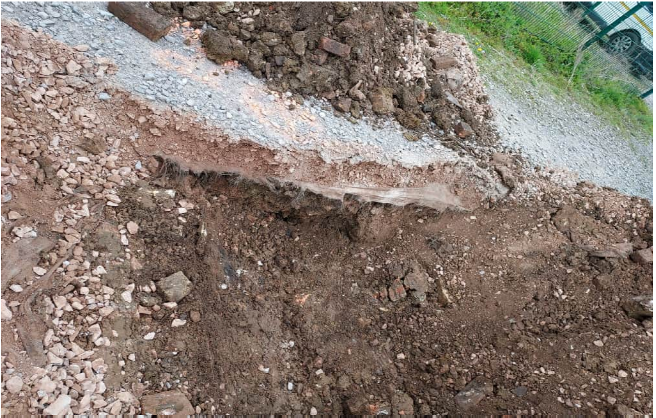
TP101 0.00m to 0.80m Side wall
