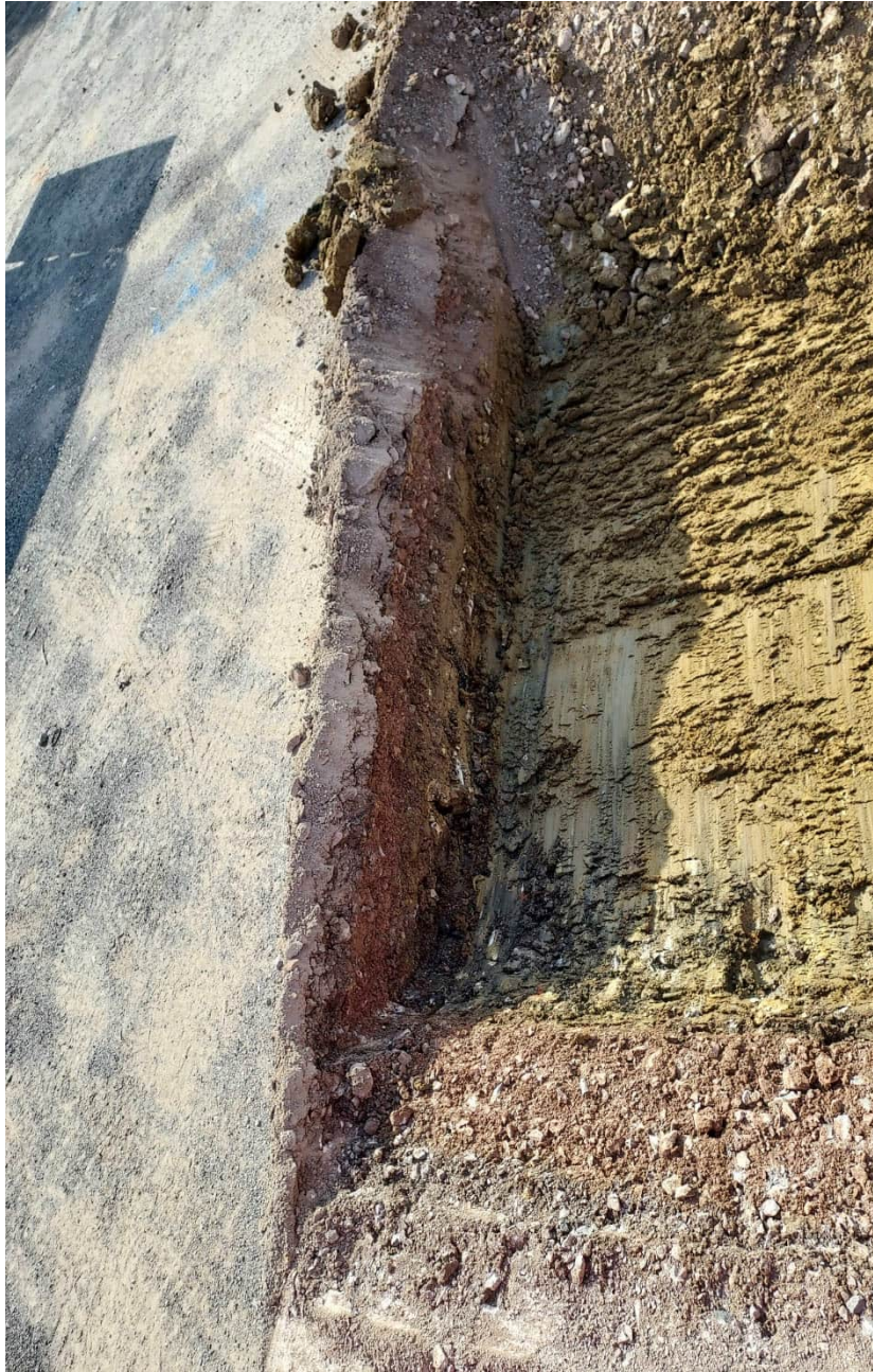
CBR003 0.00m to 0.50m Side Wall 2
