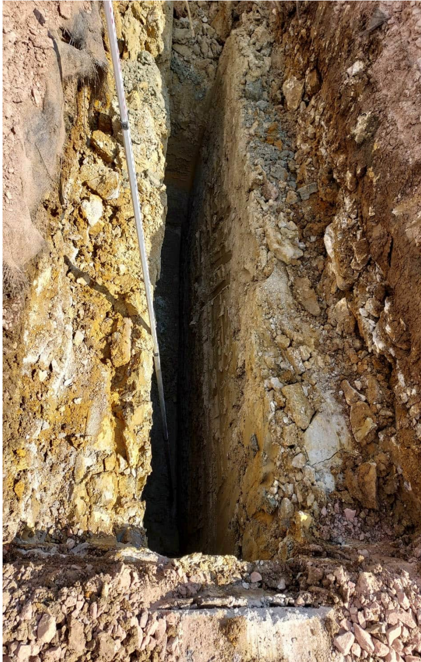
TT101 0.00m to 3.30m Side Wall 2
