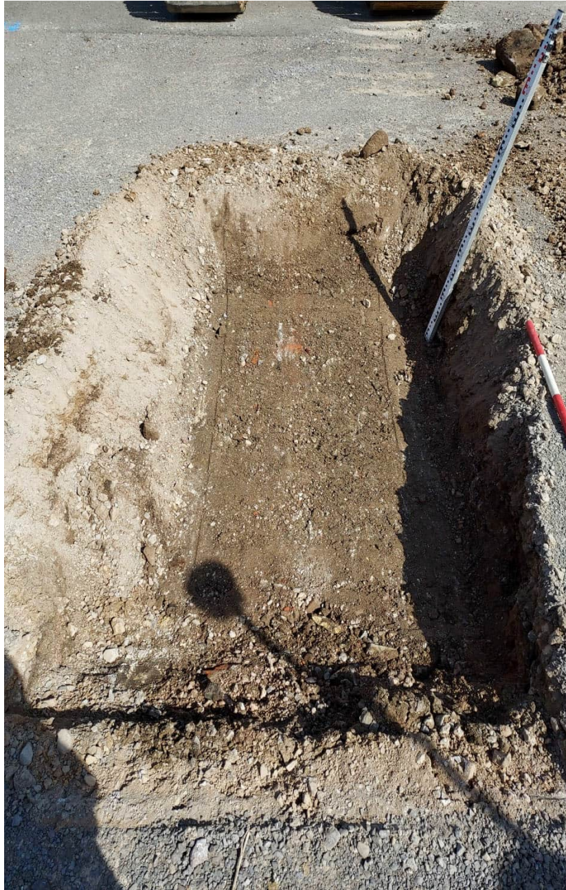
CBR001 0.00m to 0.50m End Wall
