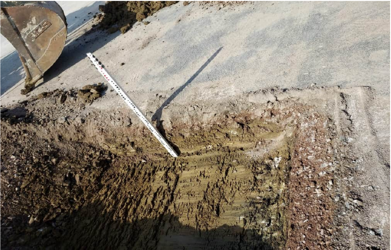
CBR003 0.00m to 0.50m Side Wall 1
