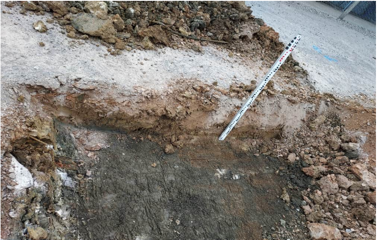
TP104 0.00m to 0.45m Side Wall
