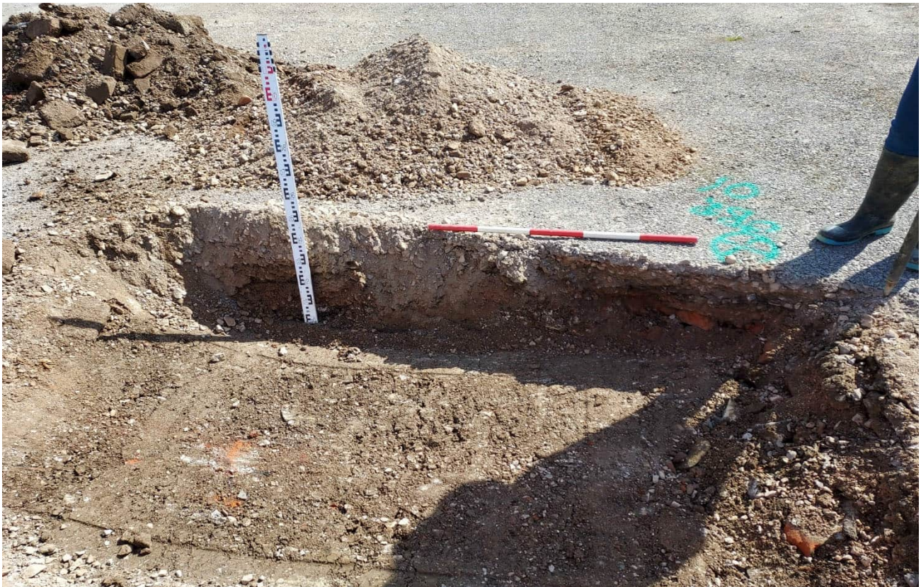
CBR001 0.00m to 0.50m Side Wall 2
