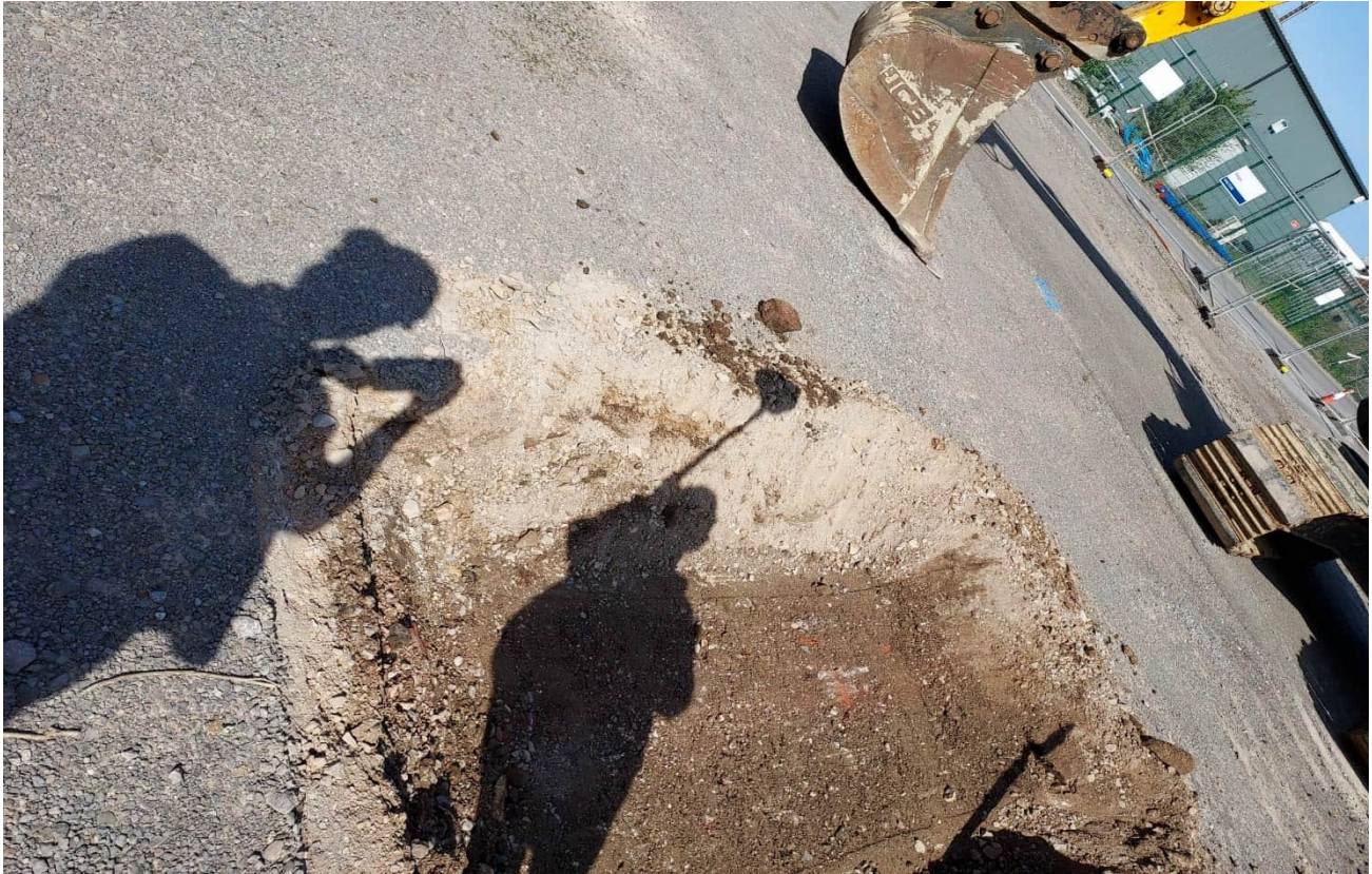
CBR001 0.00m to 0.50m Side Wall 1
