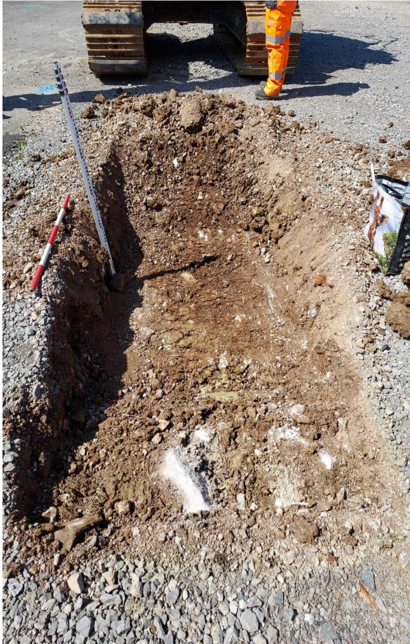
CBR002 0.00m to 0.50m End Wall
