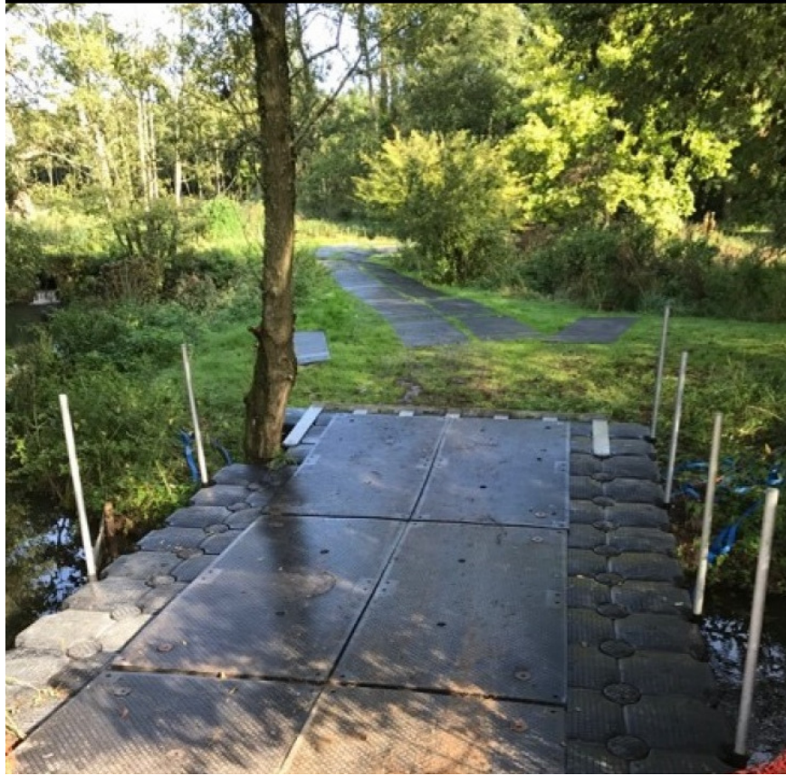
Fig. 2 Ground Guards – MultiMatts Euro Trak is ideal for the ground protection required here.
