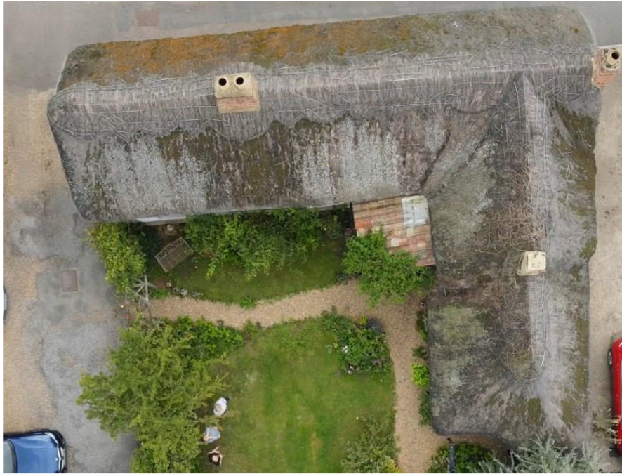
Figure 47 View of roof in 2021, from owner
