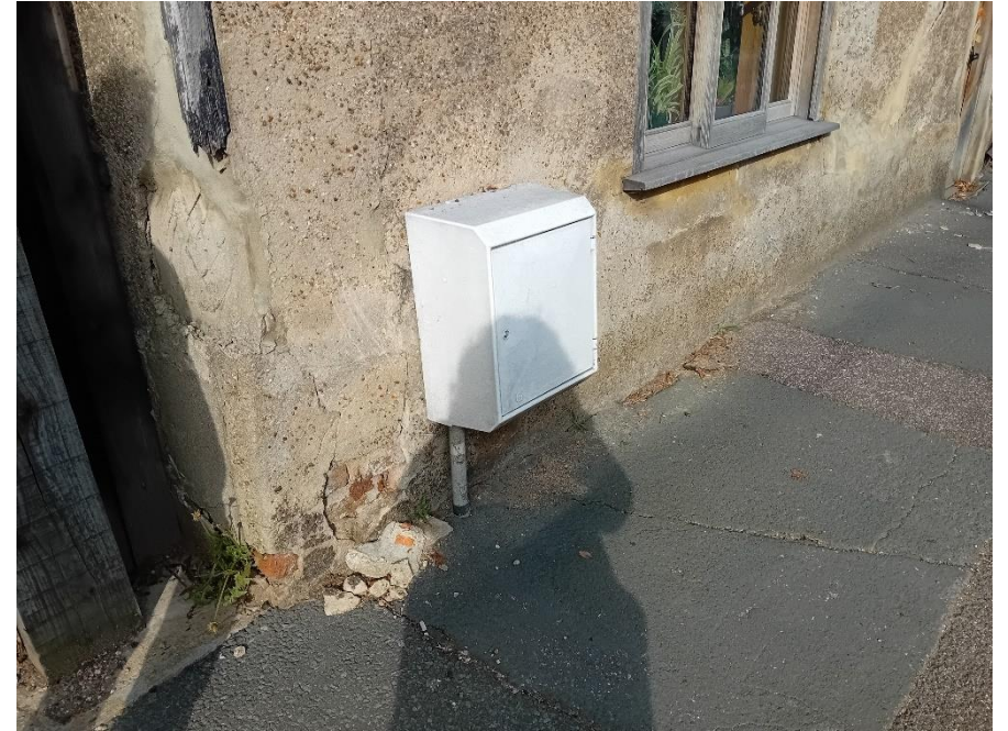
Figure 42 Image at corner of building at pavement, WHC
