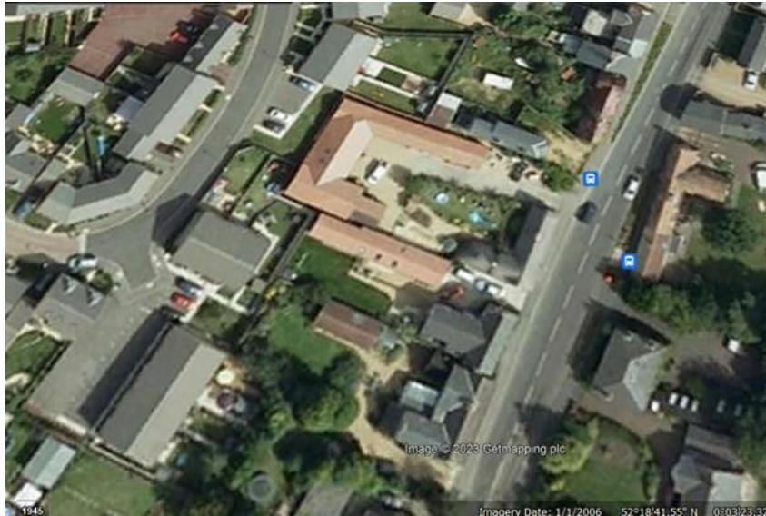
Figure 13 2006 aerial from Google Earth
