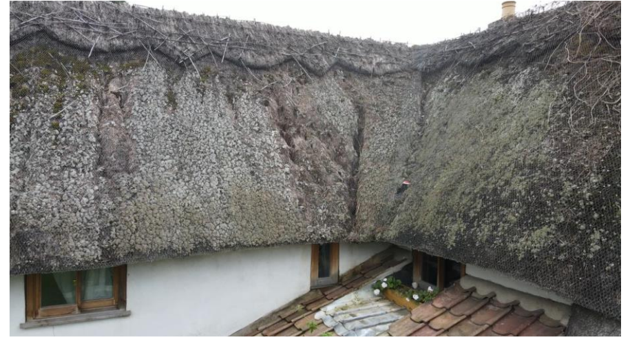
Figure 48 Image of roof at junction, from owner
