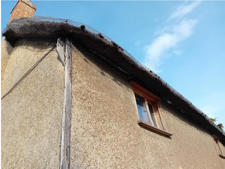
Figure 41 Image of corner timber bead, WHC
