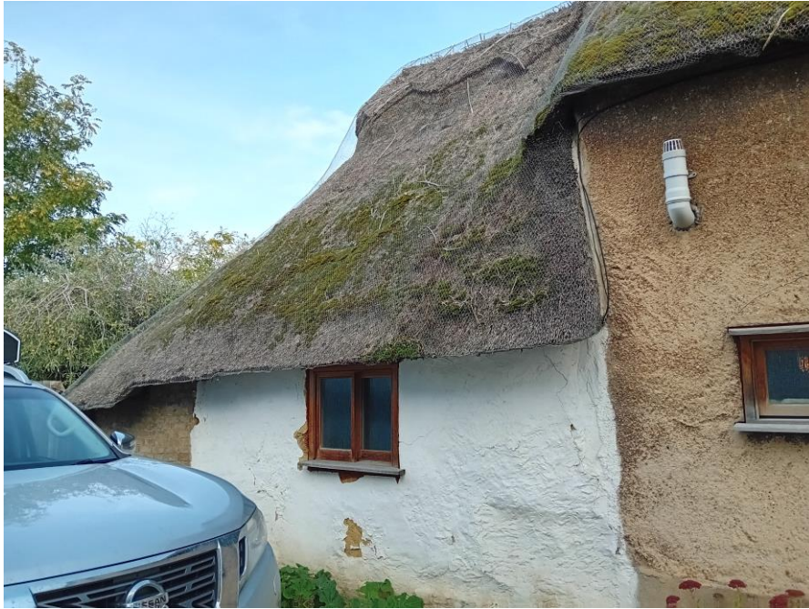
Figure 27 View on south elevation in neighbour's drive, WHC
