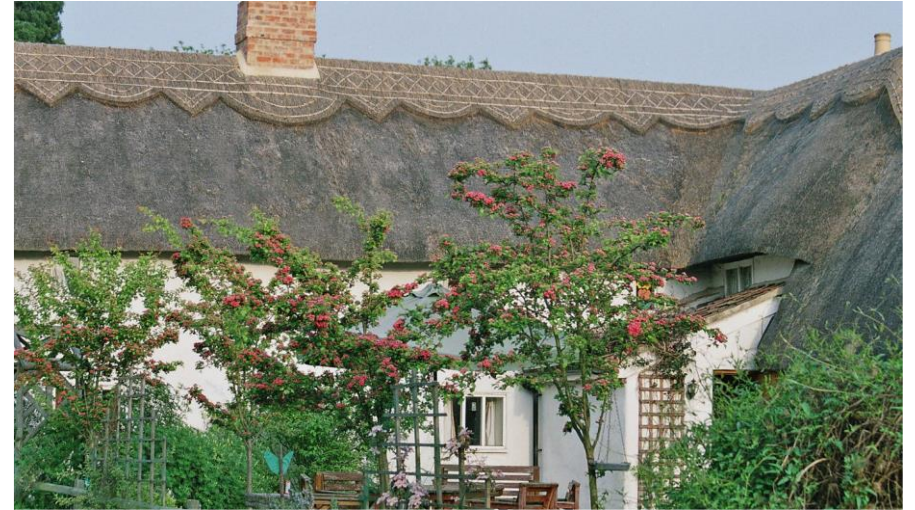
Figure 46 Re-ridge of thatch in 2007, from owner
