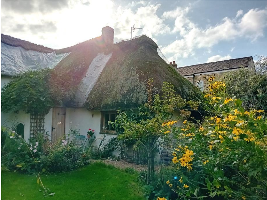
Figure 25 View looking at junction and rear extension, north elevation, WHC
