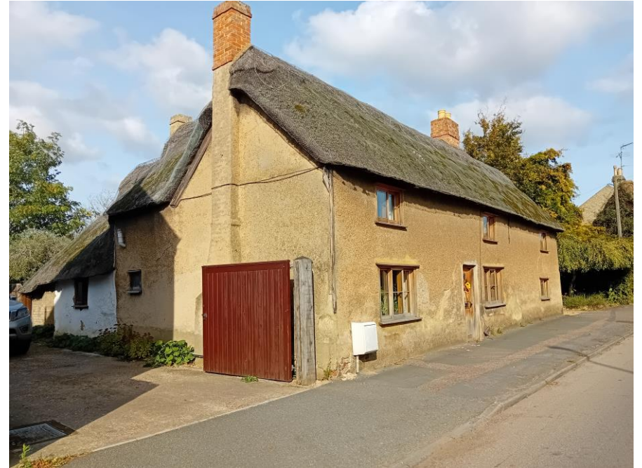
Figure 30 Front east elevation and side south elevation, WHC
