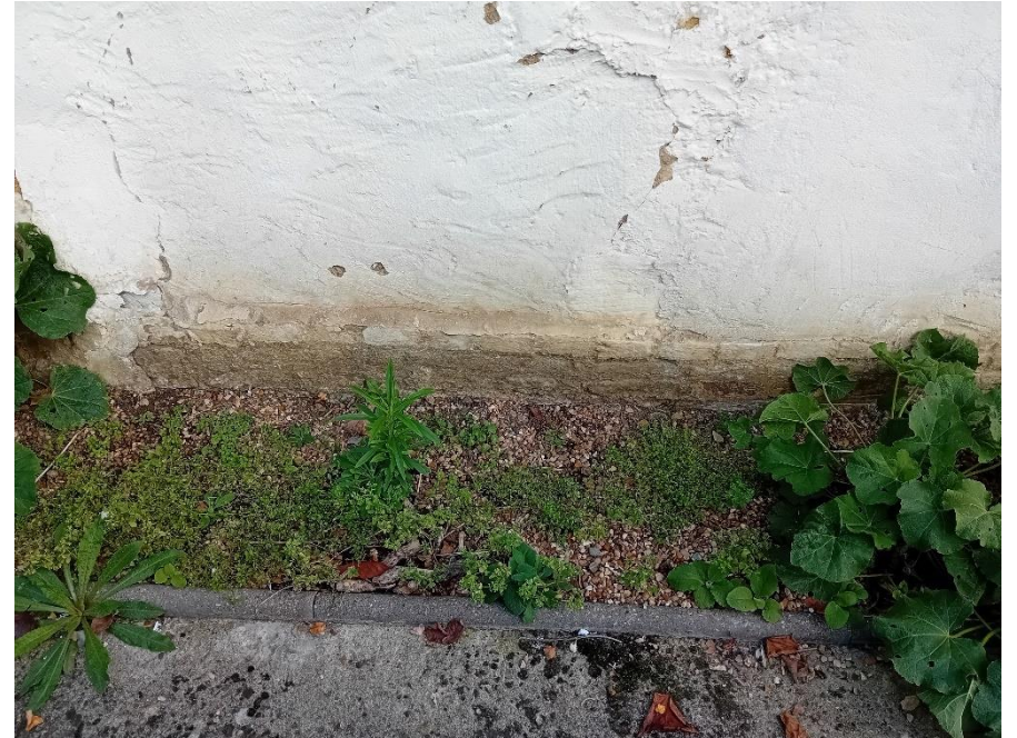
Figure 36 Image of render at base of building, WHC
