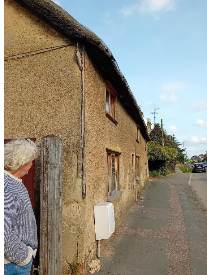
Figure 40 Image of corner timber bead, WHC
