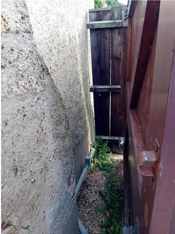
Figure 39 South elevation of building render behind neighbour's gate, WHC
