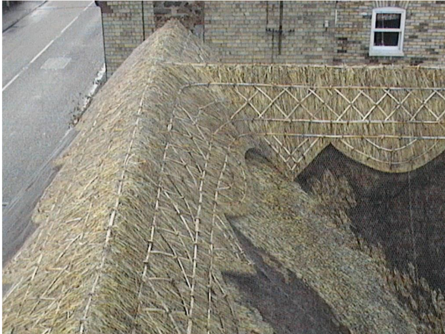
Figure 45 Re-ridge of thatch in 2007, from owner
