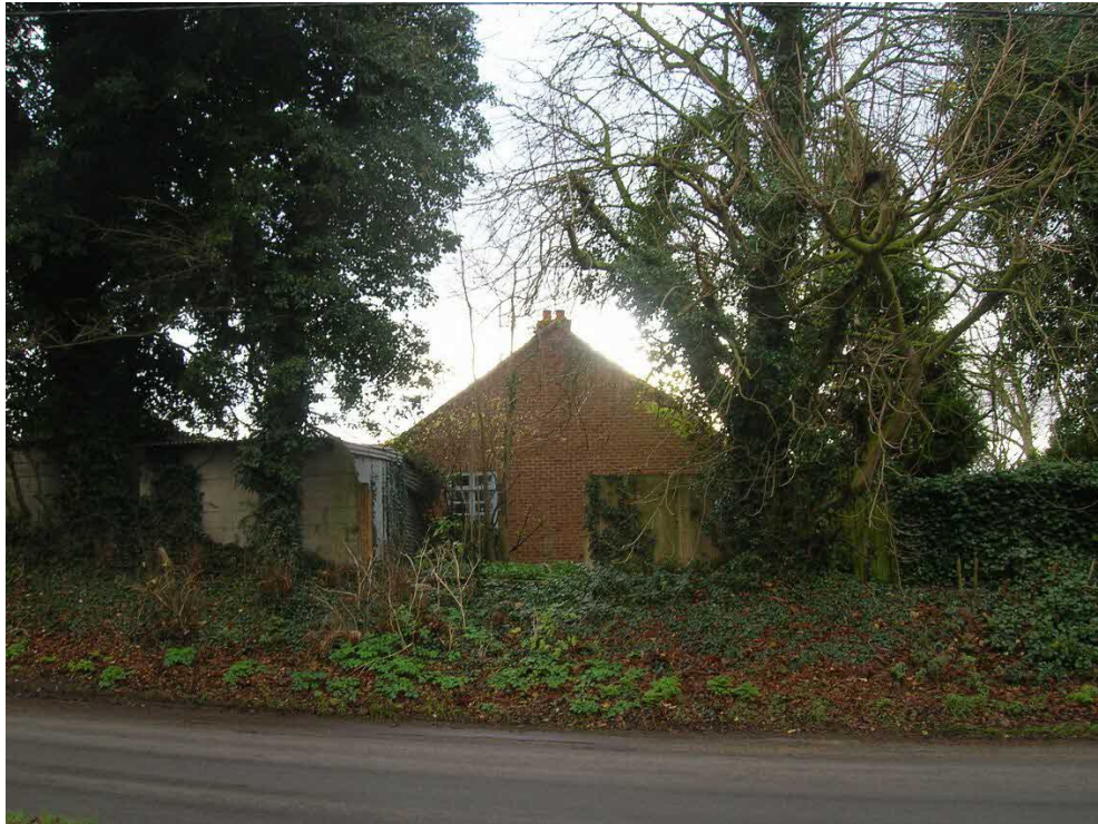
5. North Elevation From Holt Road
