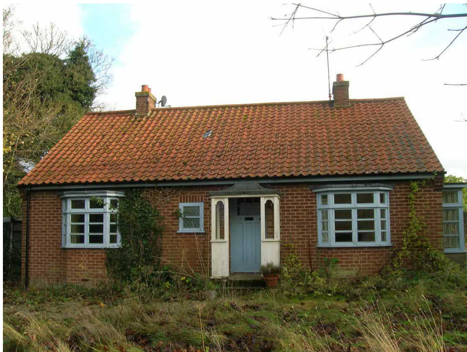
1 West Elevation (showing Front Porch)
