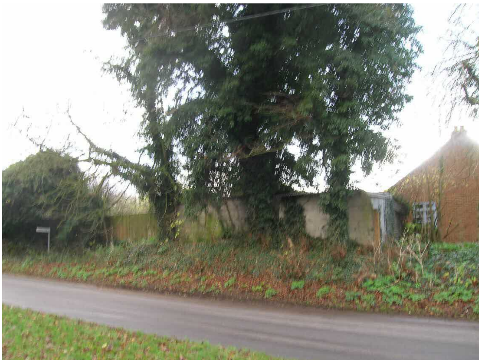
6. North Elevation with outbuildings – from Holt Road
