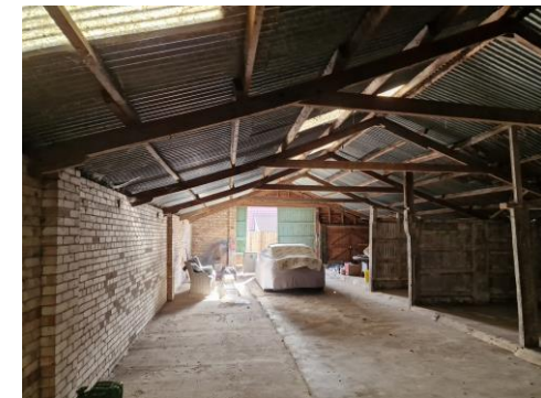
Photograph 4: Internal view of larger outbuilding
