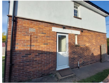
Side elevation of the property
