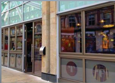
Finished in anodised Bronze with metallic RAL beading with satin nickel hardware.
