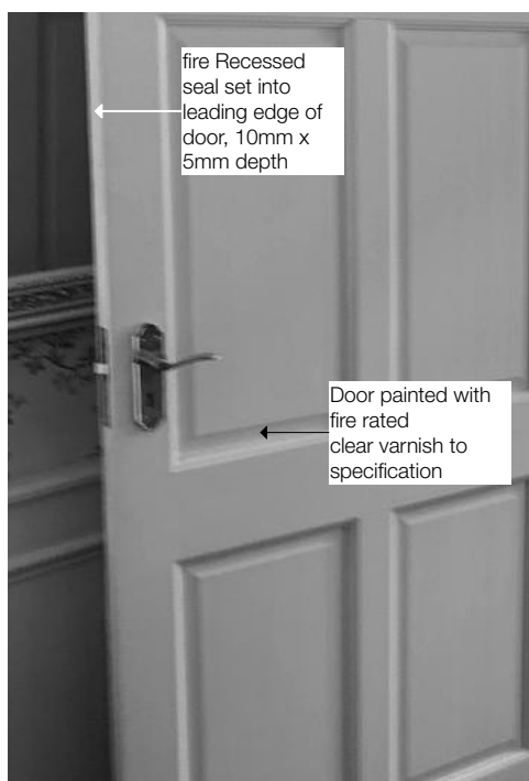
Illustration showing proposed fire seal installation
