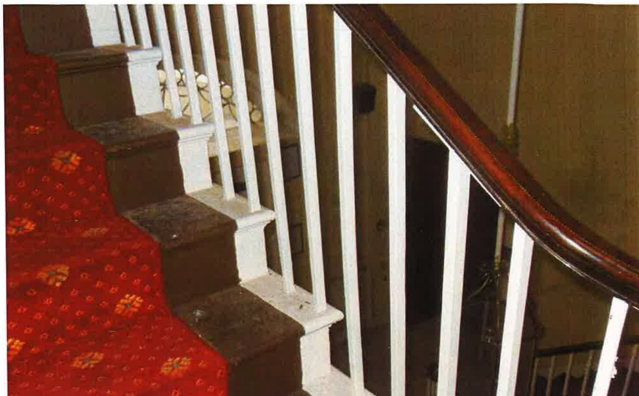
Appendix 4.33: Balustrade, handrail and treads of the 1820s staircase
