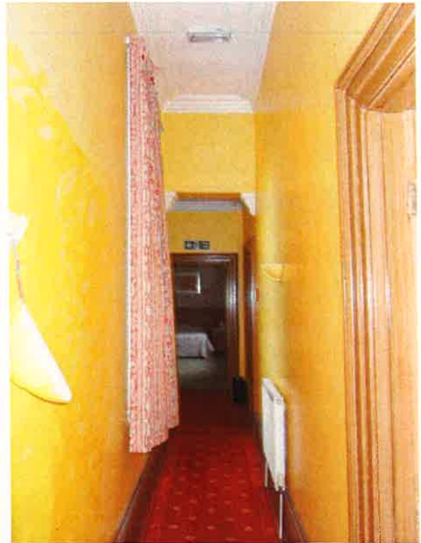
Appendix 4.40: Late 19th century corridor to be removed to open the courtyard
