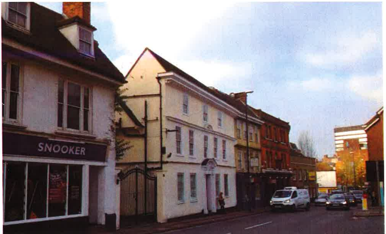
Appendix 4.2: Front elevation of the structure viewed from the south showing evidence of the development of the building to the south side elevation
