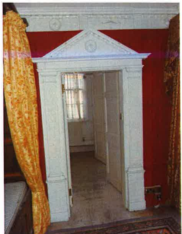
Appendix 4.18: Matching right hand side door providing access into toilet
