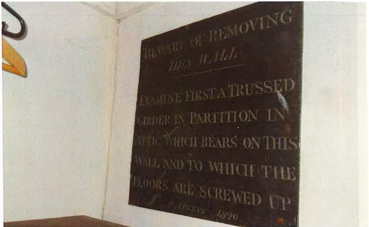
Appendix 4.19: 1820s plaque by architect T. Atkins located within first floor cupboard
