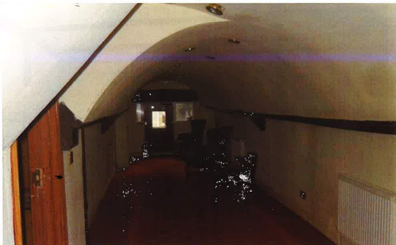
Appendix 4.22: Barrel arched hallway at second floor within front portion of the building
