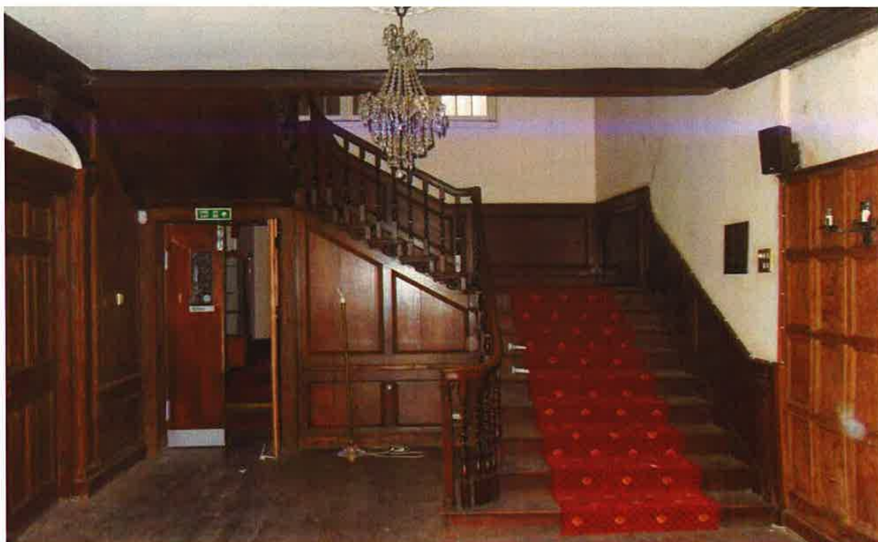
Appendix 4.8: 18th century staircase
