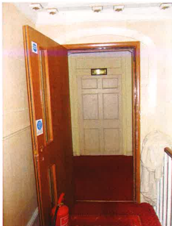
Appendix 4.28: Existing sealed door to be reopened to provide access to Unit 14
