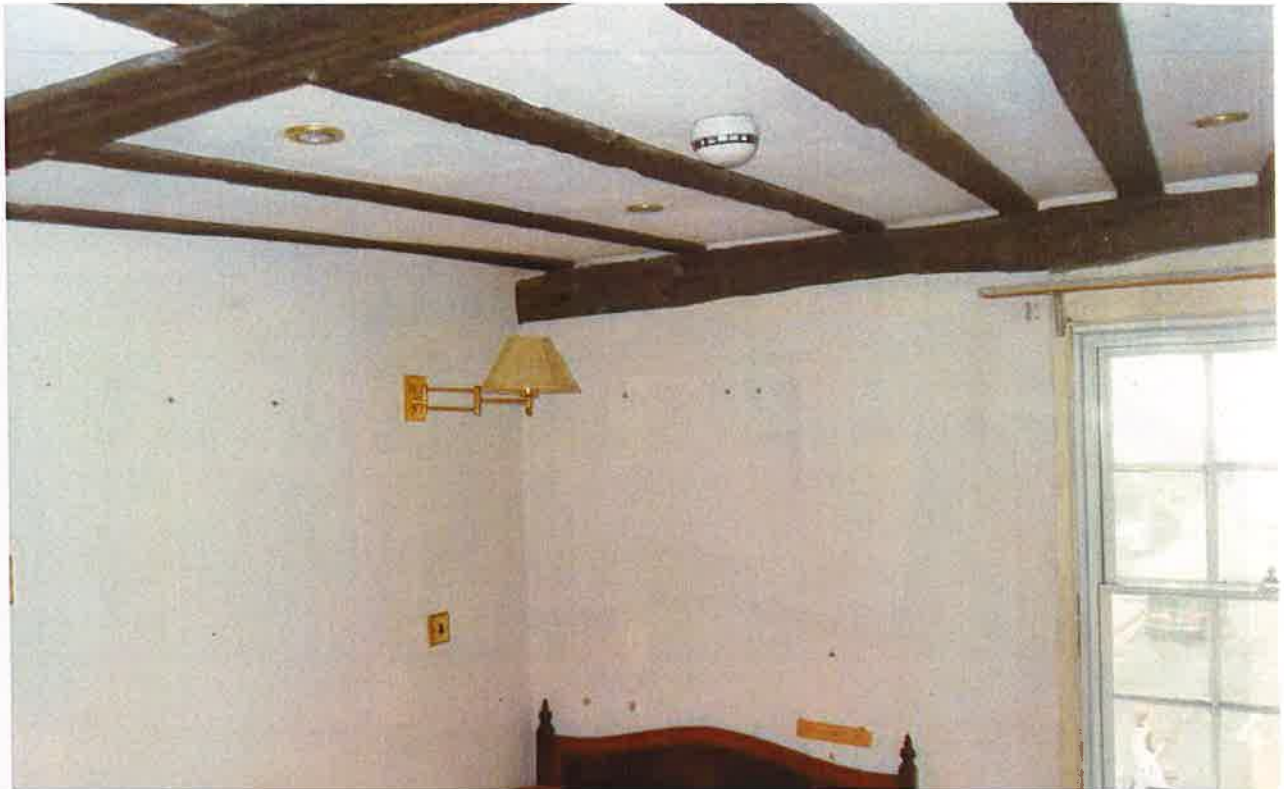
Appendix 4.23: Second floor bedroom with exposed timber beams
