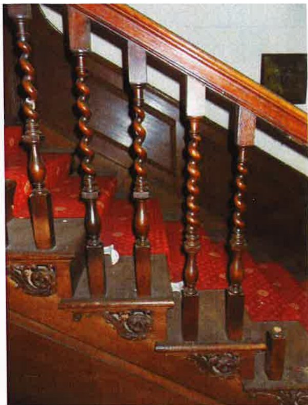
Appendix 4.9: Turned balustrade of 18th century staircase
