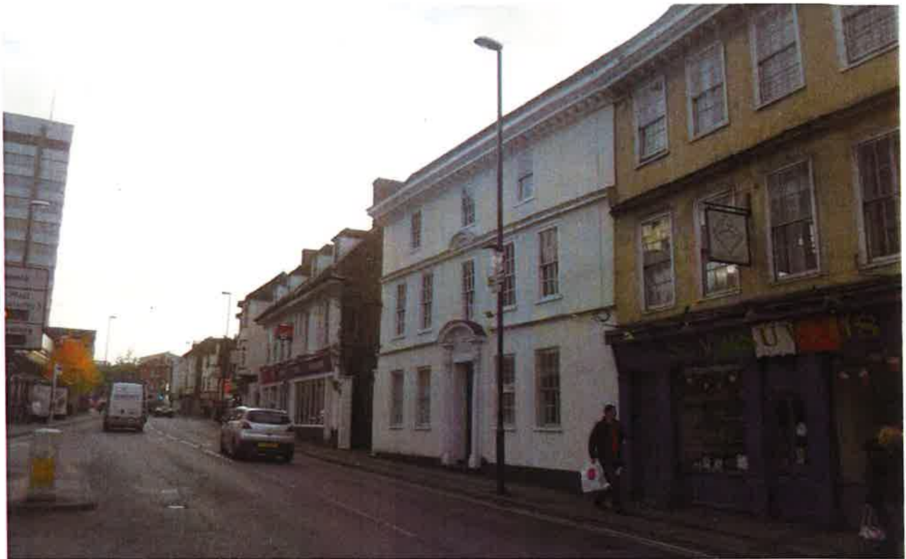
Appendix 4.1: Front elevation of Stone Court Hotel viewed from the north
