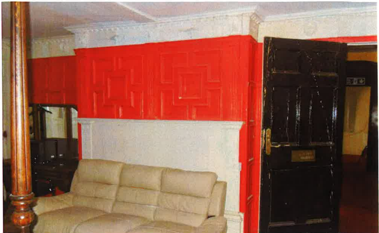
Appendix 4.16: Southern most panelled room at first floor with blockedup fireplace
