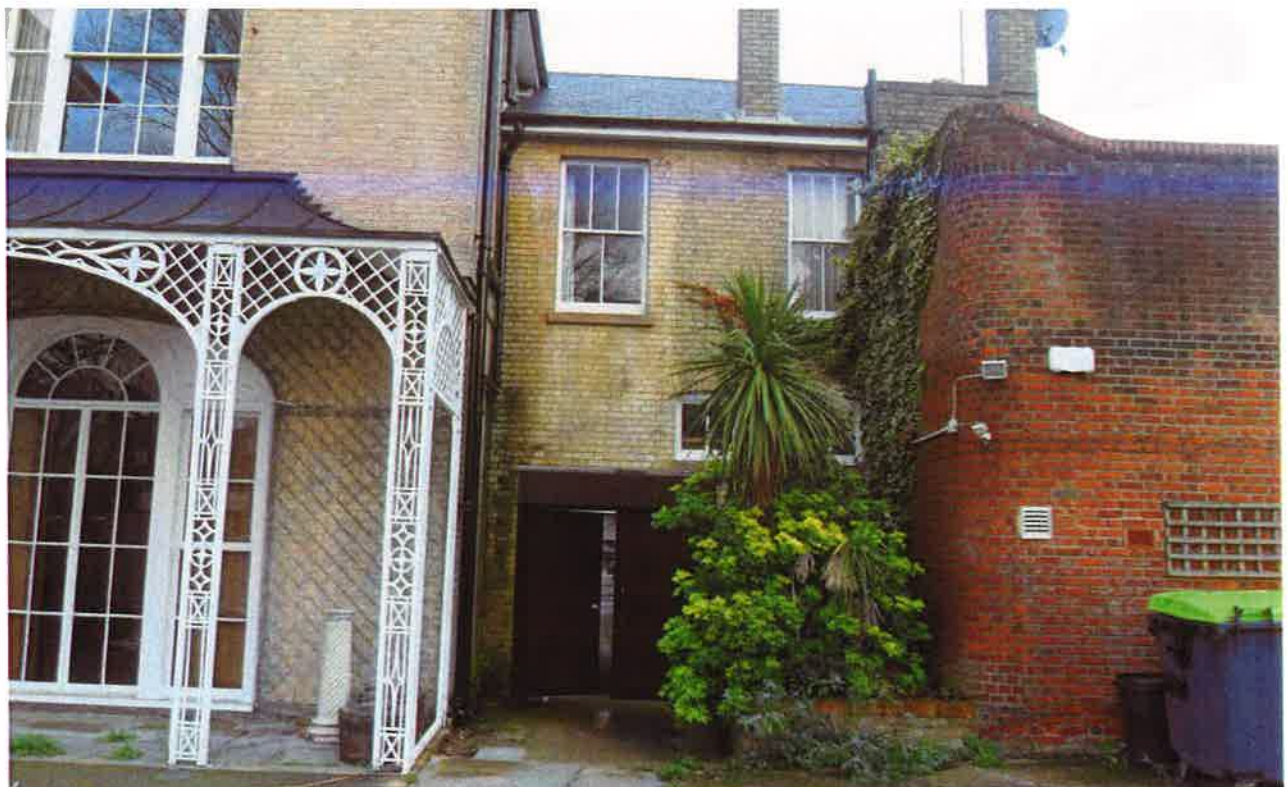
Appendix 4.4: Rear elevation of with the flying freehold and boiler room
