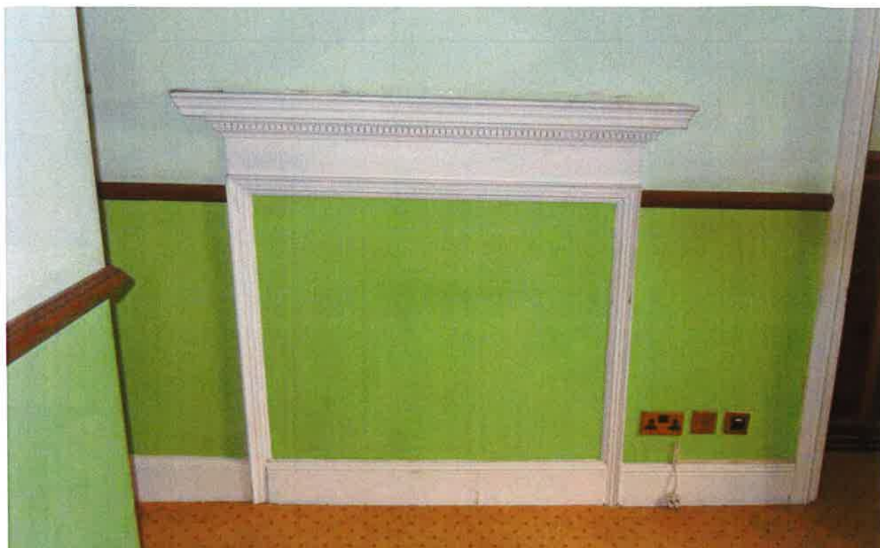
Appendix 4.21: First floor rear room (within front portion of building) with blocked up fireplace
