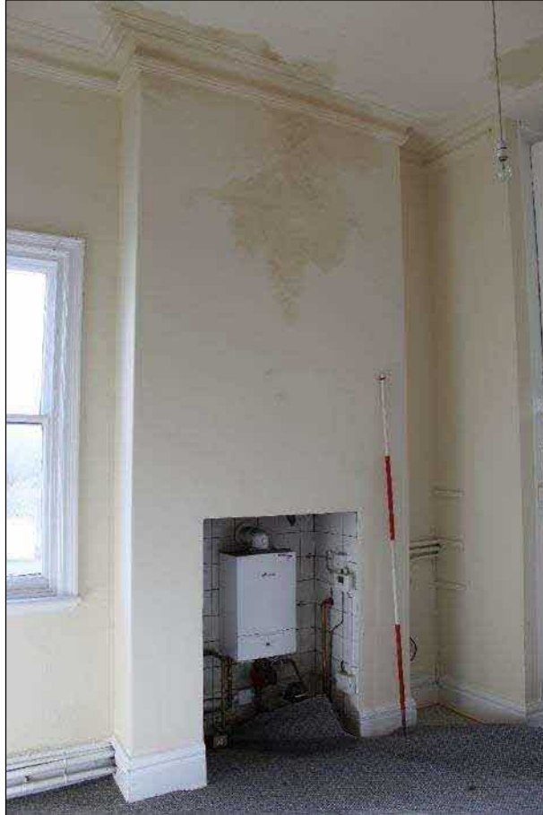
Plate 47 (shot 52): Modified fireplace in Bedroom 1.9. Looking east-northeast, 2m scale
