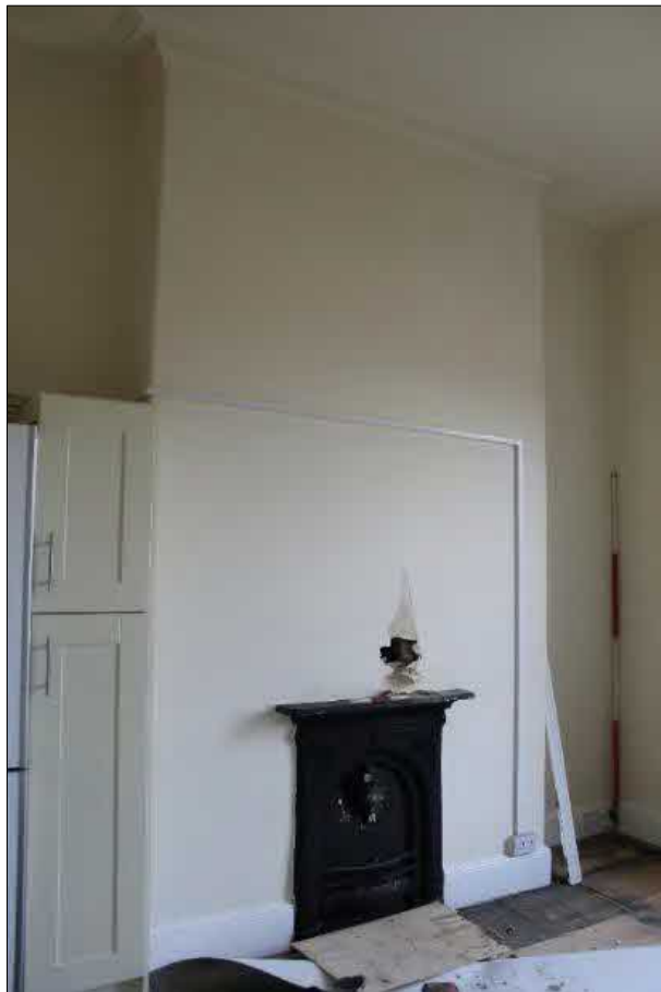
Plate 41 (shot 81): Retained fireplace along the southwest wall in room 1.5. Looking west-northwest, 2m scale
