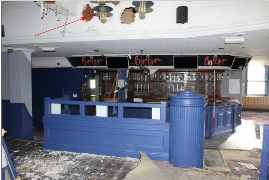
Plate 23 (shot 113): View from Lounge 1, arrow points to possible closed string of a former staircase. Looking southeast, 2m scale
