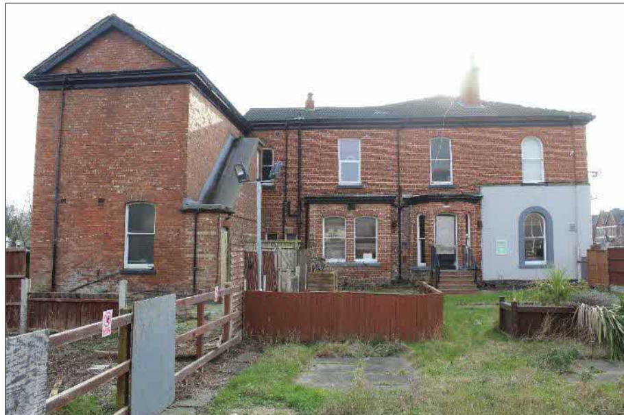
Plate 6 (shot 22): General view of the northwest elevations and yard area. Looking southeast
