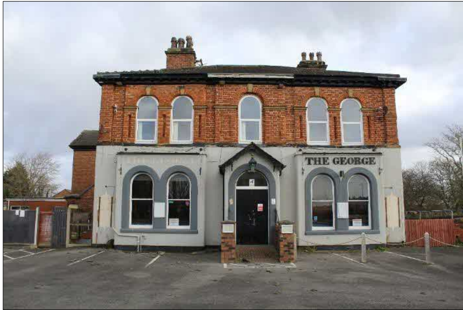
Plate 2 (shot 2): View of five-bayed front elevation. Looking northeast, 2m scale
