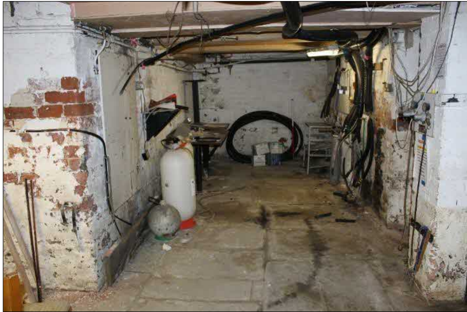
Plate 12 (shot 153): General view of cell A0.3. Looking southeast, 1m scale
