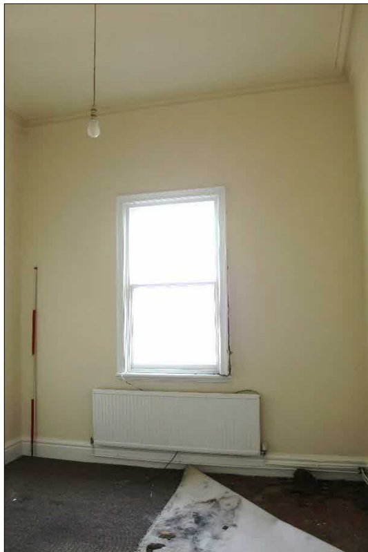
Plate 49 (shot 43): General view of Bedroom 1.11. Looking northeast, 2m scale
