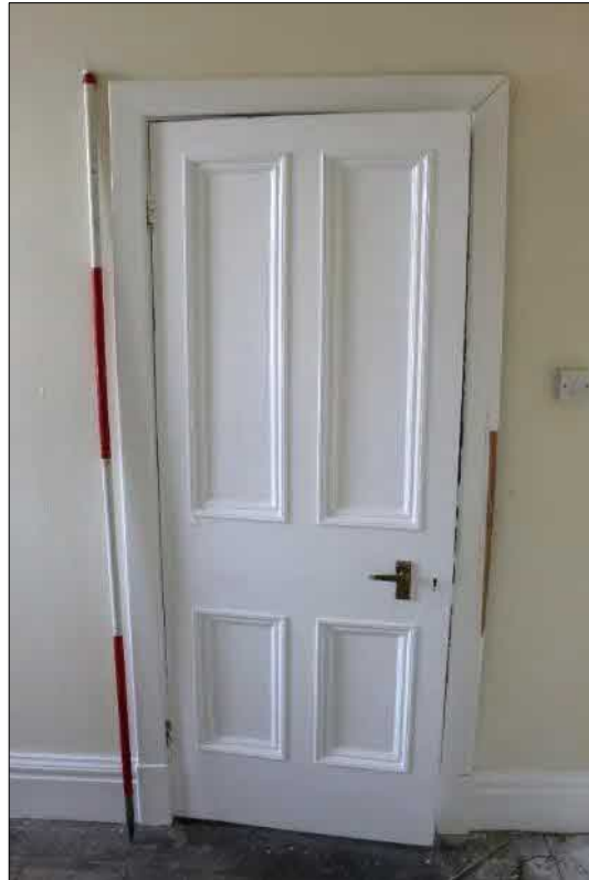
Plate 48 (shot 48): Representative shot of door (in Bedroom 1.10). Looking southeast, 2m scale
