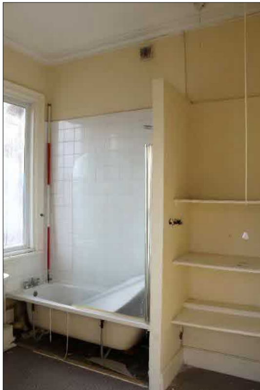
Plate 46 (shot 59): General view of bathroom 1.8, in the annex B. Looking south-southwest, 2m scale
