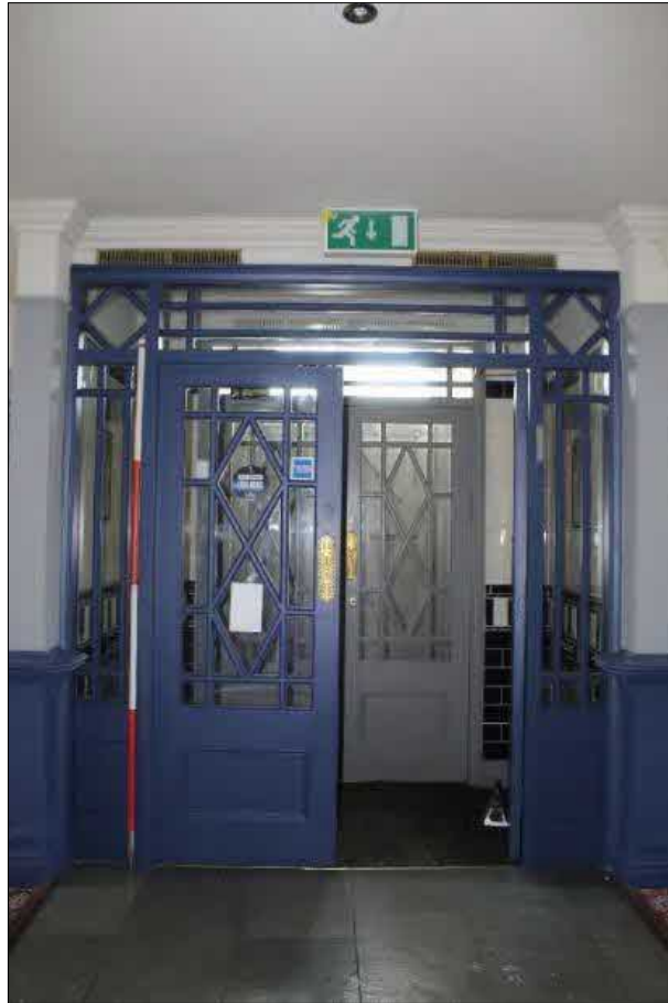
Plate 19 (shot 121): Main entrance from Duke Street. Looking southwest, 2m scale
