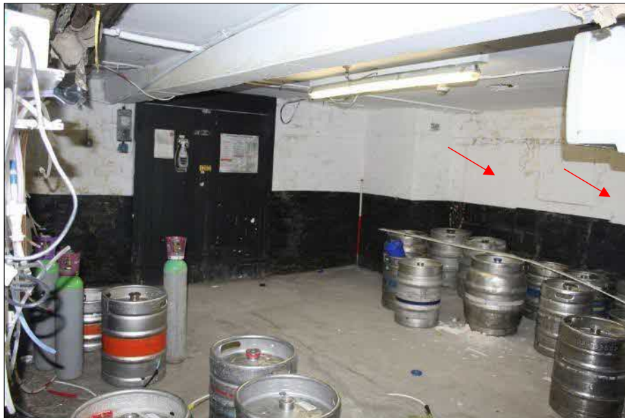
Plate 11 (shot 156): General view of A0.2 with bricked up openings on the southwest wall, see arrows. Looking southwest
