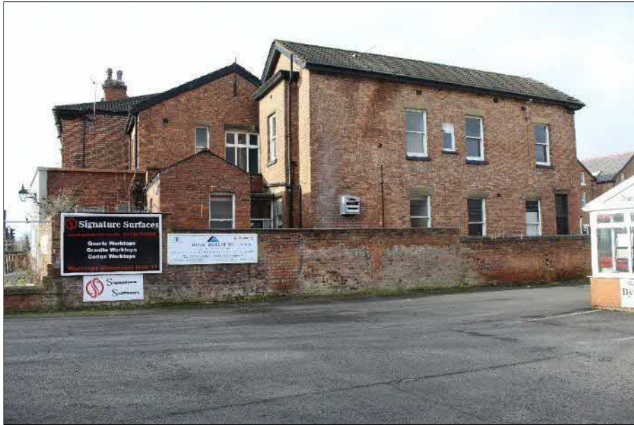
Plate 5 (shot 17): General view of the northeast elevations. Looking west-southwest
