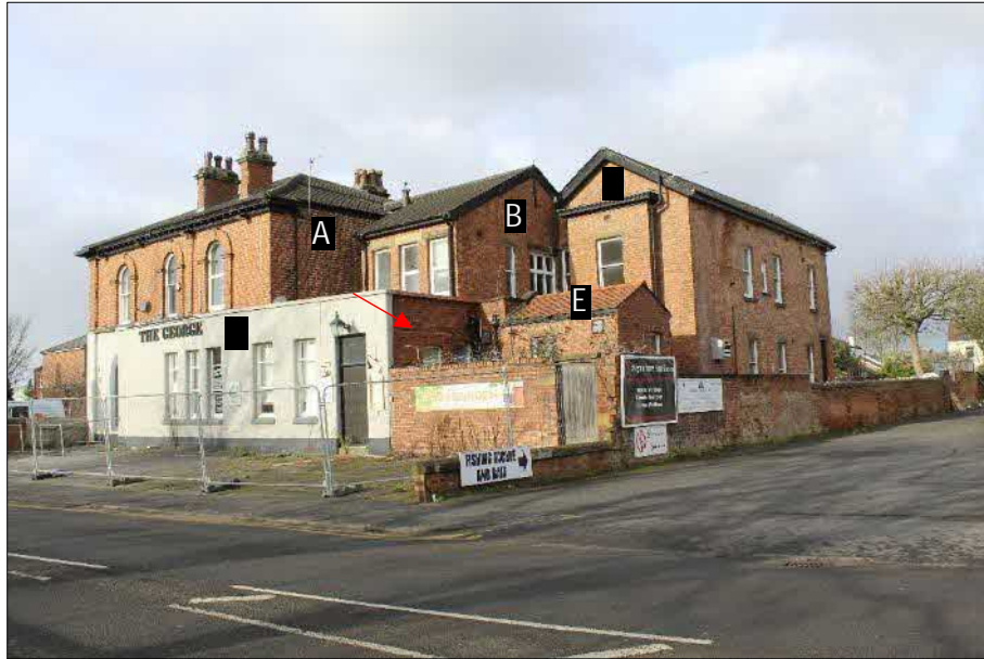
Plate 1 (shot 16): General view of the George Hotel, showing its various extensions. Arrow points to raised roof or incorporating earlier structure into a new extension. Looking west-northwest
