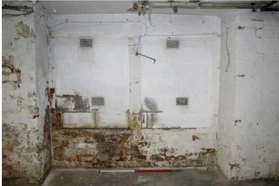
Plate 16 (shot 146): Blocked openings on the southeast wall. Looking southeast, 1m scale
