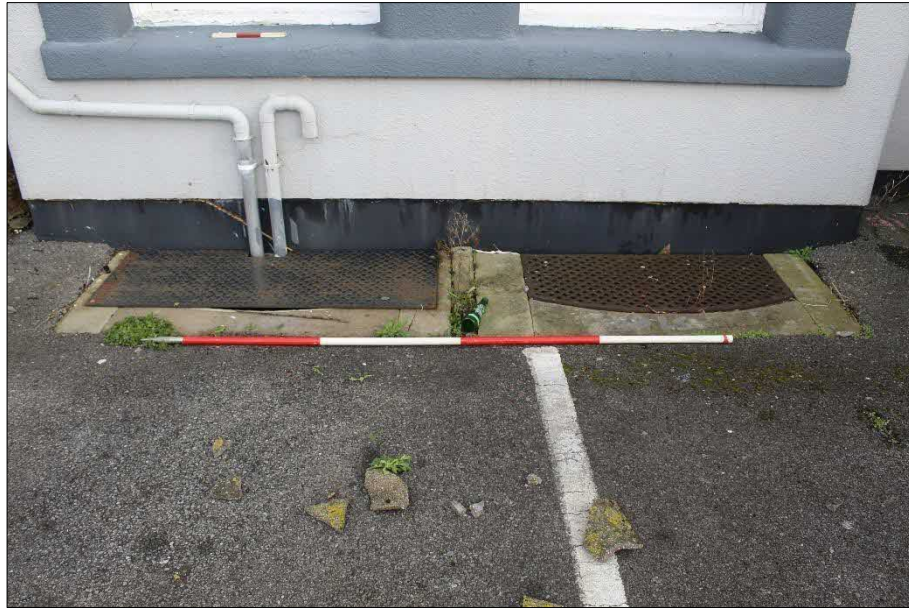
Plate 4 (shot 3): Capped off cellar lights. Looking northeast, 2m scale
