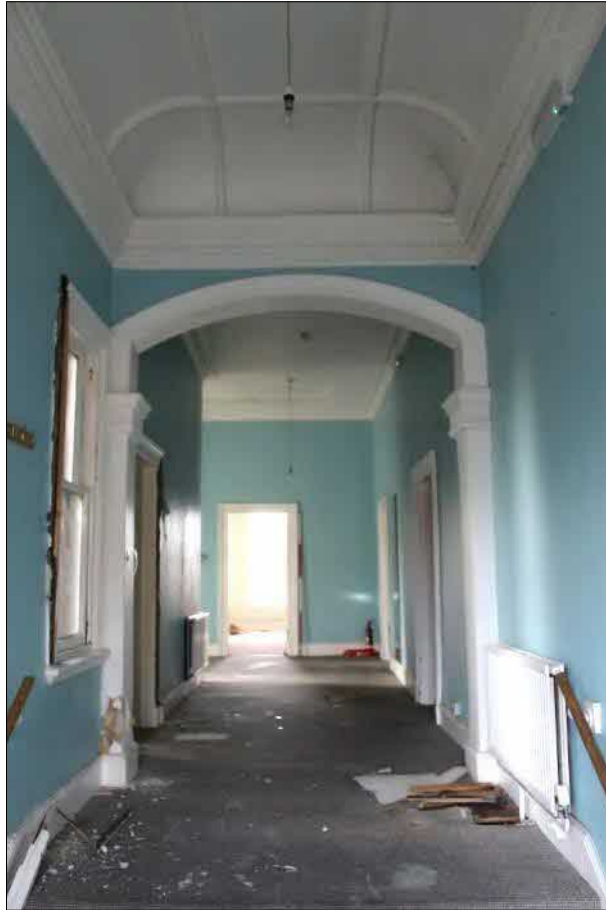
Plate 34 (shot 62): General view of the first floor corridor of the main hotel. Looking southwest, 2m scale
