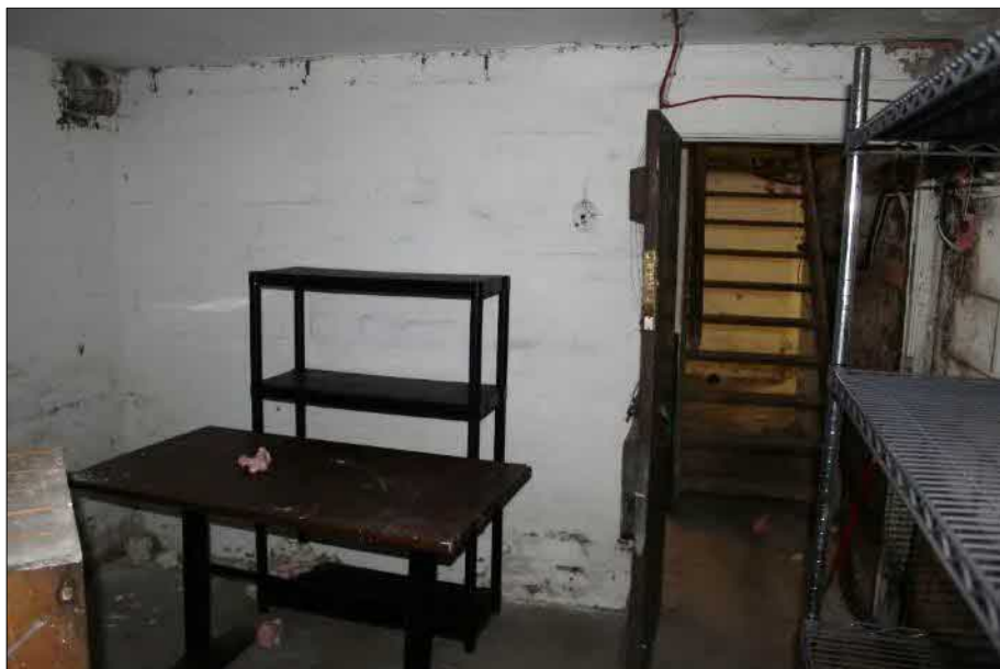
Plate 17 (shot 169): General view of Cell C0.2, looking southeast
