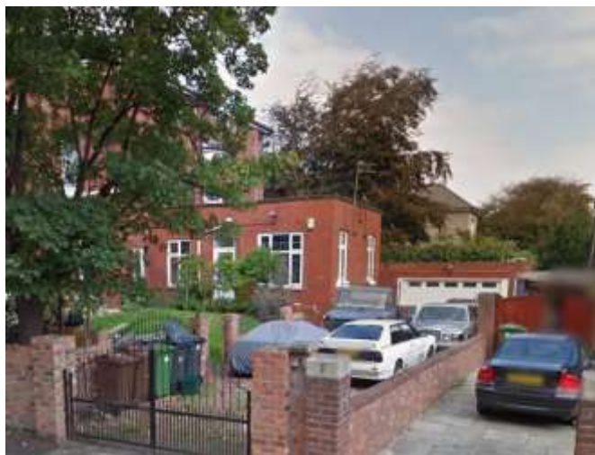
Fig. 3 - Annex that used to occupy No. 1E
