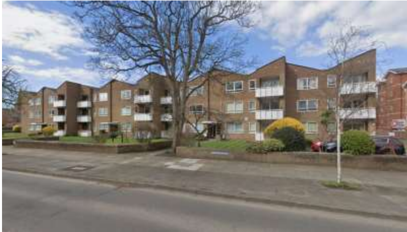
Fig. 4 - Example of post-war flats on Lulworth Road, in close proximity to the site
