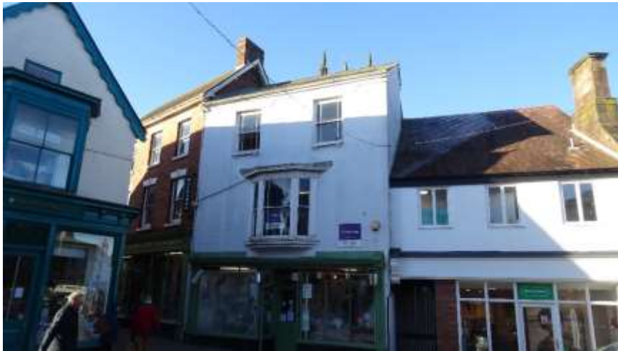
Figure 4.4. Site frontage from east
