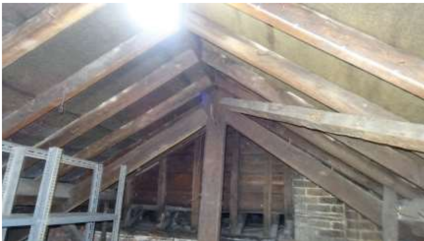
Figure 4.6. Inside parts of rooms open to roof
