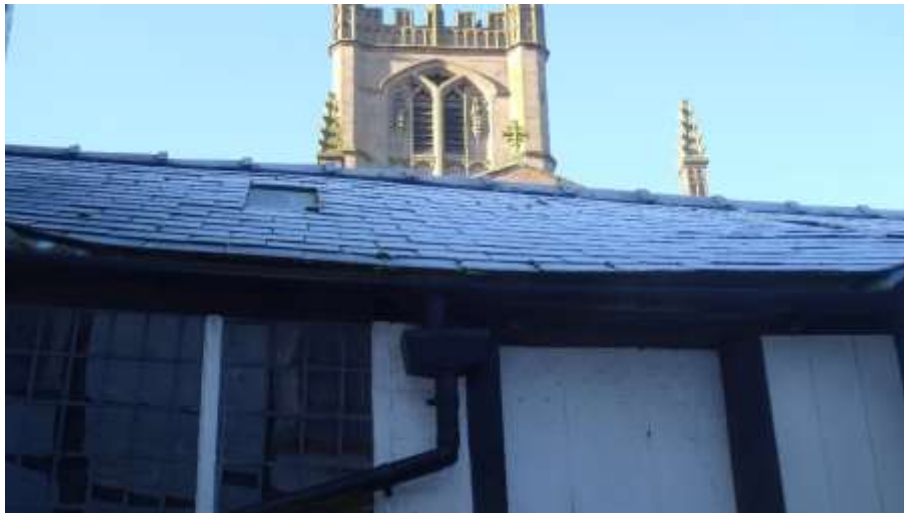
Figure 4.7. Roof seen over western part of building
