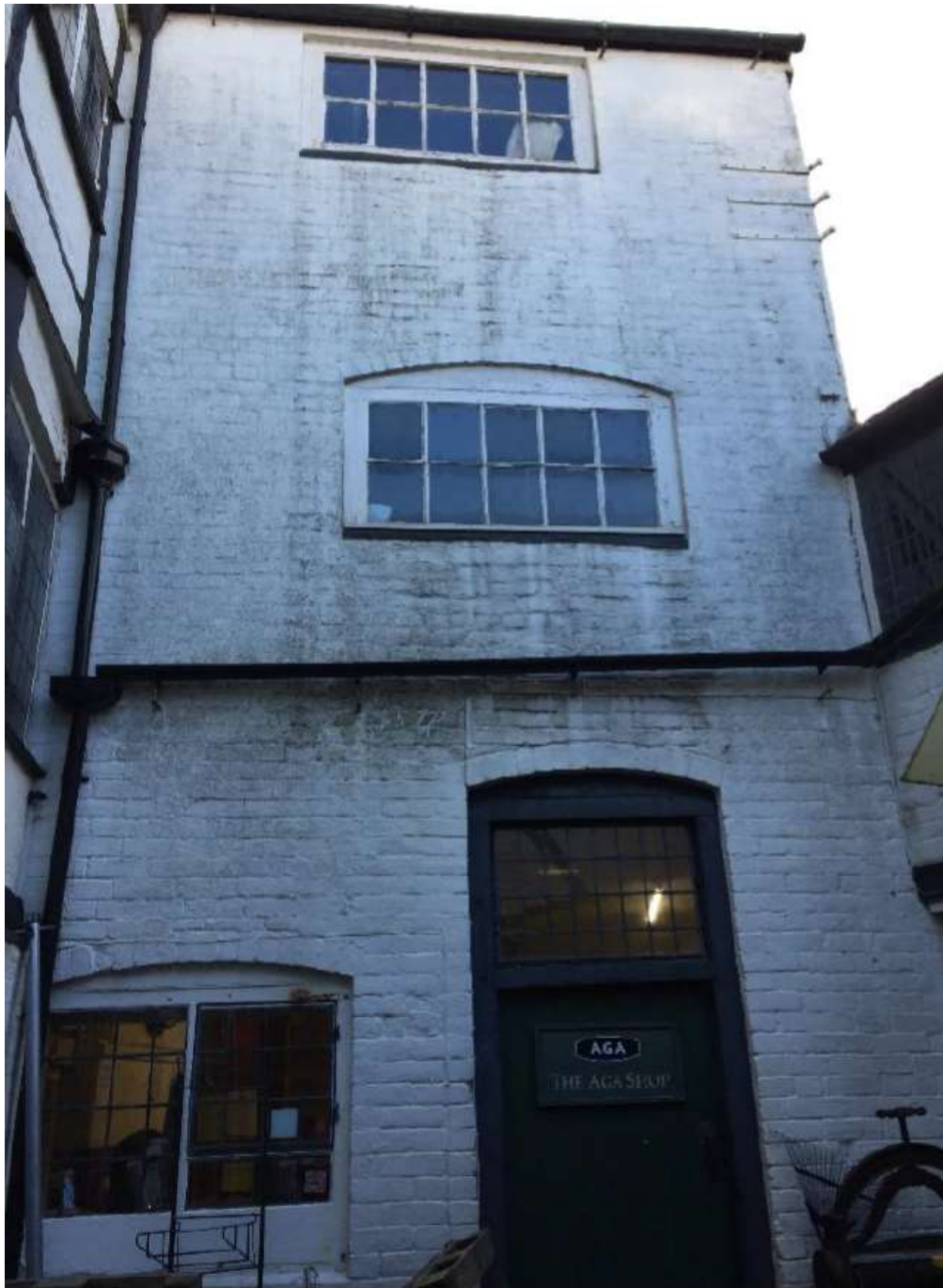
Walls within Courtyard - Photo 6
