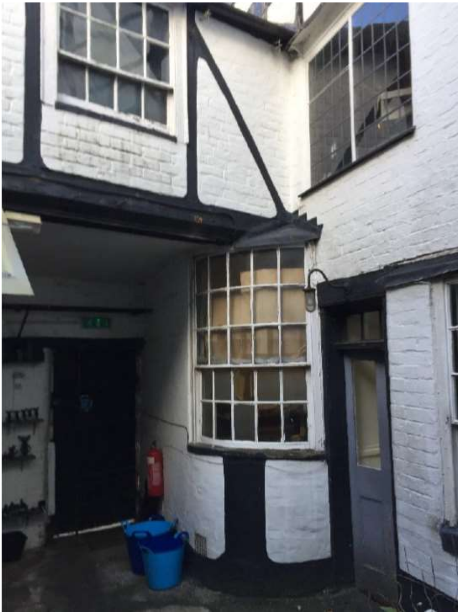
Walls within Courtyard - Photo 9
