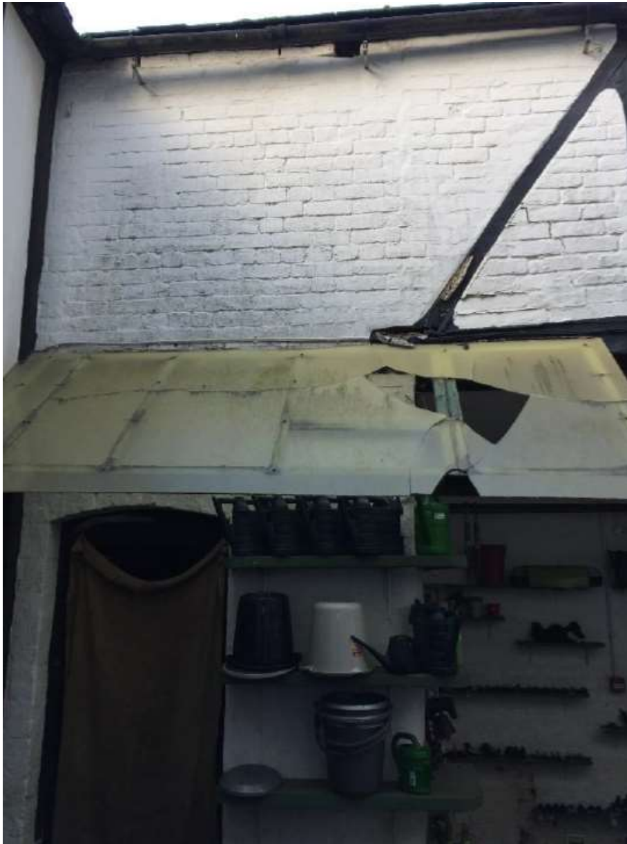
Walls within Courtyard - Photo 8
