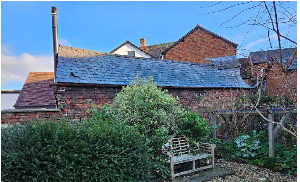
Rear of Courtyard Section – Photo 3
