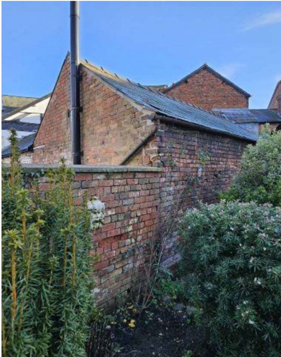
Rear of Courtyard Section – Photo 4
