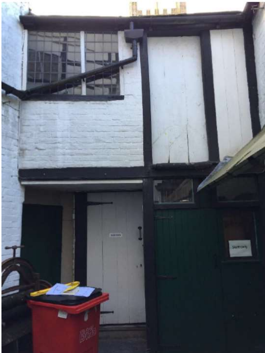
Walls within Courtyard - Photo 7
